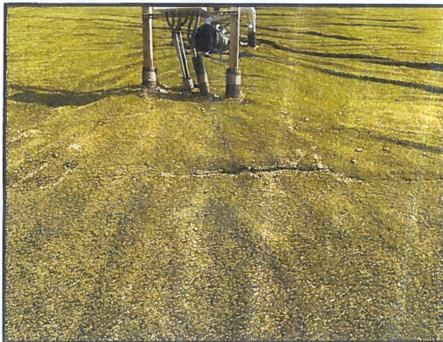
Photograph 7: Tear in ClosureTurf® near LCS-4.
