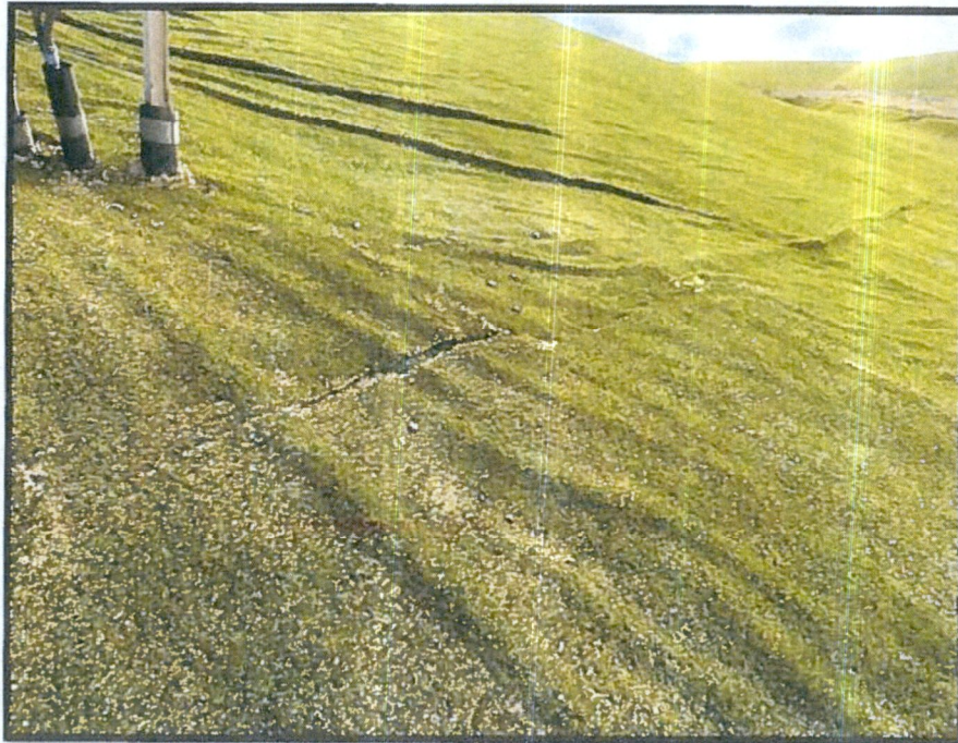
Photograph 9: Additional view of tear in ClosuresTurf®.
