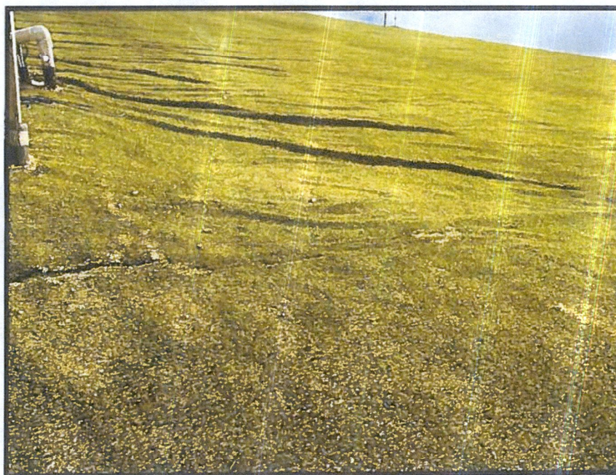
Photograph 8: Additional view of tear in ClosureTurf®.
