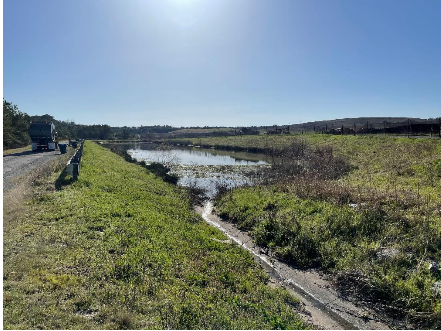
Photo 3: Stormwater Pond North of Compost Facility.
