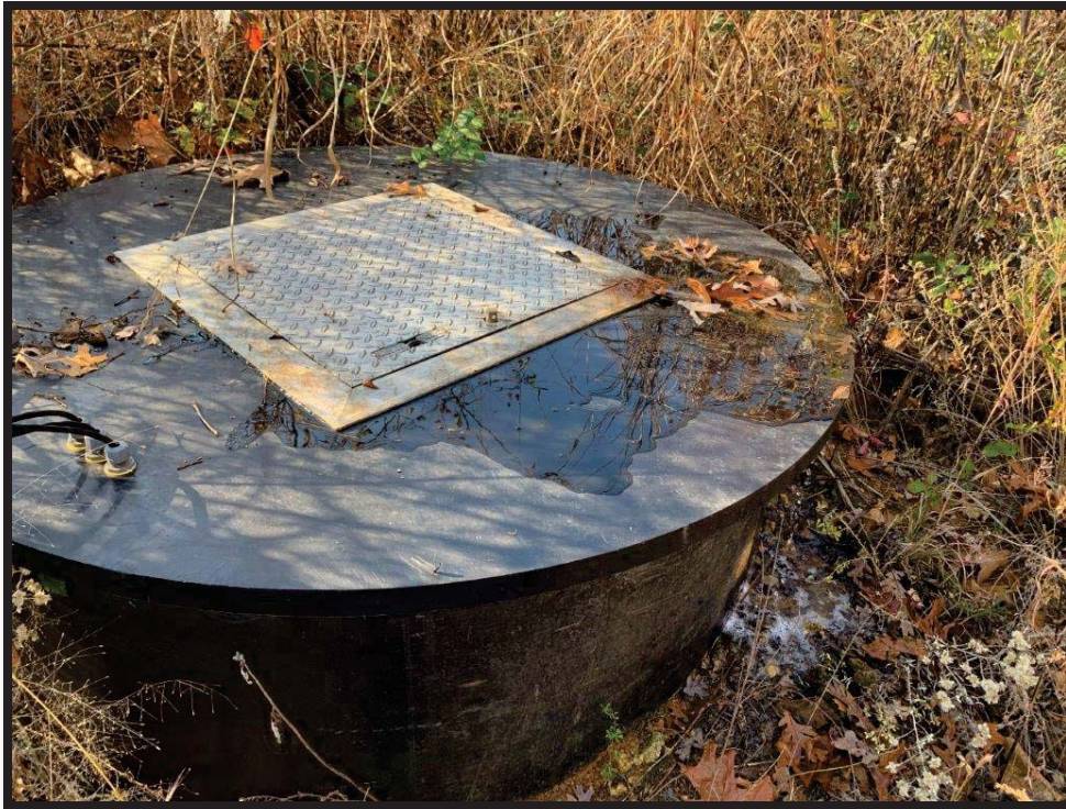
Photograph 1: View of VLCS-2 at capacity.
