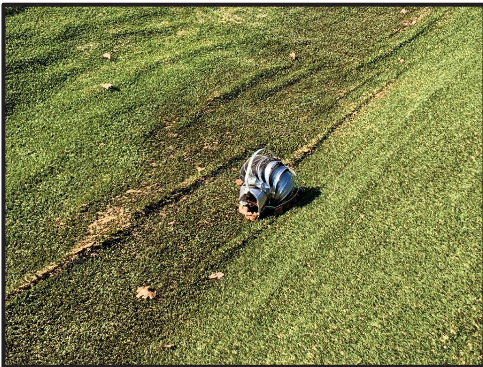
Photograph 6: View of turbine vent near LCS-6 on east side of Area 1-3 cell.
