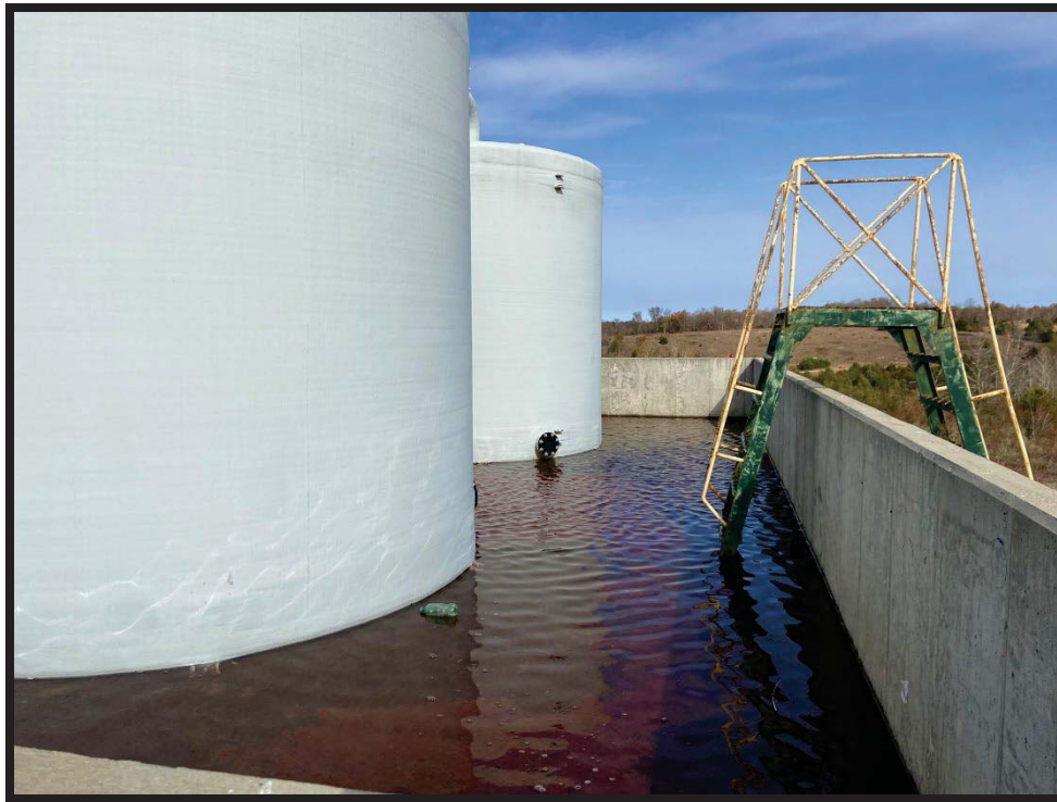
Photograph 1: View north of stormwater in leachate tank containment.
