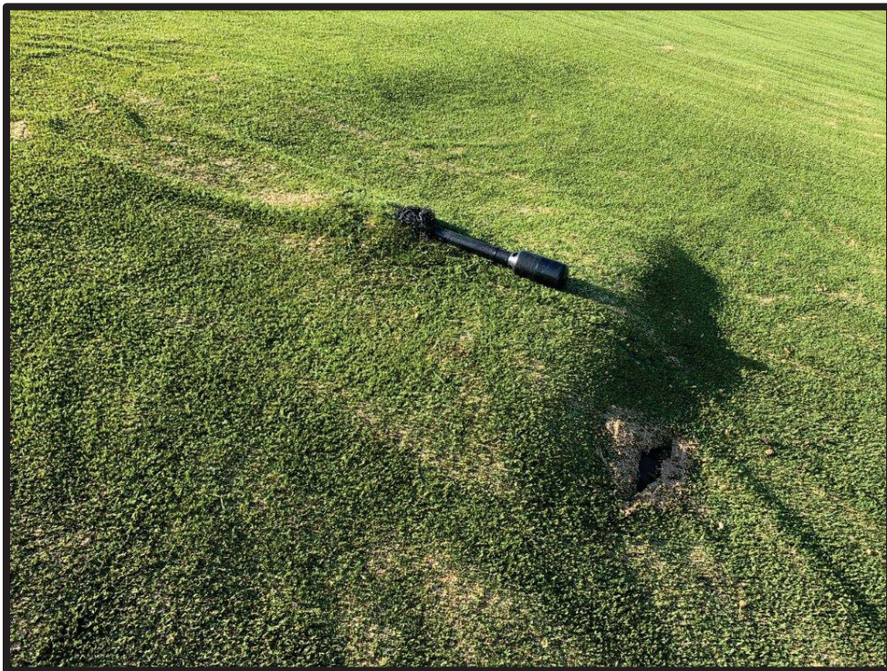
Photograph 4: View southwest of damaged vent pipe near LCS-1.
