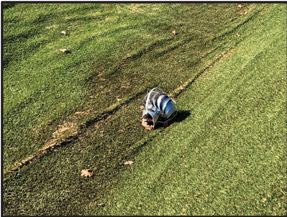
Photograph 6: View of turbine vent near LCS-6 on east side of Area 1-3 cell.
