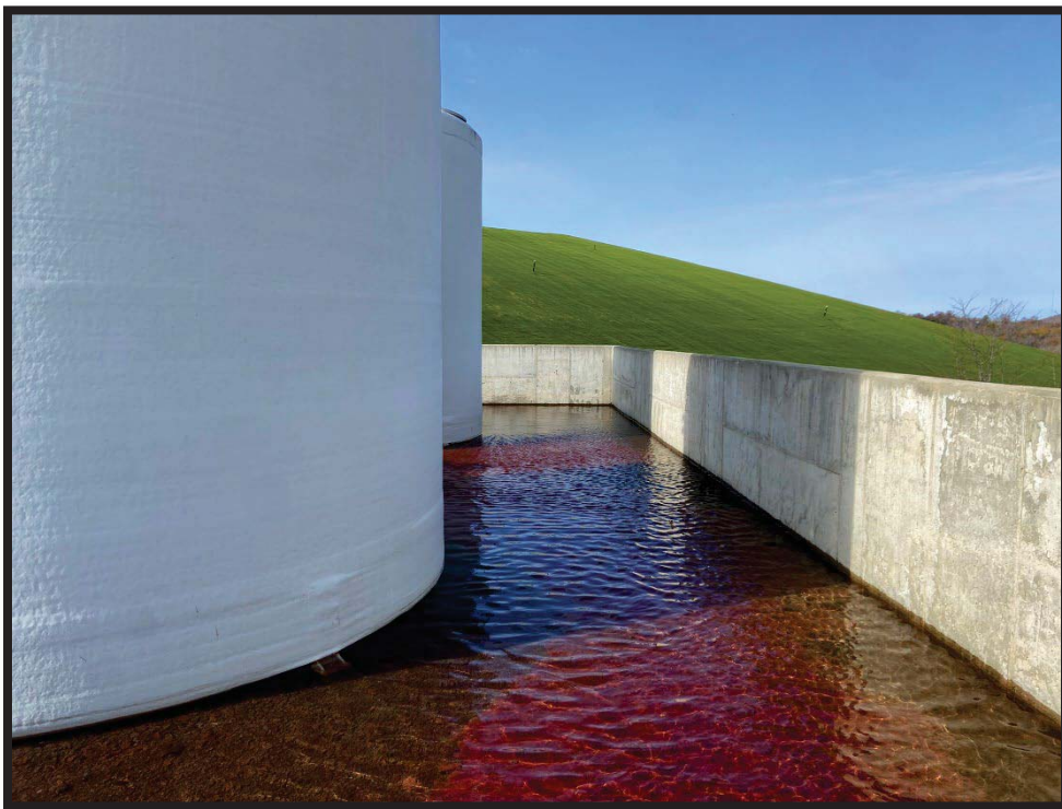
Photograph 2: View west of stormwater in leachate tank containment.
