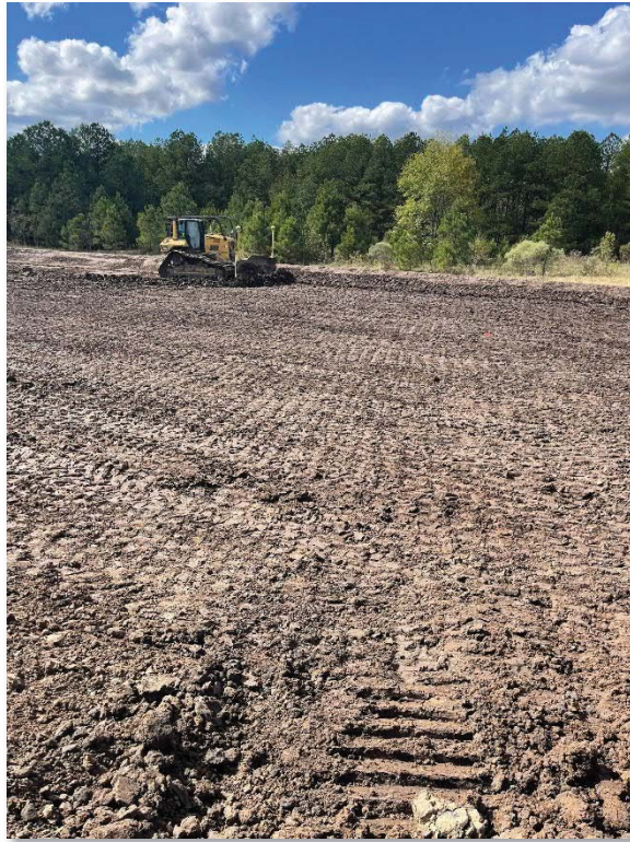
7. Clay Liner Grading with Dozer
