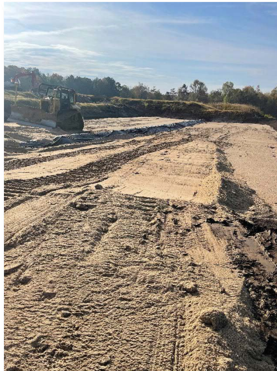
12. Protective Cover Construction
