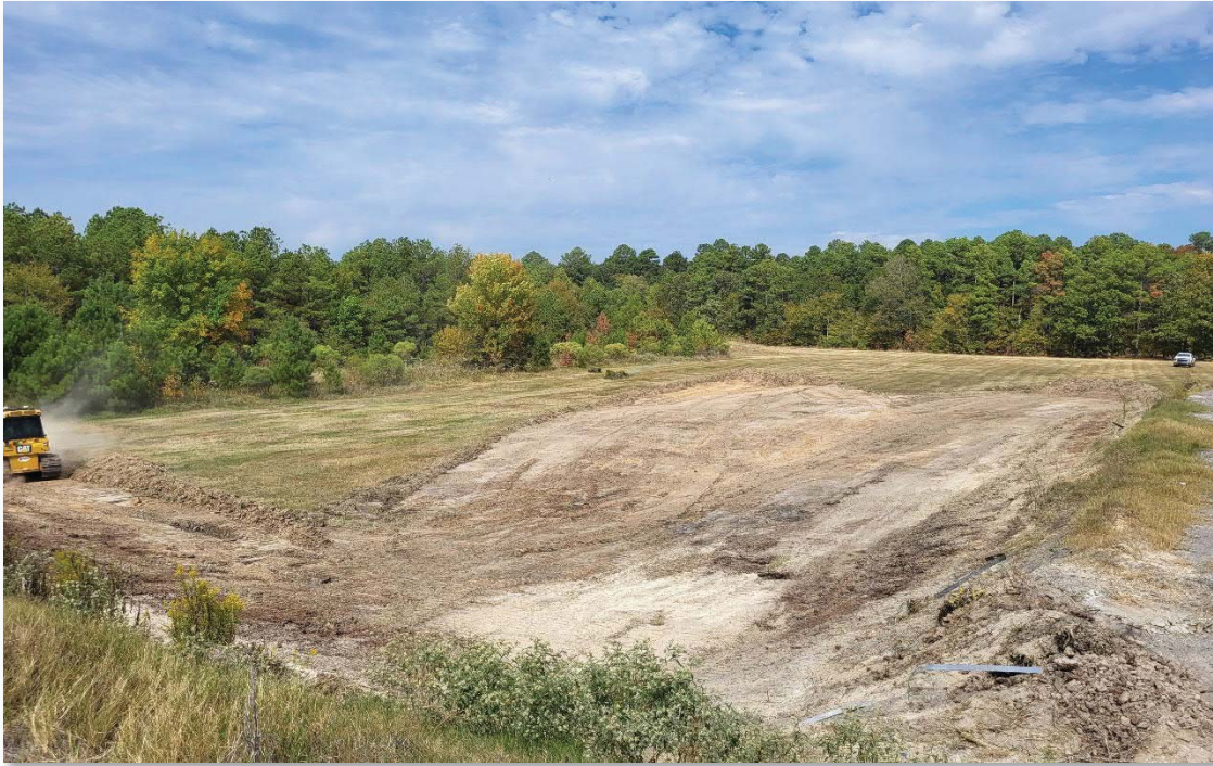
1. Stripping Topsoil
