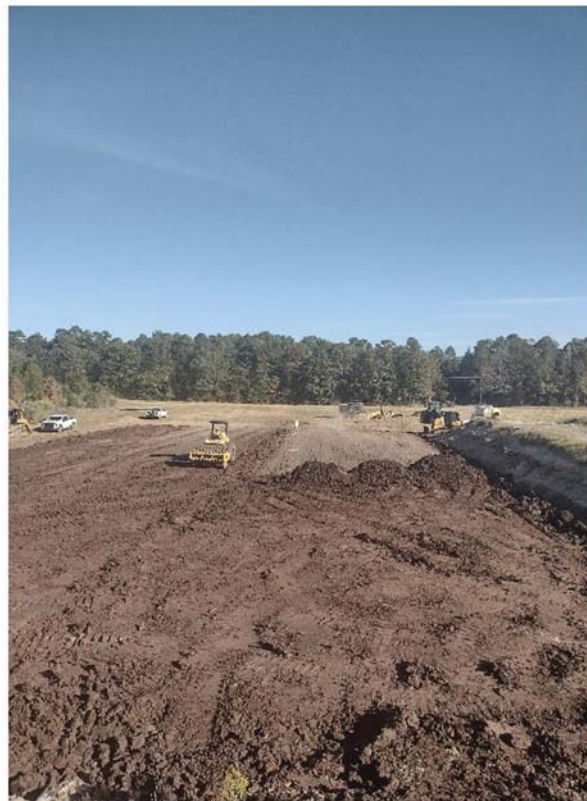
4. Clay Liner Construction
