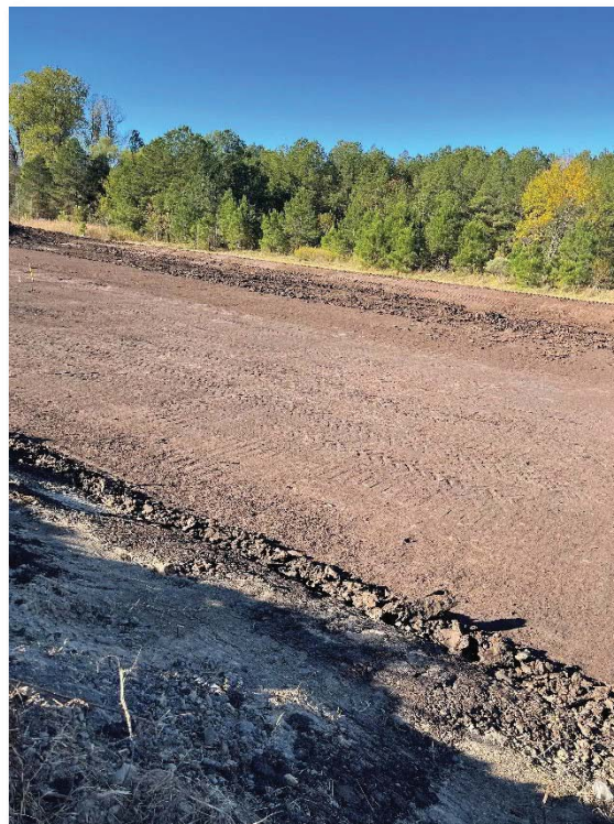
8. Completed Clay Liner
