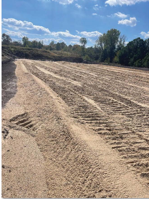
13. Completed Protective Cover
