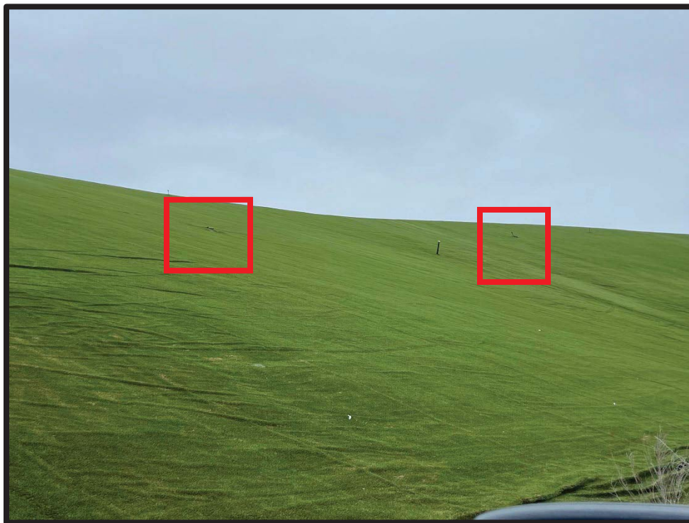
Photograph 4: View of damaged vent pipes near LCS-1.
