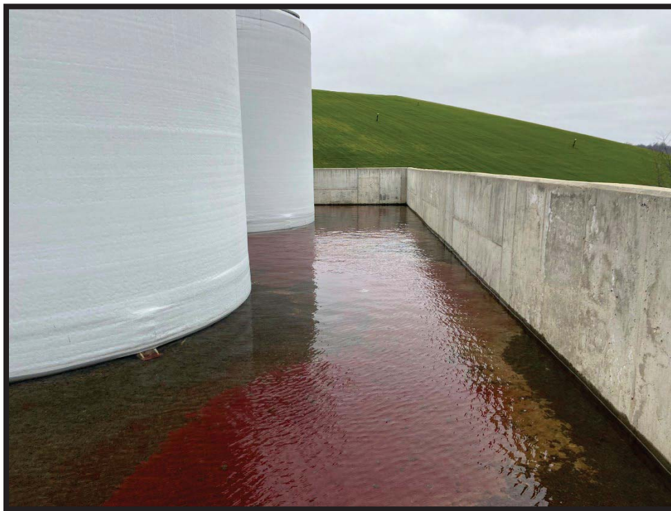
Photograph 2: View west of leachate tank containment.
