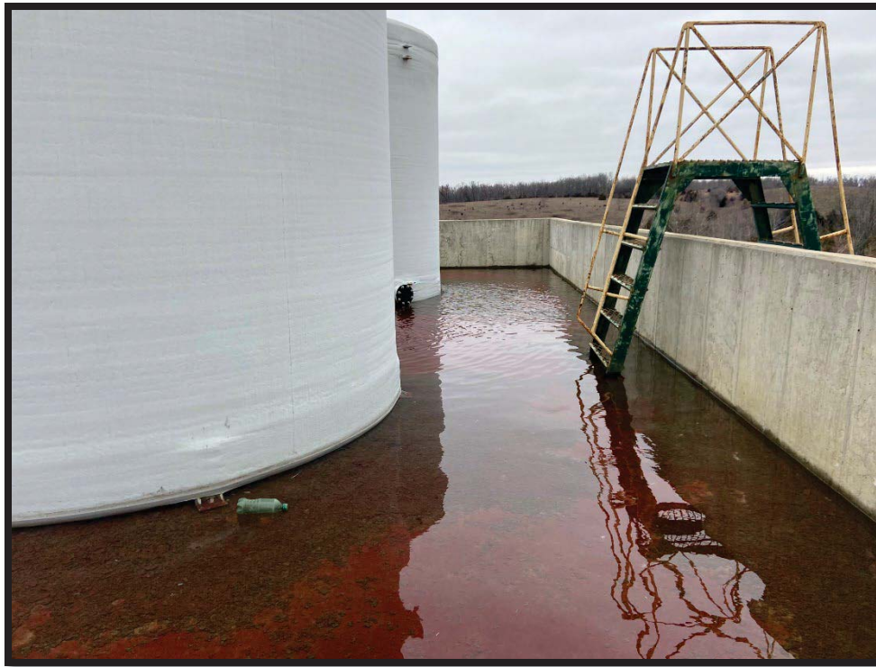
Photograph 1: View north of leachate tank containment.
