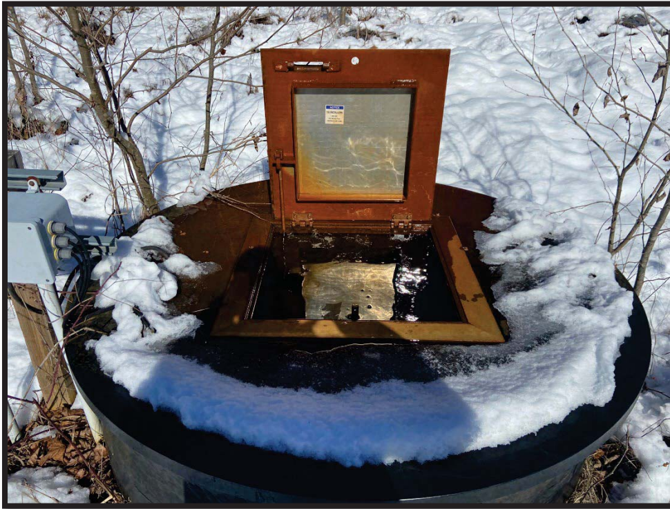
Photograph 3: View of VLCS-1 at capacity.
