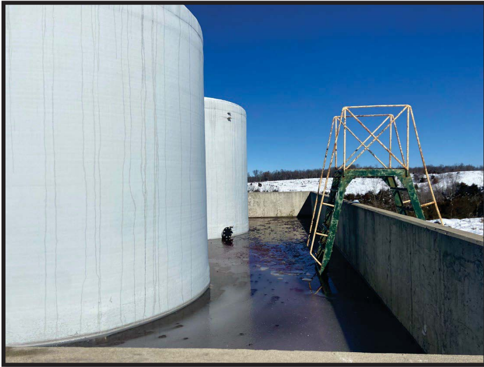
Photograph 1: View north of leachate tank containment.
