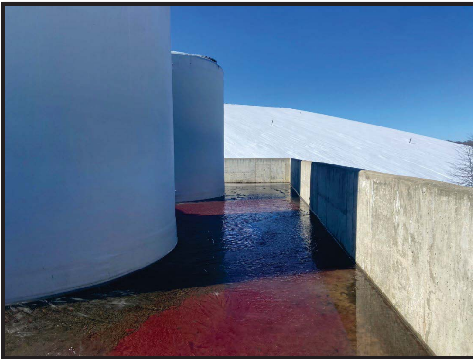
Photograph 2: View west of leachate tank containment.
