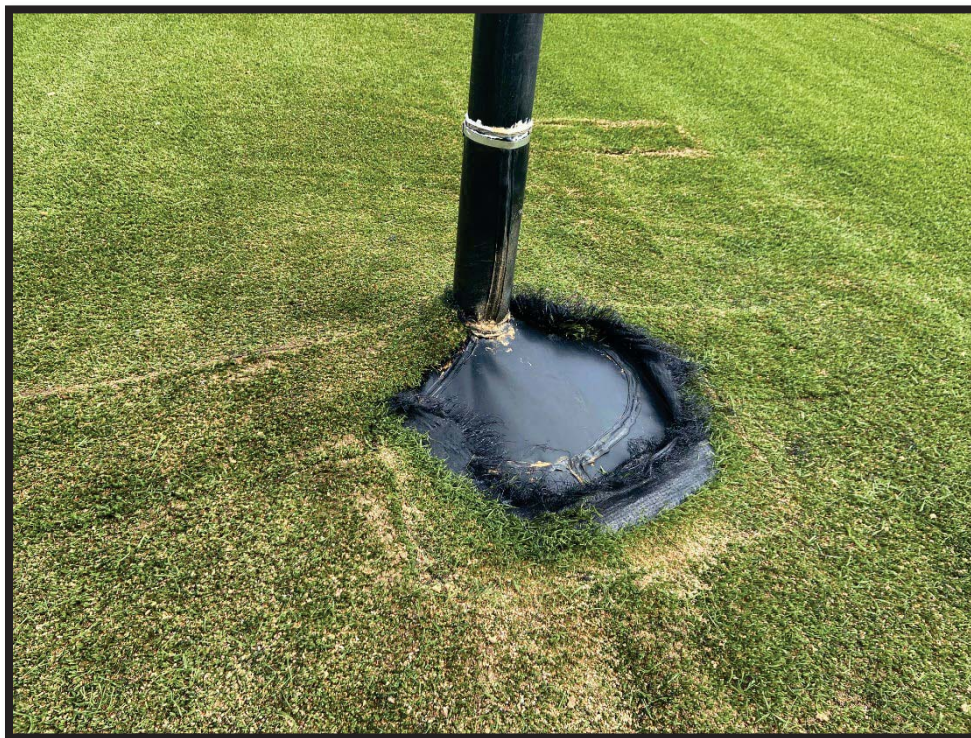
Photograph 2: View of damaged closure turf near LCS-4.
