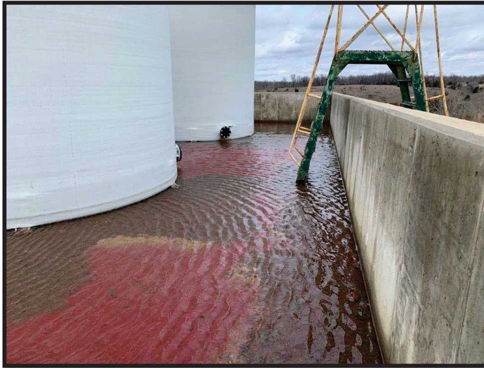
Photograph 1: View of stormwater in leachate tank containment.
