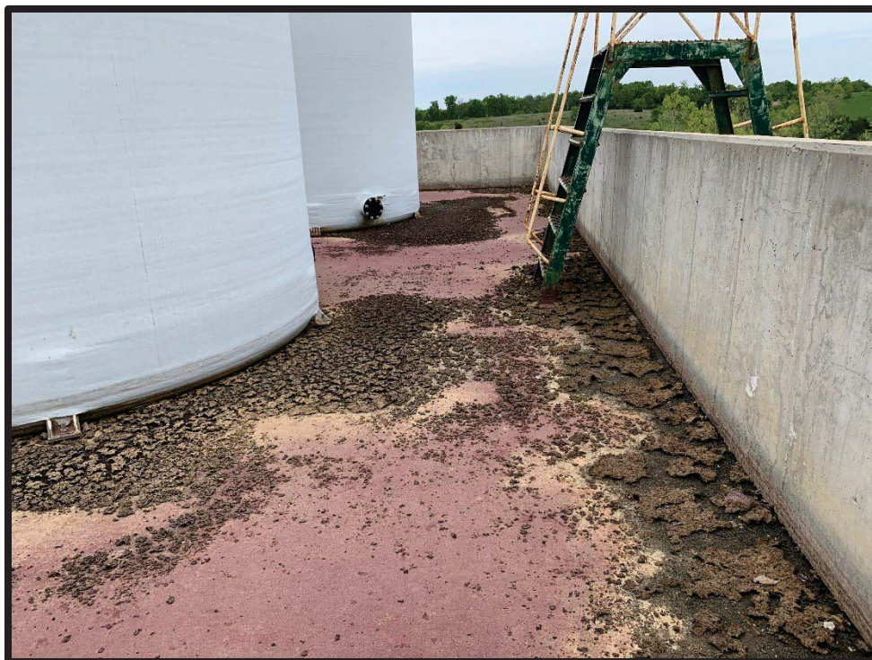
Photograph 2: View of dry conditions in leachate tank secondary containment.
