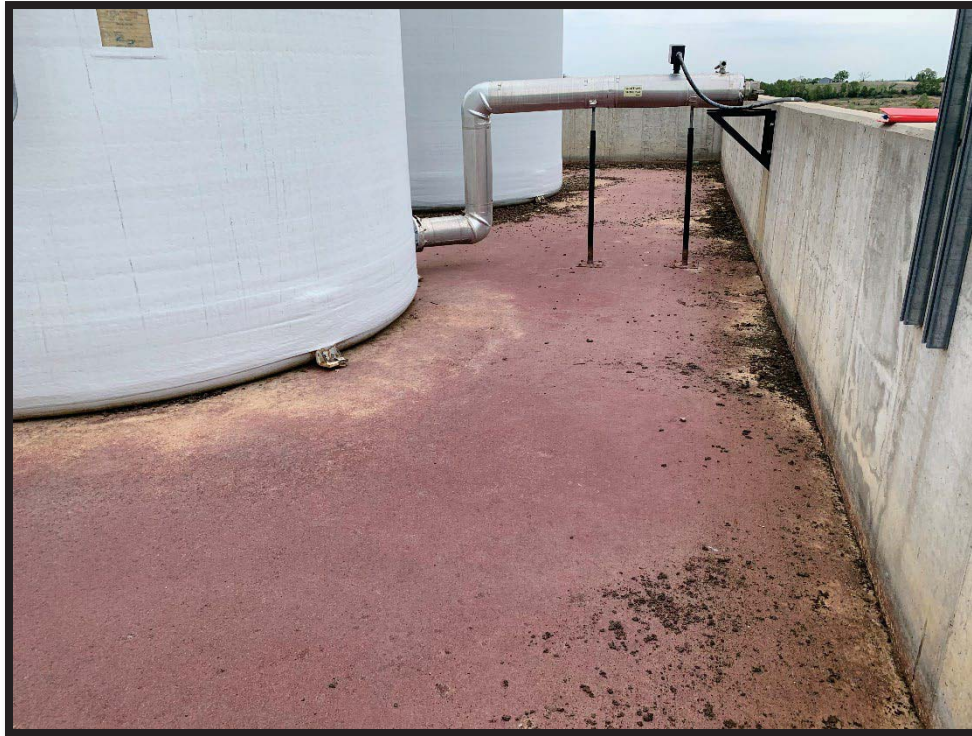
Photograph 1: View of dry conditions in leachate tank secondary containment.
