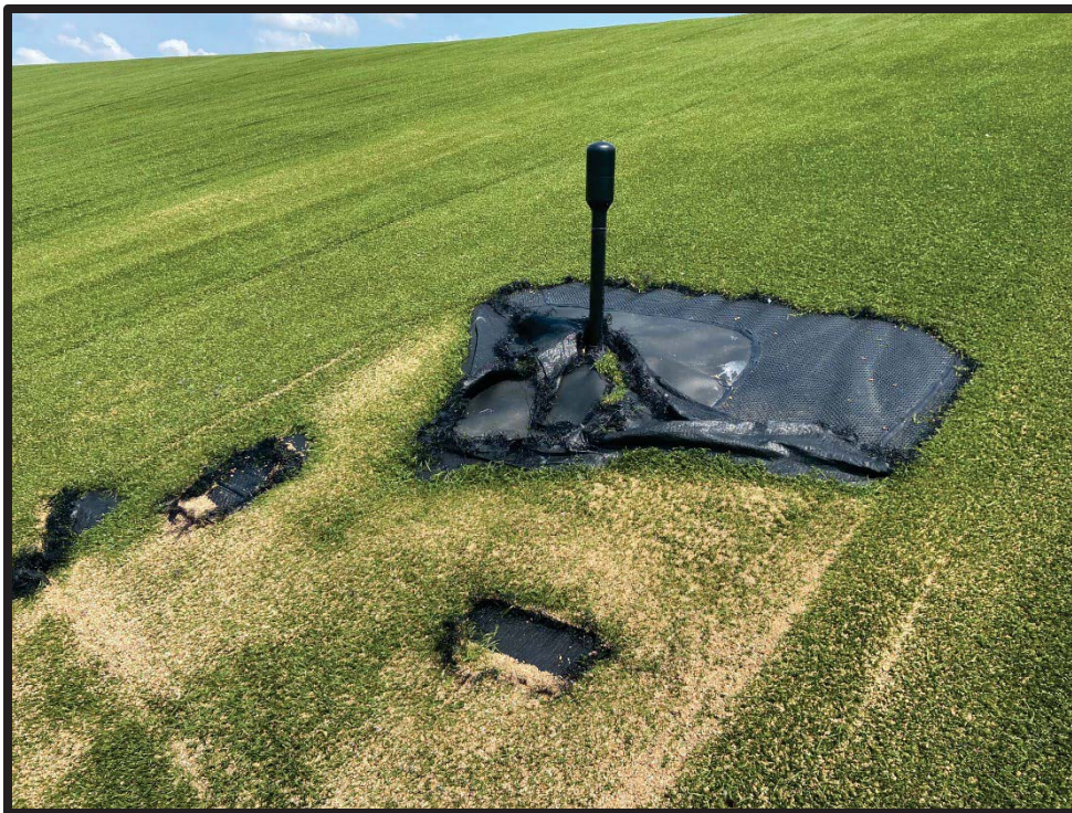
Photograph 4: Closure turf tear around PRV on the south side of Area 1-2, near LCS-4.
