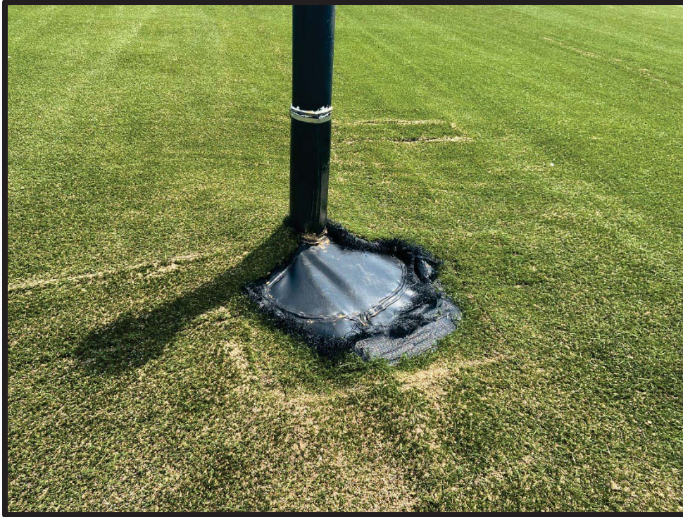
Photograph 3: Closure turf tear around turbine vent on the south side of Area 1-2, near LCS-4.
