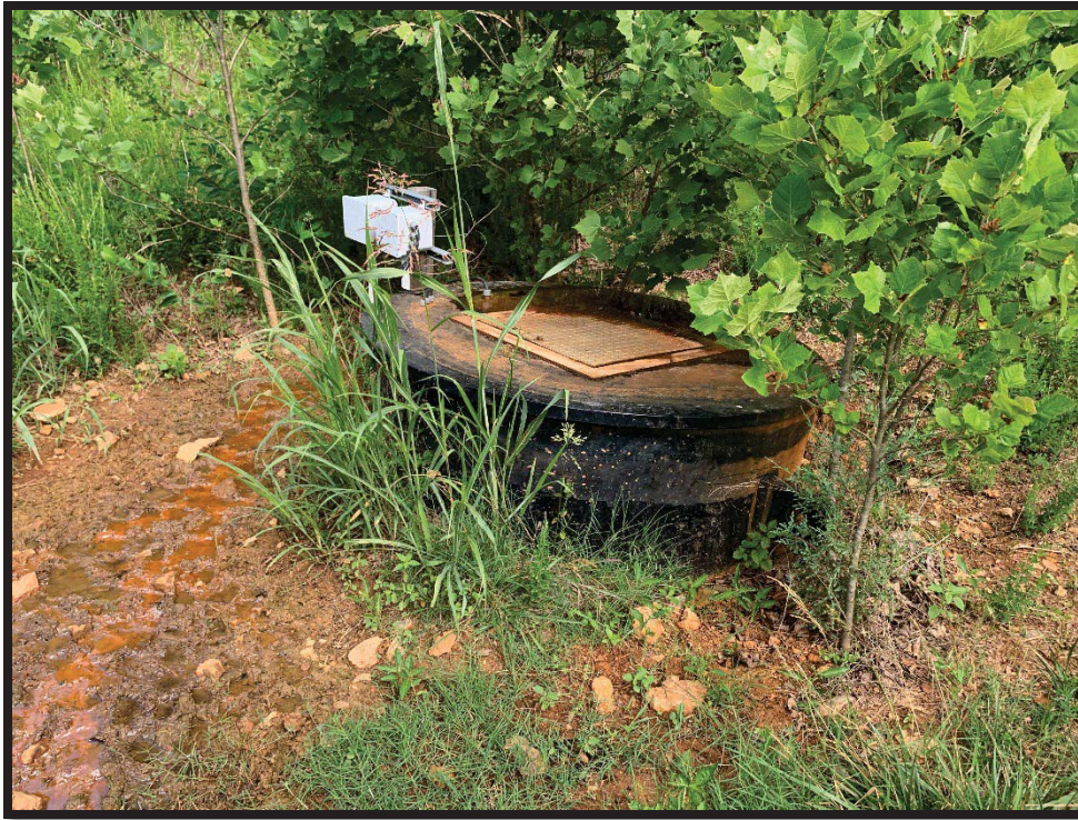
Photograph 5: View of stressed vegetation from VLCS-1 overflow. Abundant deer tracks visible in mud.
