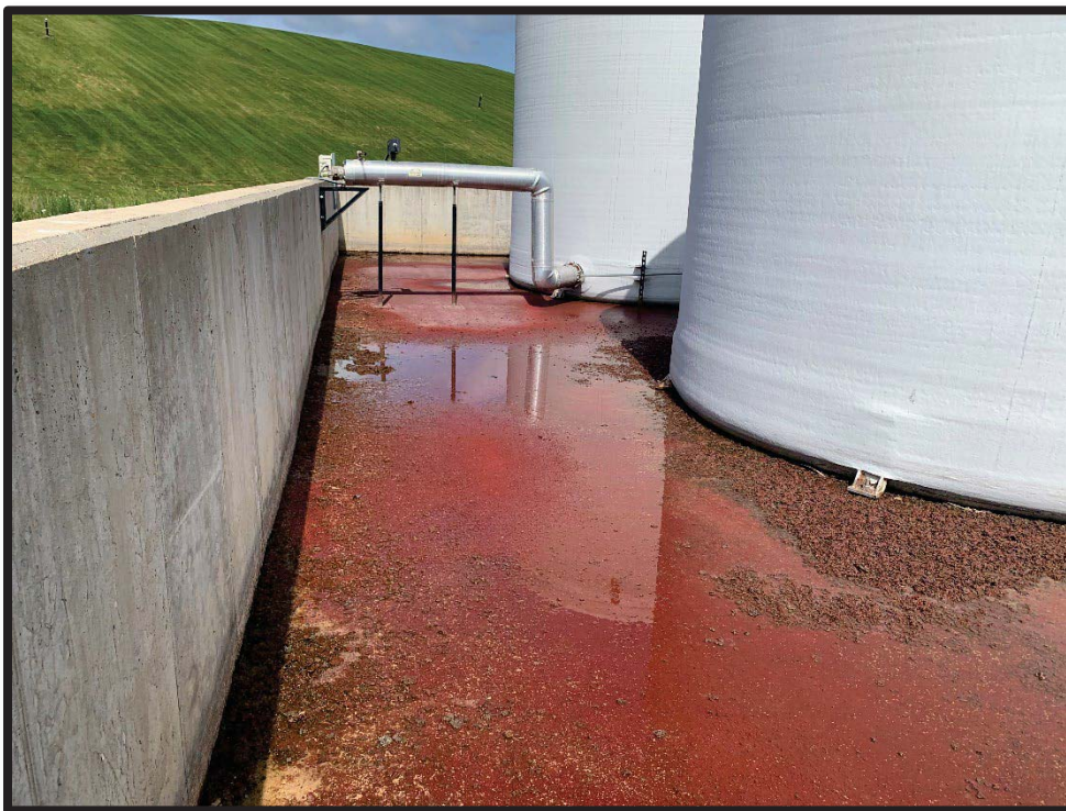
Photograph 2: View north of leachate tank secondary containment.
