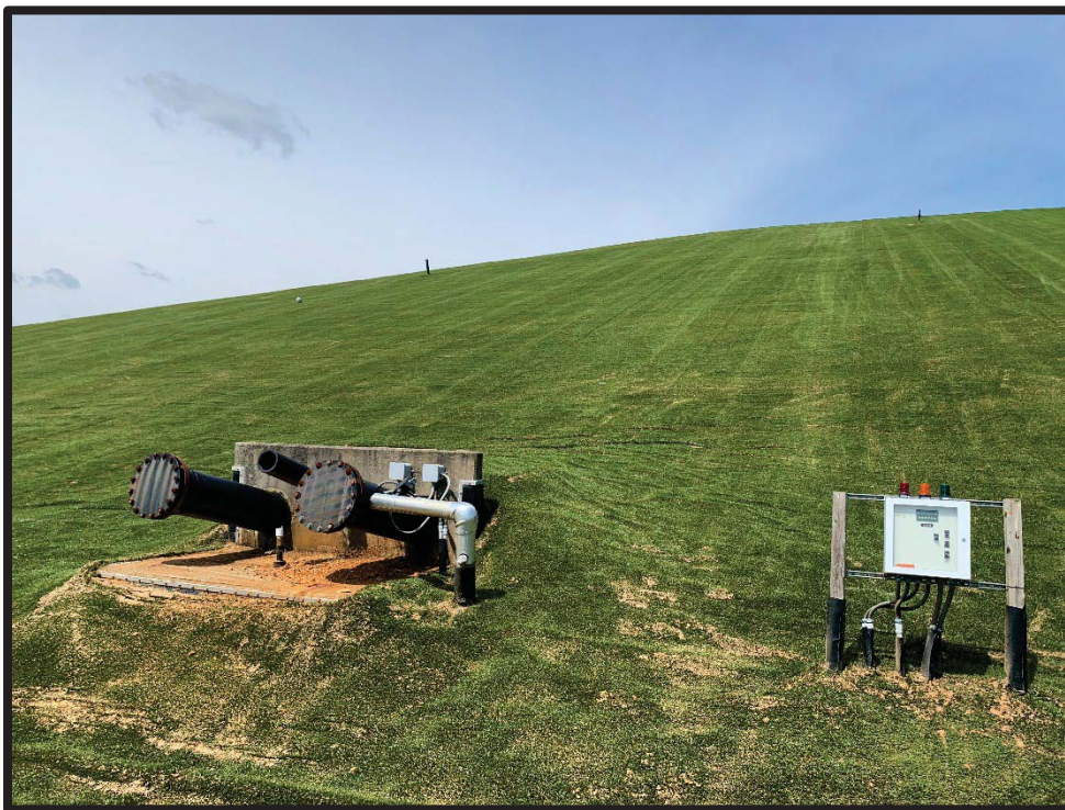
Photograph 8: View southwest of LCS-8. Detached whirligig vent visible in distance.
