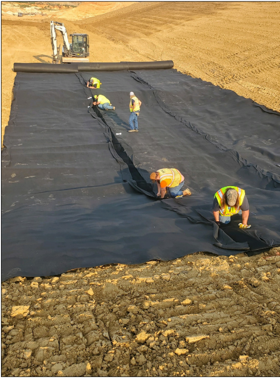
Photo No. 7 Contractor installing Geocomposite in the leachate sump.
