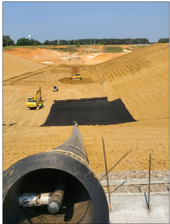
Photo No. 8 Looking west and installed 18" side slope riser.
