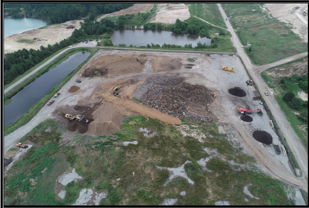
3. East side of compost facility looking West
