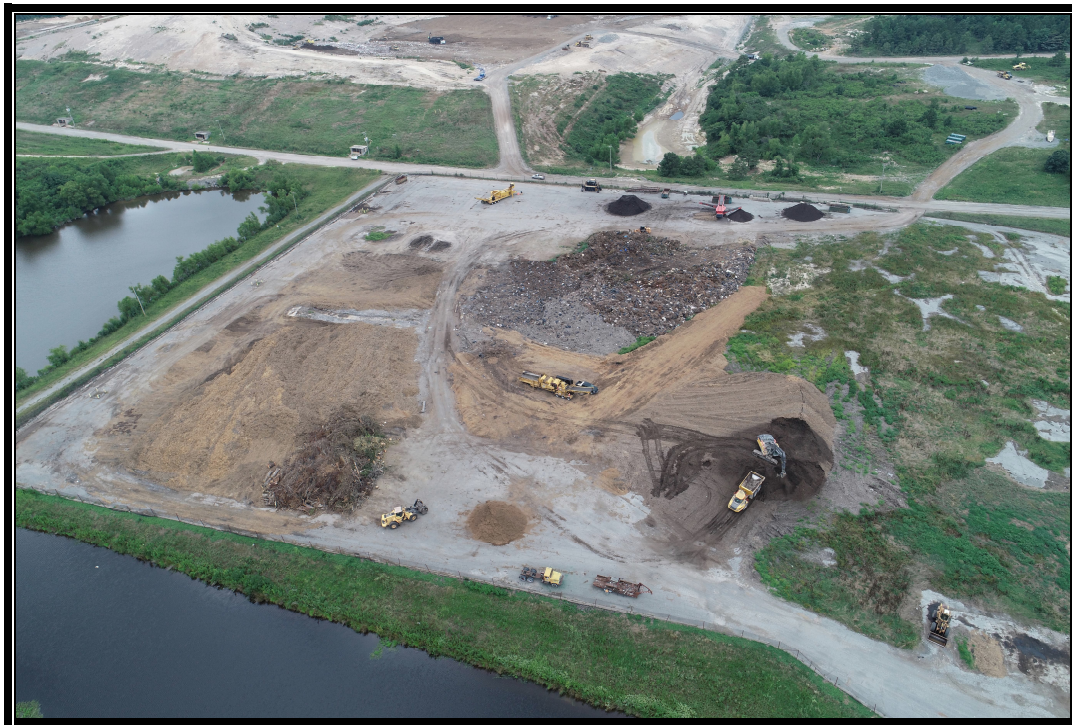
4. North side of compost facility looking South
