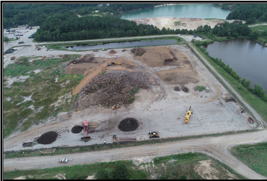
2. South side of compost facility looking North
