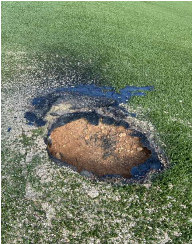
9. Turf and Liner damage (before and during repair)
