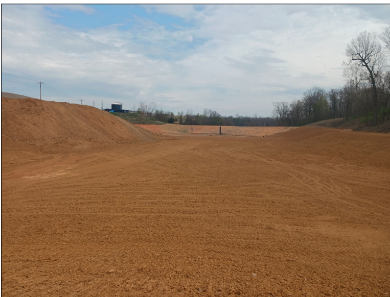
Photo No. 10 Looking east at the West Basin (under construction).
