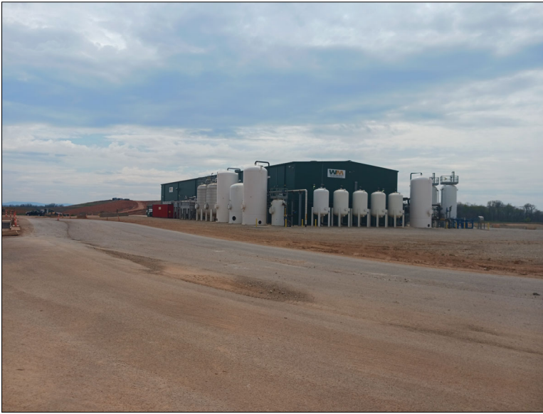
Photo No. 8 Looking southwest at the RNG Facility.
