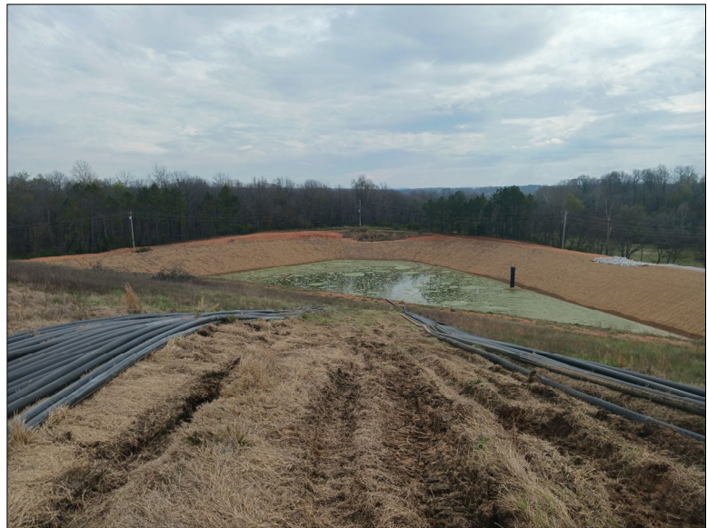
Photo No. 12 Looking south at the South Basin.
