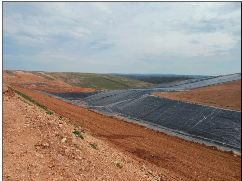
Photo No. 5 Looking southeast at Cell 13A (under construction).
