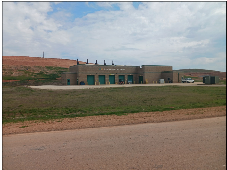
Photo No. 6 Looking east at the Landfill Gas to Energy Plant.
