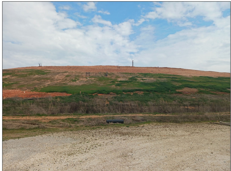
Photo No. 2 Looking east at the west slope of the active Class 1 Landfill.
