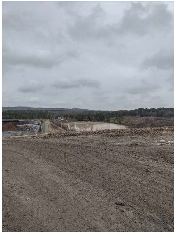
Looking North over Compost Pad (left), Detention Pond (center), Class 4 (right)
