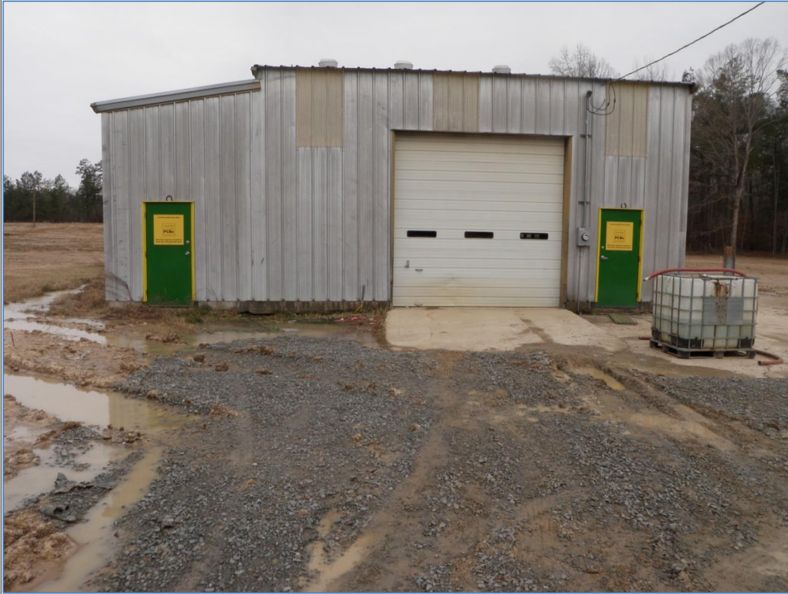
Warning Signs Placed on the Warehouse Building
