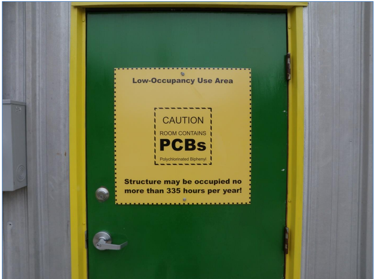
Warning Sign Placed on Entrance to Warehouse Building
