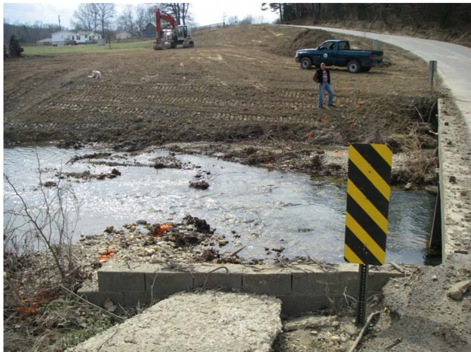
Two more photos of the downstream side of the current bridge, with the unstabilized areas right down to the water line. There were no erosion controls at this site.
