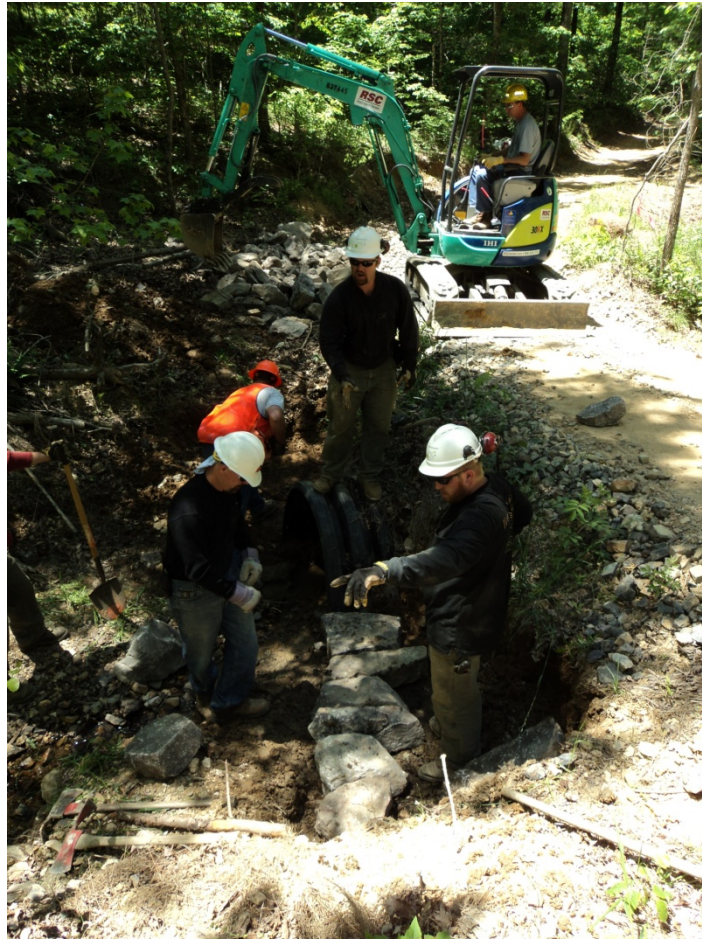
Figure 2. Ouachita ATV Club, Trails Unlimited, and Ouachita NF employees installing an arch culvert to reduce sediment and improve water quality.
