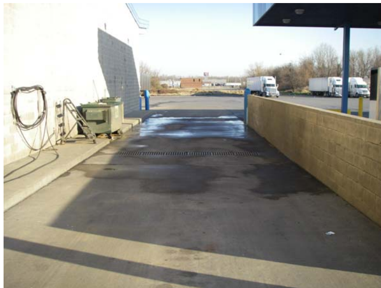
This photo shows the outdoor washing station. The grated drain seen in this photo is allowing rain water to enter the pretreatment system, thereby diluting the process wastestream.
