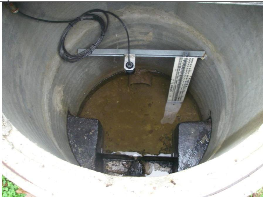
**Photographer:** John Fazio      **Witness:** Gerald Cantrell**Photo #** 4    **Of** 4    **Date:** 11/21/11    **Time:** 1113**Description:** Improvements made to one of the two sand filter beds to allow for a more uniform wastewater distribution over the bed.
