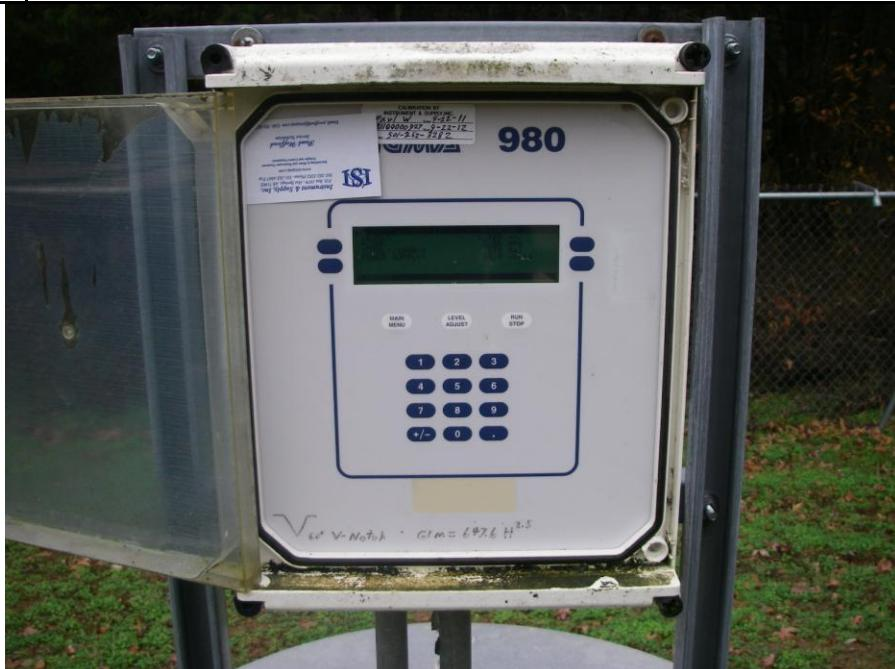
**Photographer:** John Fazio      **Witness:** Gerald Cantrell**Photo #** 2    **Of** 4    **Date:** 11/21/11    **Time:** 1112**Description:** Effluent meter and effluent weir sump.
