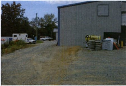
Used oil container system eliminated & removed. Spilled oil contaminated dirt removed disposed of properly and new material added to ground. Water Department Building.
