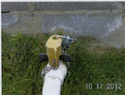
Lock placed on refueling detention basin drain valve. Water/Waste Water.
