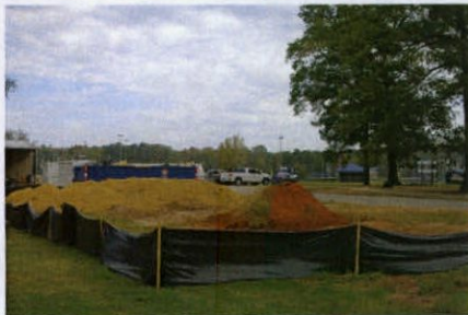
Parks field treatment materials encased on three sides to stop silt from leaving site. This is temporary fix till permanent bays are constructed.
