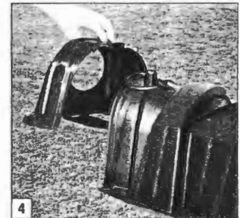
Place end cap onto first chamber.
