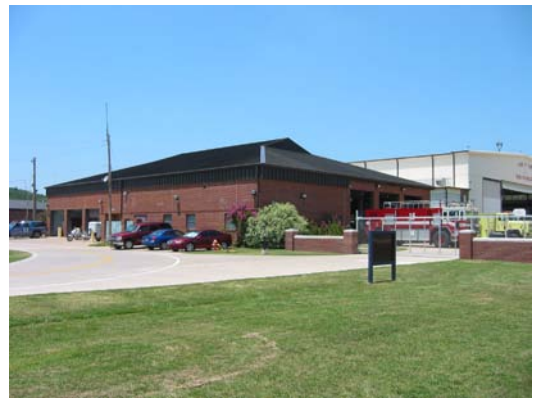
Building 201, the existing Fire/Crash Rescue Station, would be demolished upon construction of a new facility.
