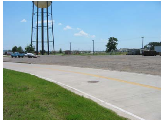
This gravel area would be paved as part of the water tower parking area project.
