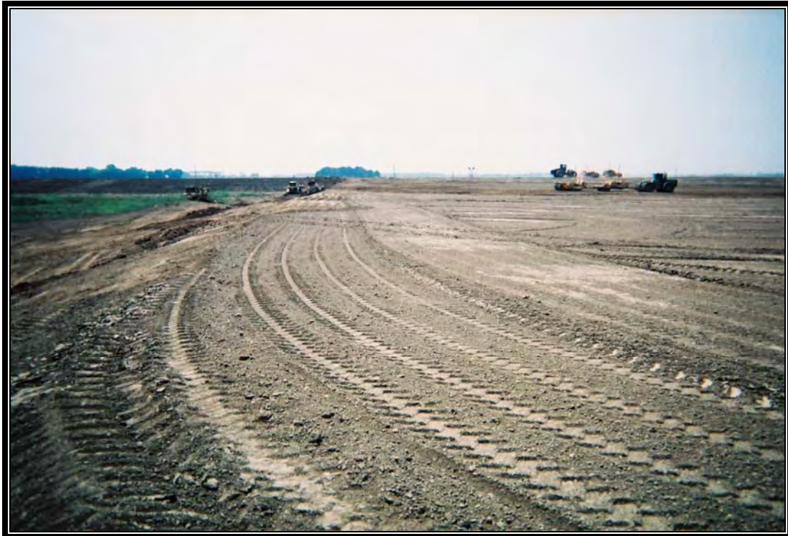
Installation of subgrade on south end of Cell 1
