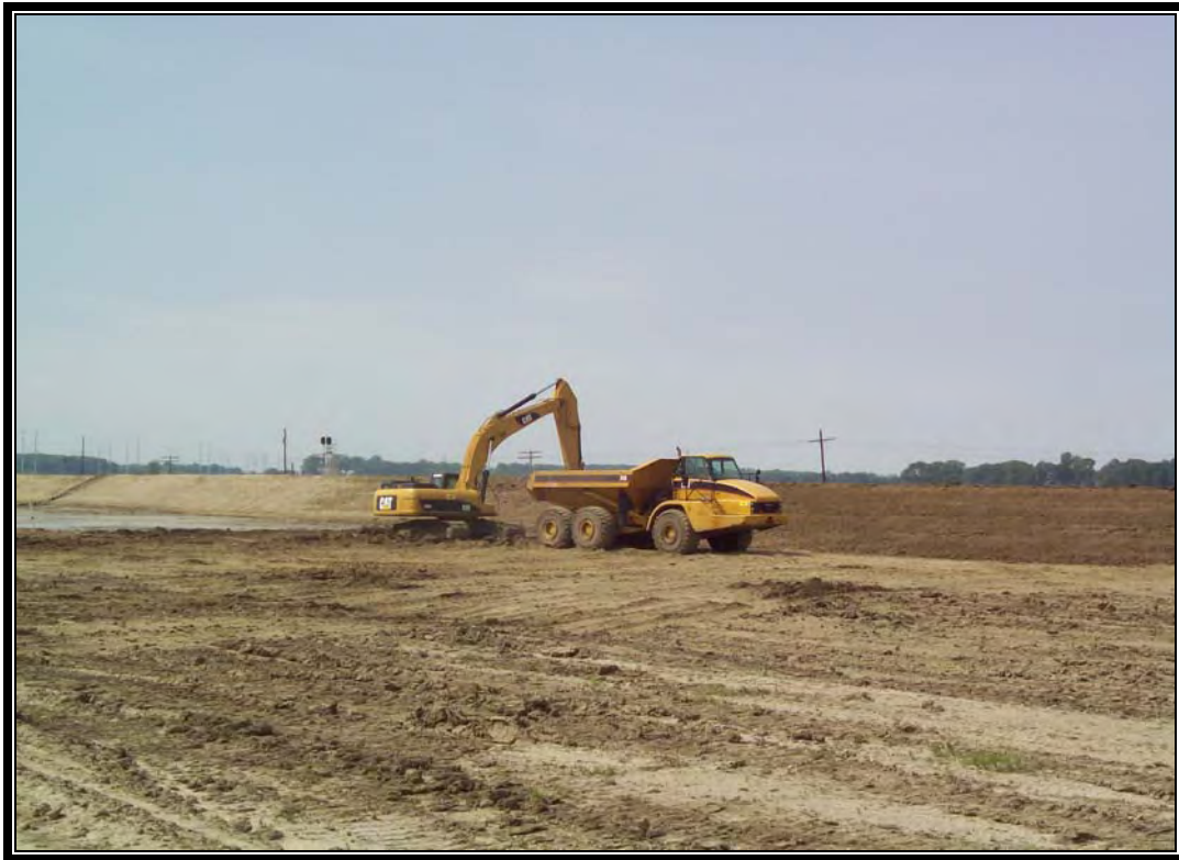
Looking west at excavation of Cell 1
