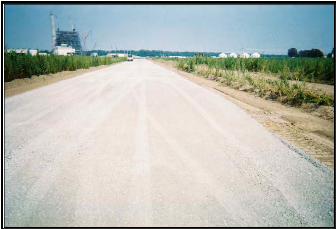
Looking west at construction of north perimeter road
