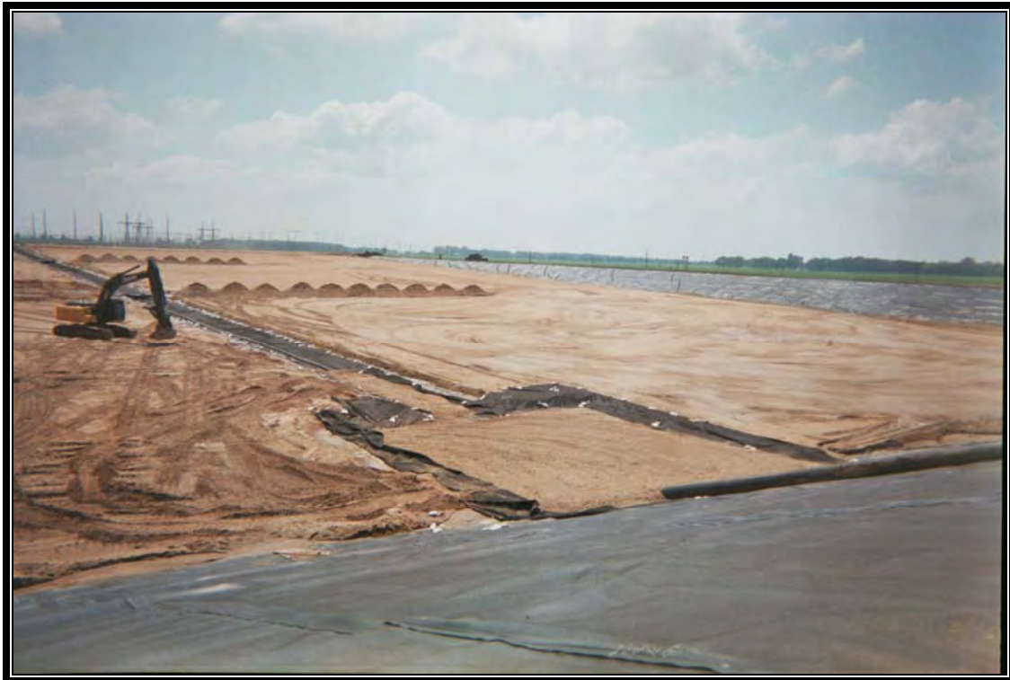
Looking south east at installation of protective cover layer
