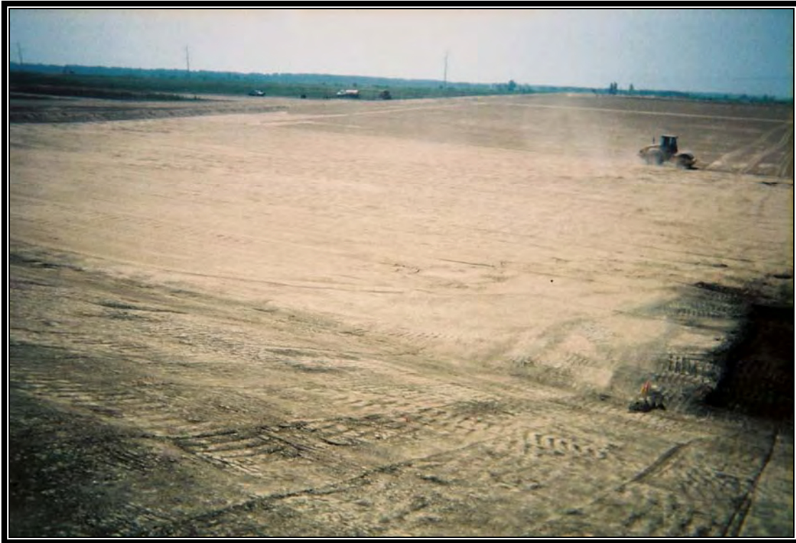
Looking south at completed clay liner
