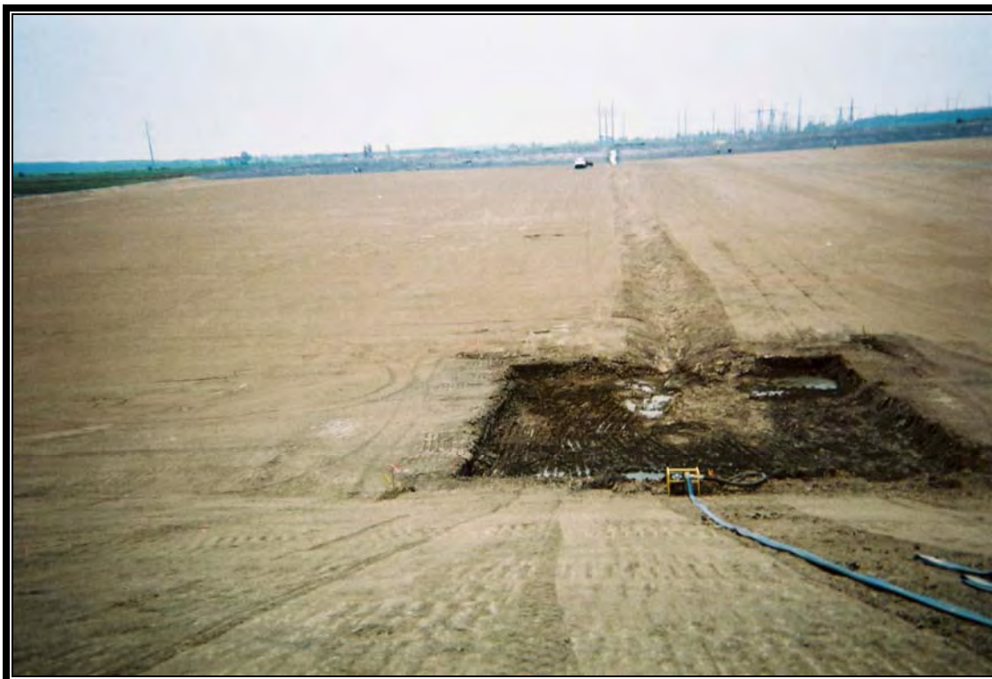
Installation of sump at north end of Cell 1
