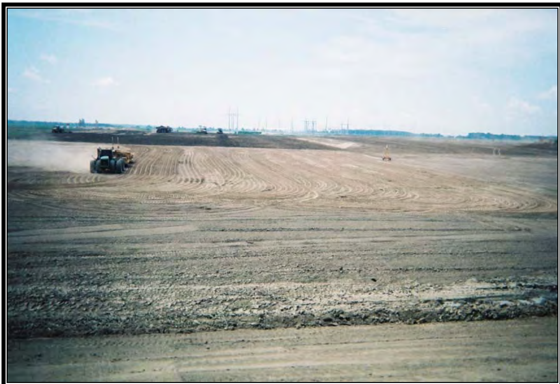
Looking south at installation of compacted clay liner
