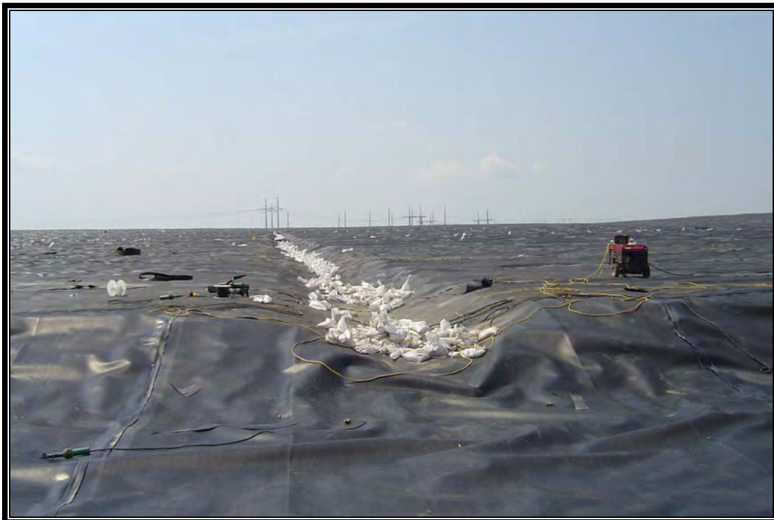
Looking south at completed 60-mil geomembrane liner installation in Cell 1
