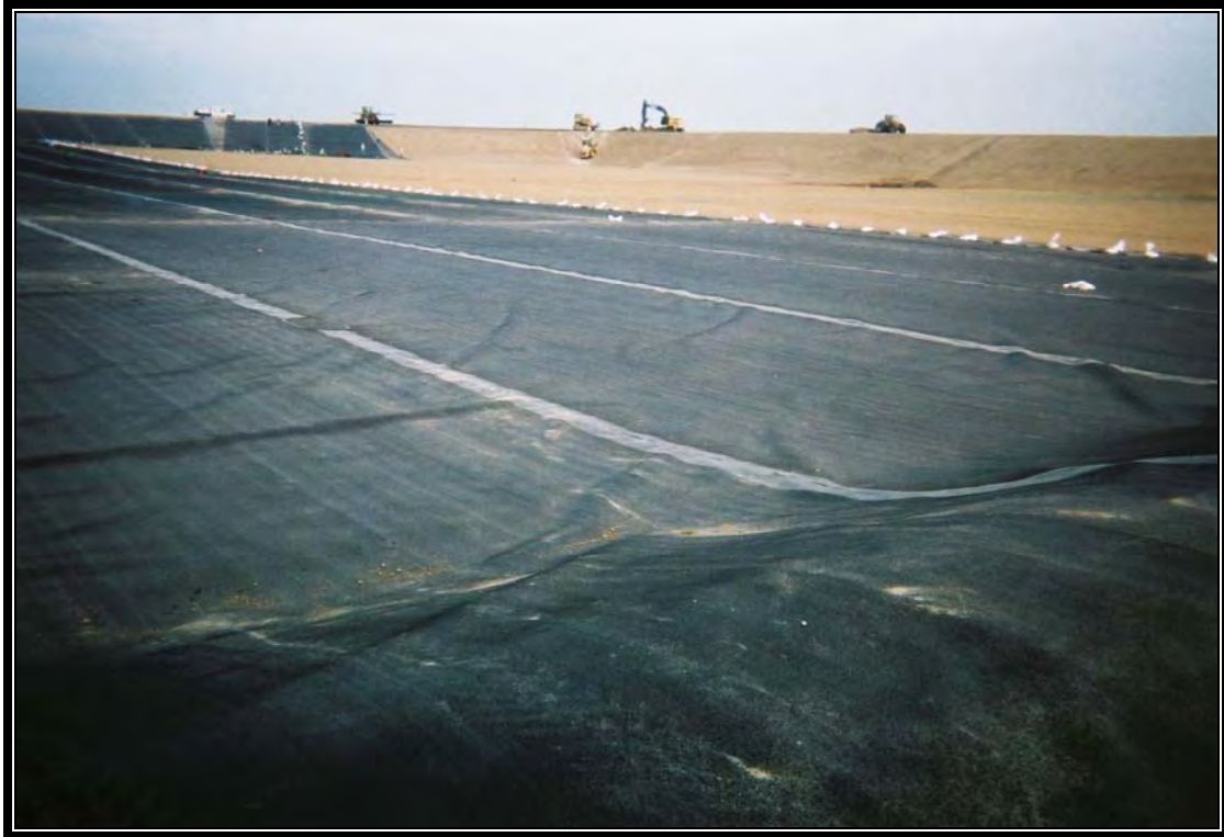
Looking northwest at 60-mil geomembrane liner installation in Cell 1
