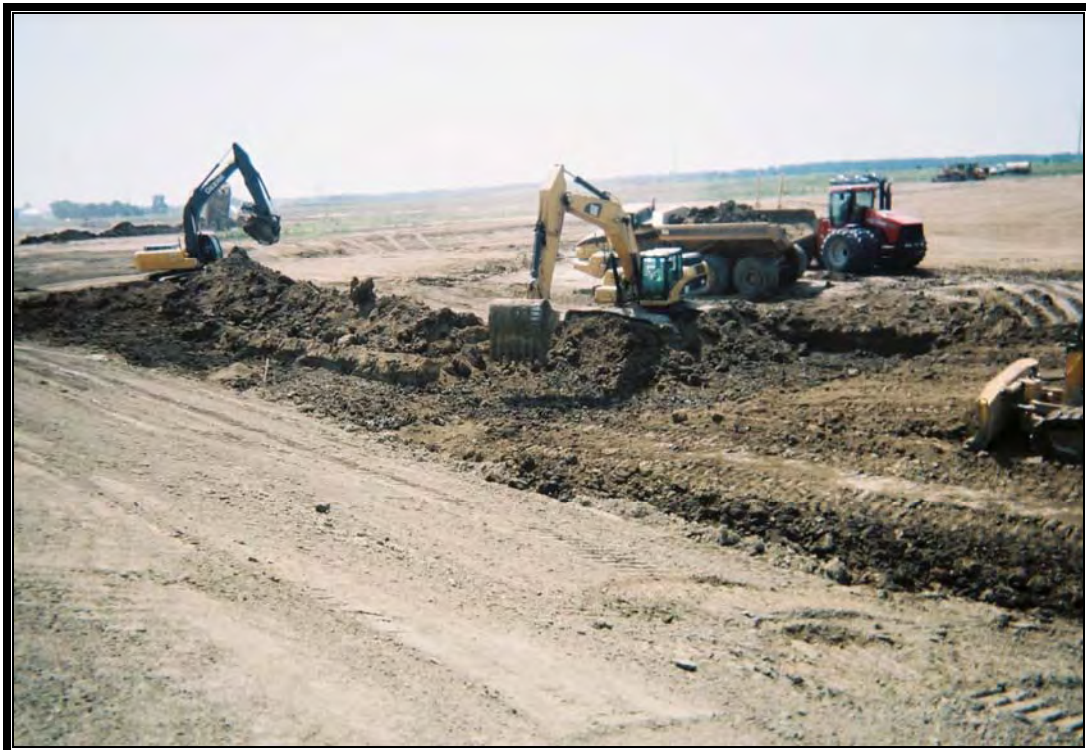
Looking southwest at excavation of north end of Cell 1
