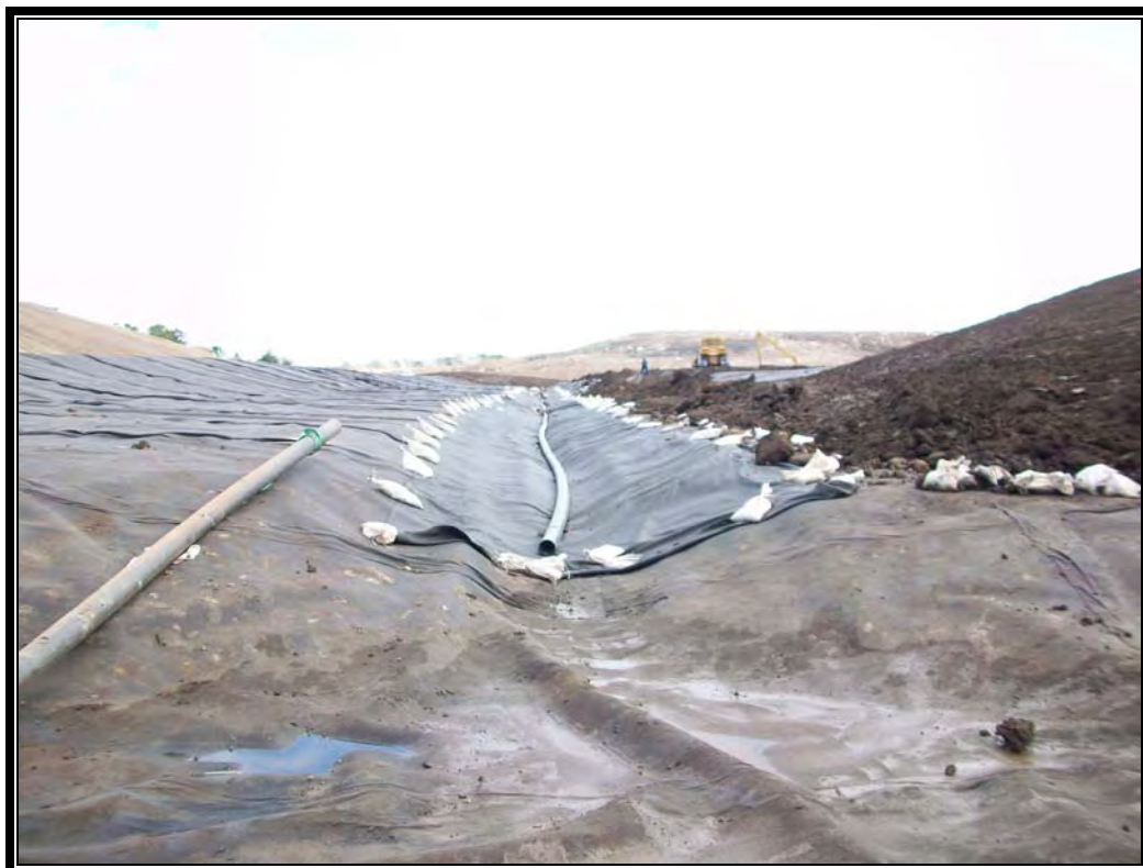
Installation of leachate collection trench in Cell 4
