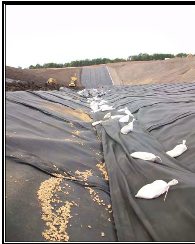
Completed leachate collection system in Cell 4
