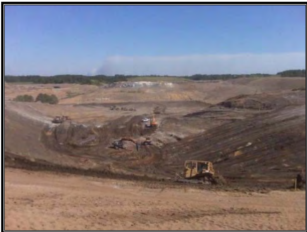
Looking east at excavation of Cell 4
