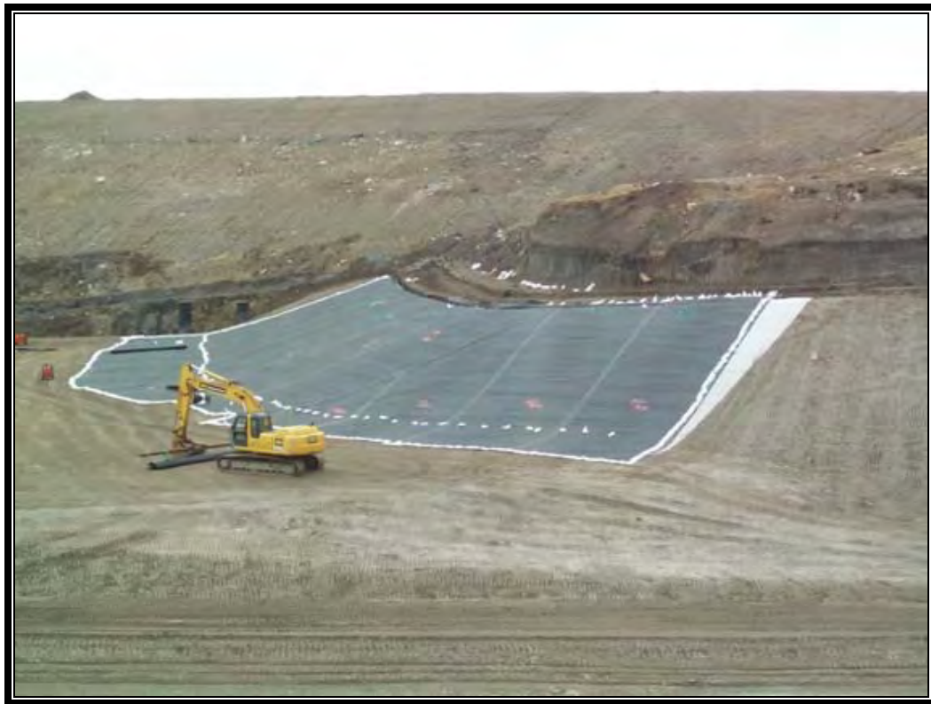
Looking south at installation of GCL and 60mil geomembrane in Cell 4
