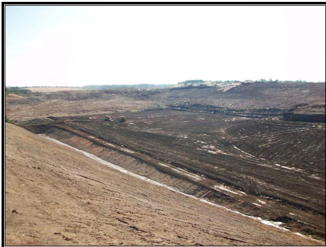
Looking southwest at completed Cell 4
