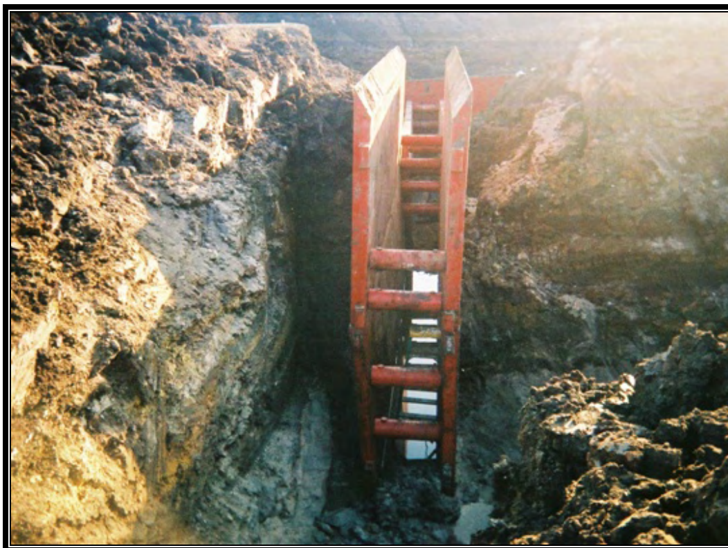
Installation of under-drain system in Cell 4
