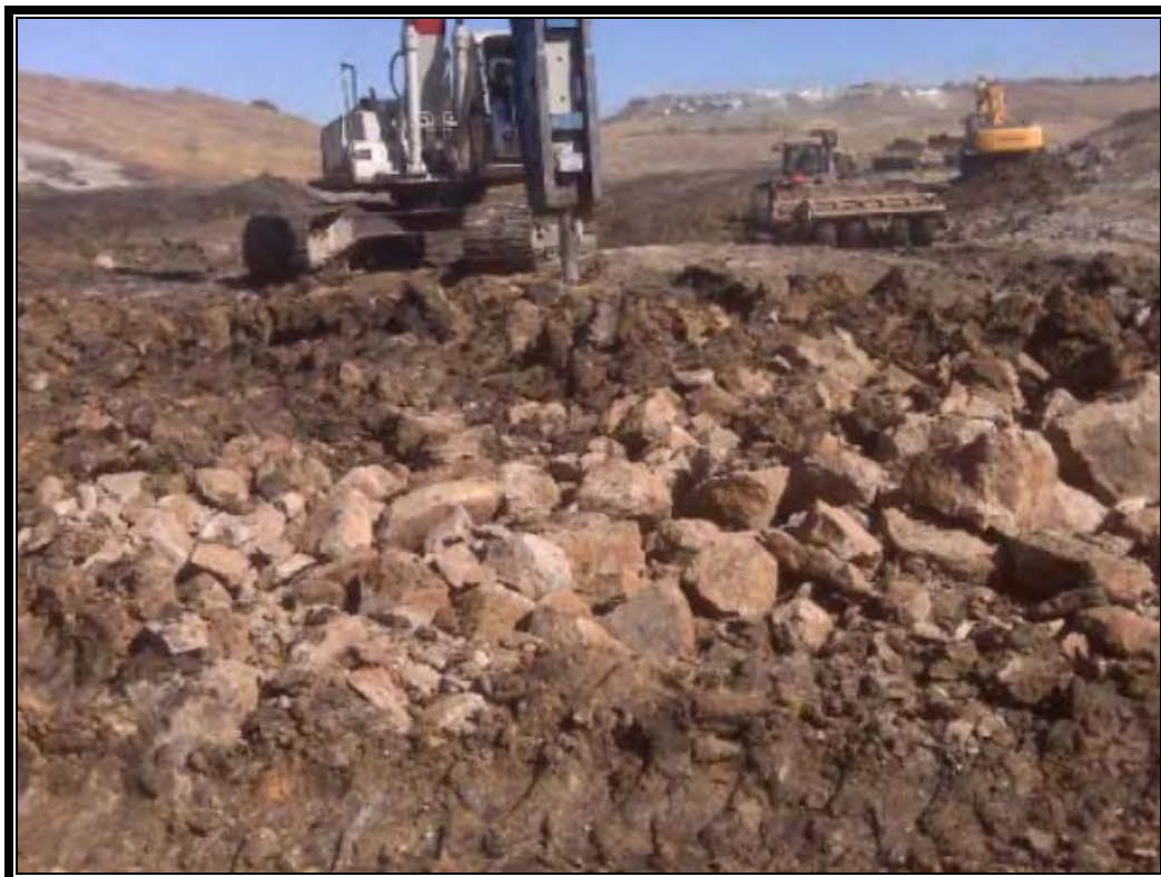
Excavation of rock near sump of Cell 4
