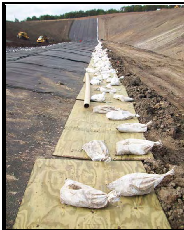
Looking west at north liner overbuild
