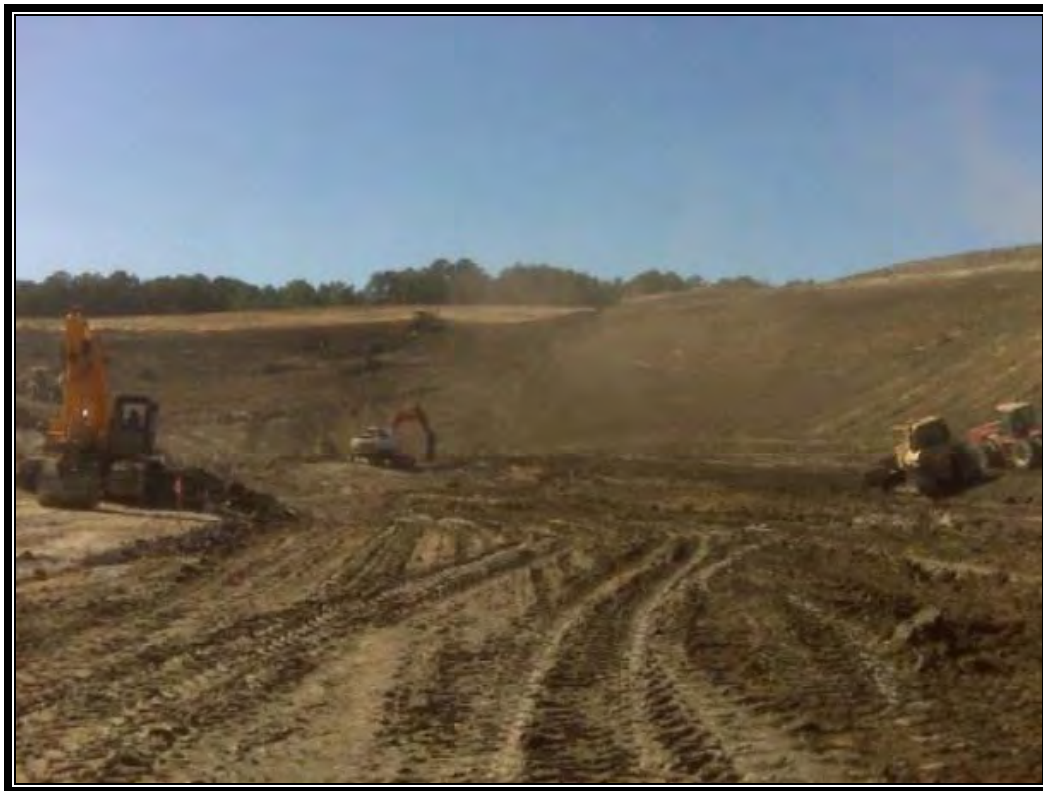
Excavating and grading subgrade in Cell 4
