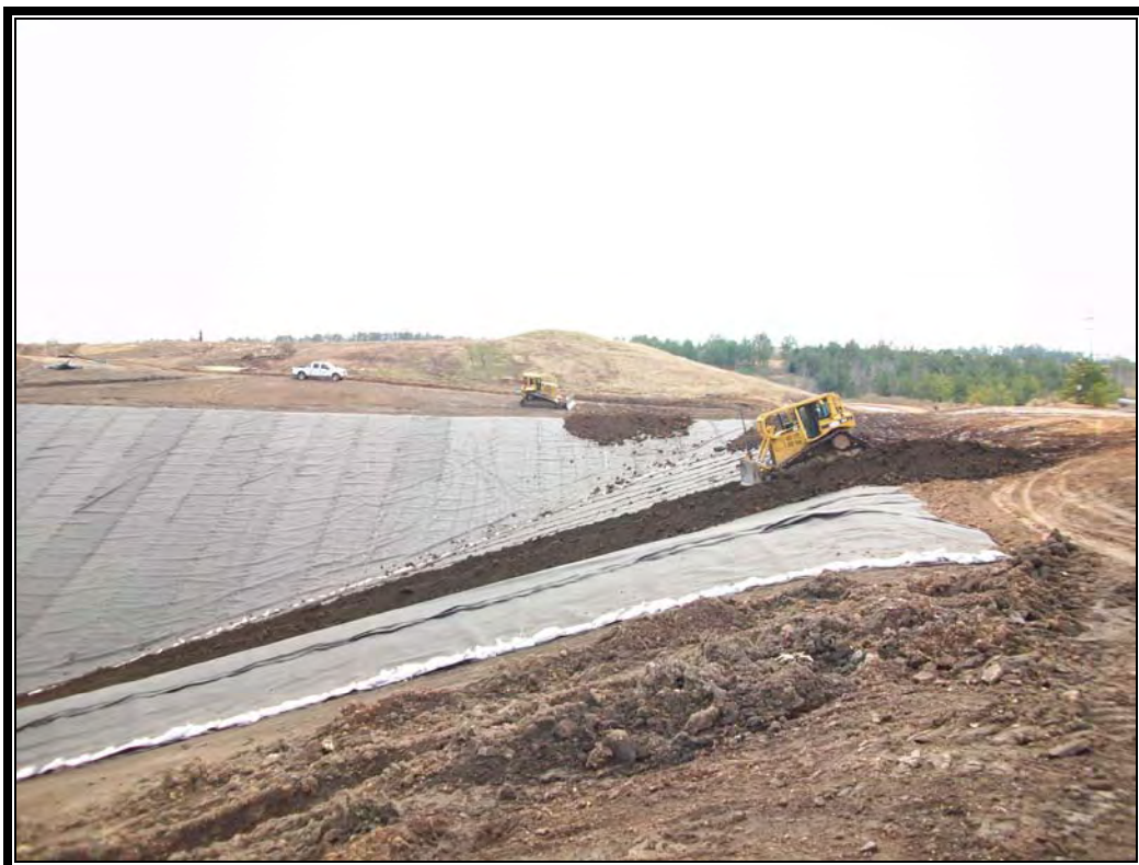
Placing protective cover material on west slope Cell 4
