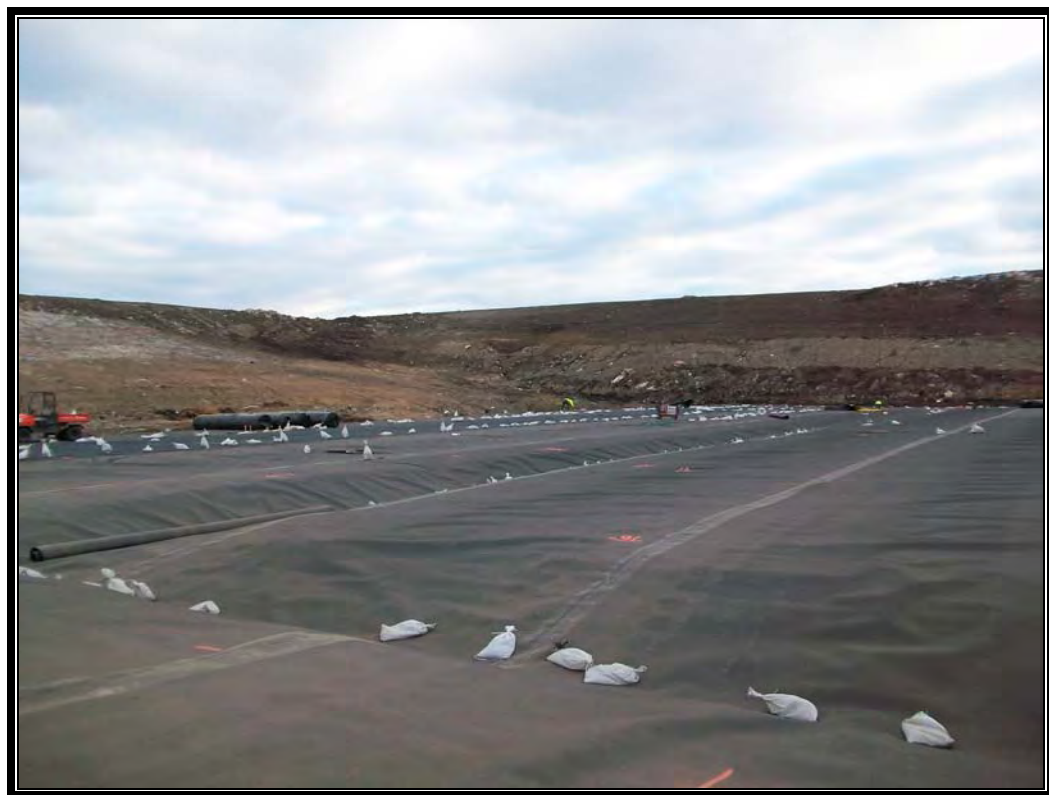
Looking southeast at installation of 60mil geomembrane on east half of Cell 4
