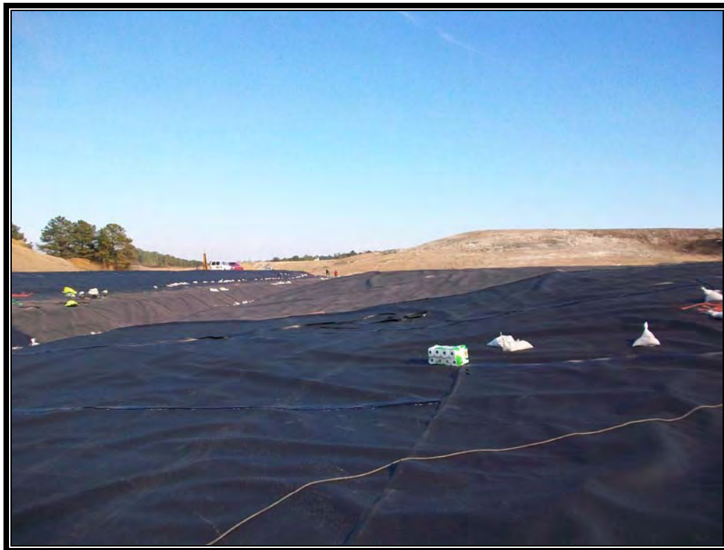
Looking east at placement of 8 ounce double sided geocomposite in Cell 4
