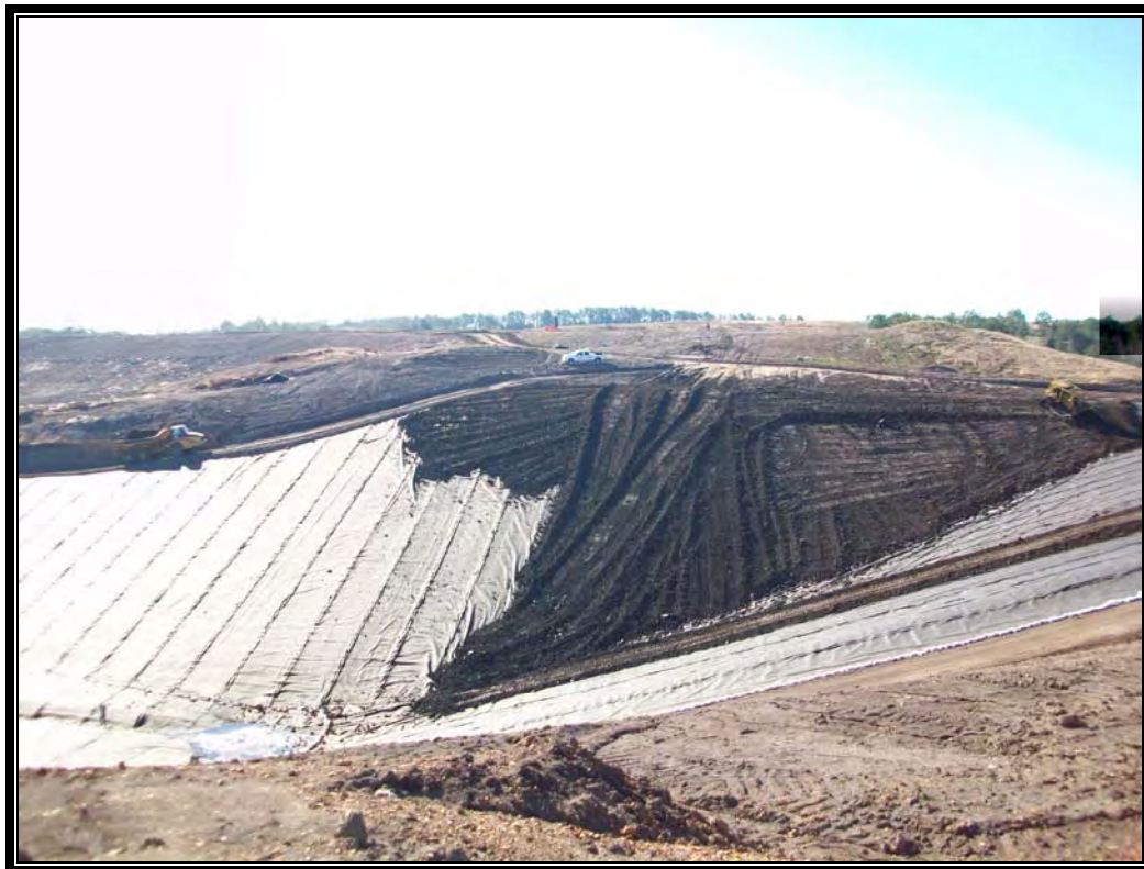
Placing protective cover material on south slope of Cell 4
