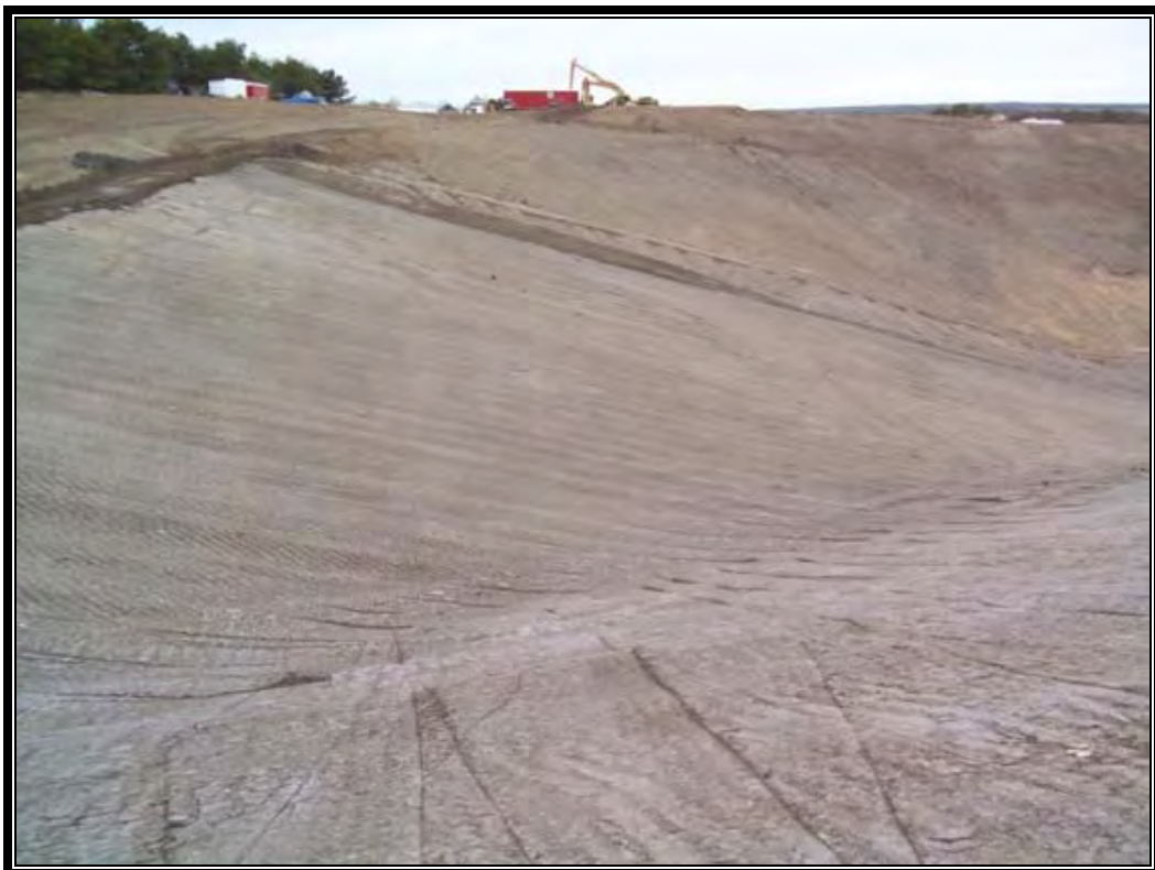
Completed prepared subgrade on west and south slopes of Cell 4
