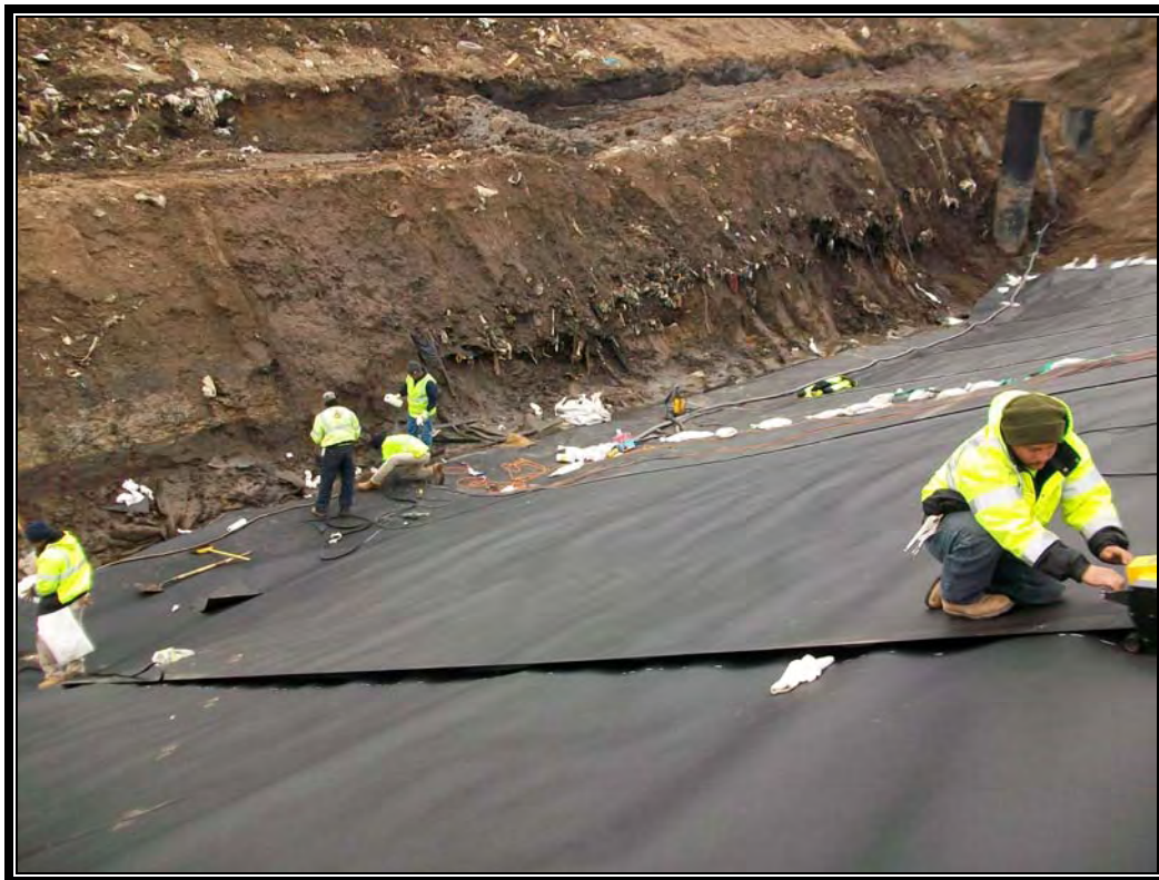
Liner tie-in between Cell 2 (Zones 1 & 2) and Cell 4
