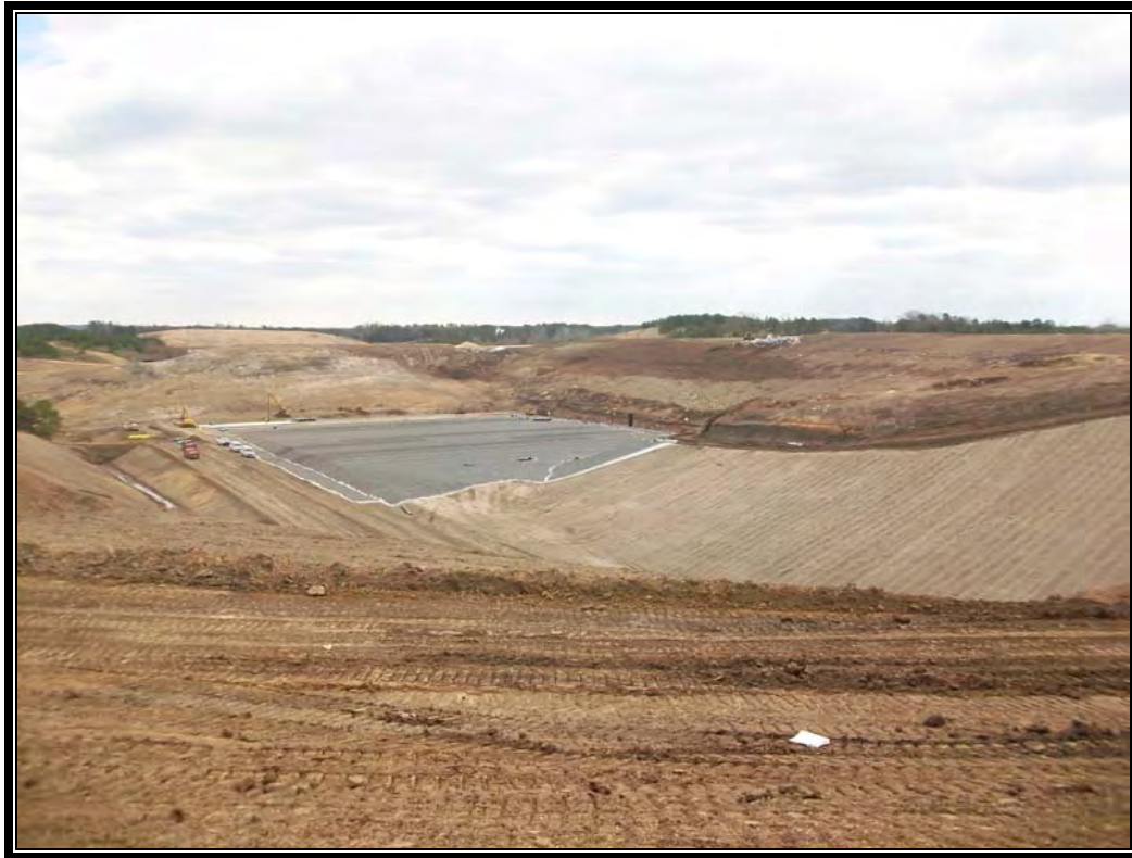
Looking east at installed GCL and 60mil geomembrane on east half of Cell 4
