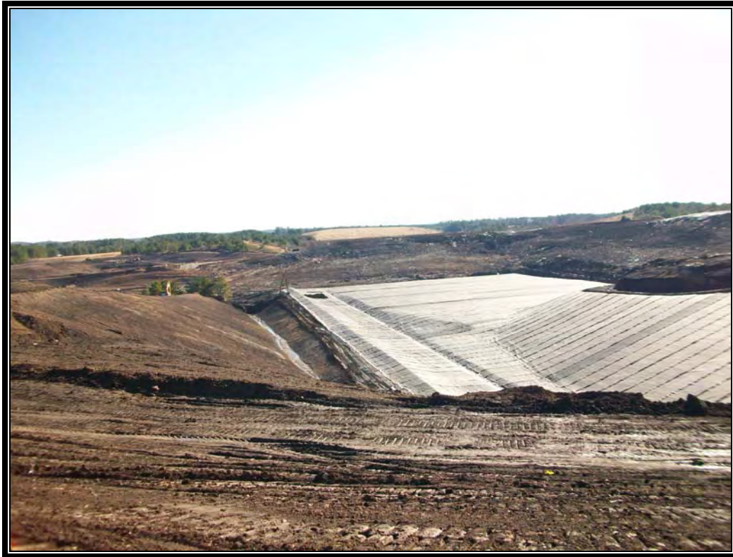
Looking east at completed liner system in Cell 4
