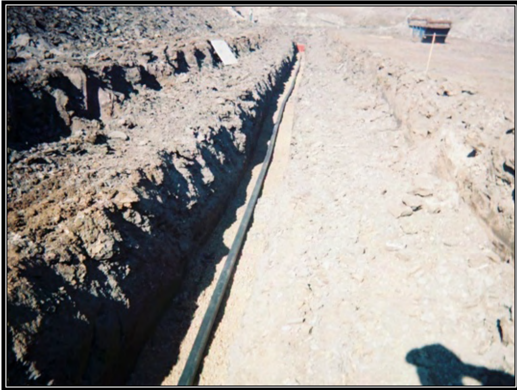
Installation of under-drain lateral in Cell 4
