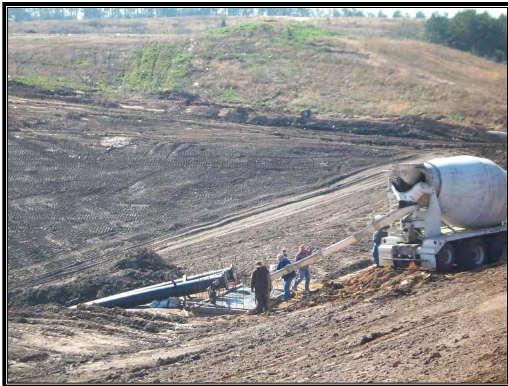
Pouring concrete base for leachate headwall
