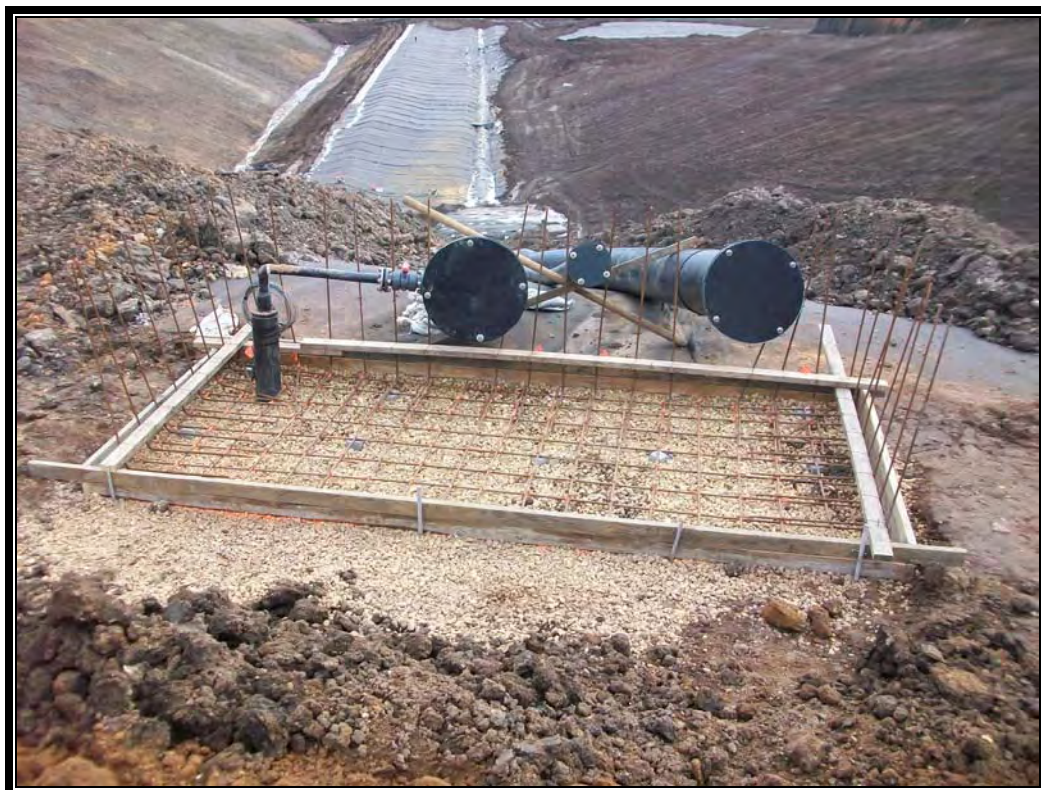
Forming up Leachate Headwall at west end of Cell 4
