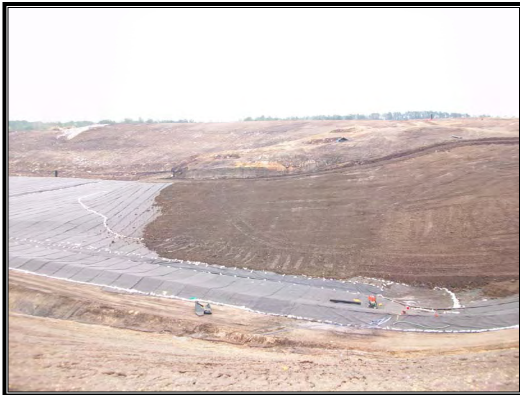
Placement of protective cover on south slope of Cell 4
