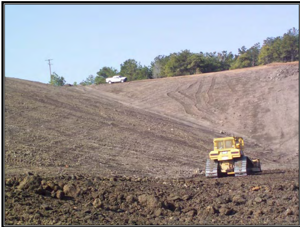
Placing and grading of prepared subgrade
