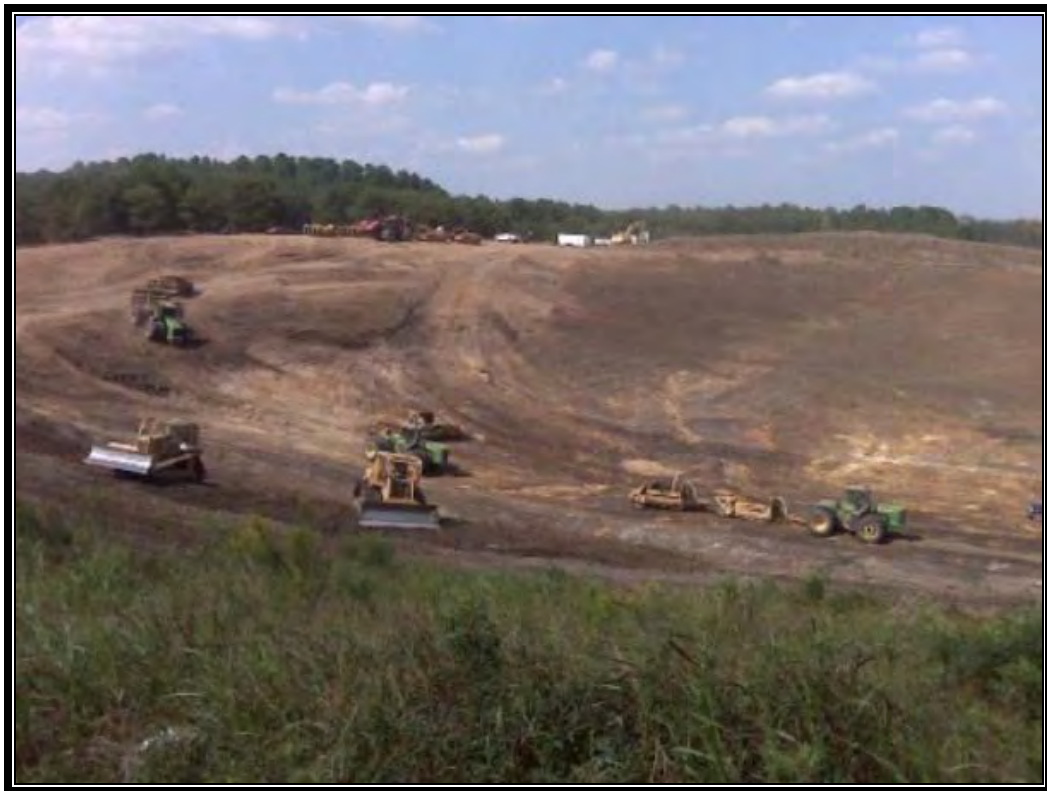
Looking north at excavation of Cell 4
