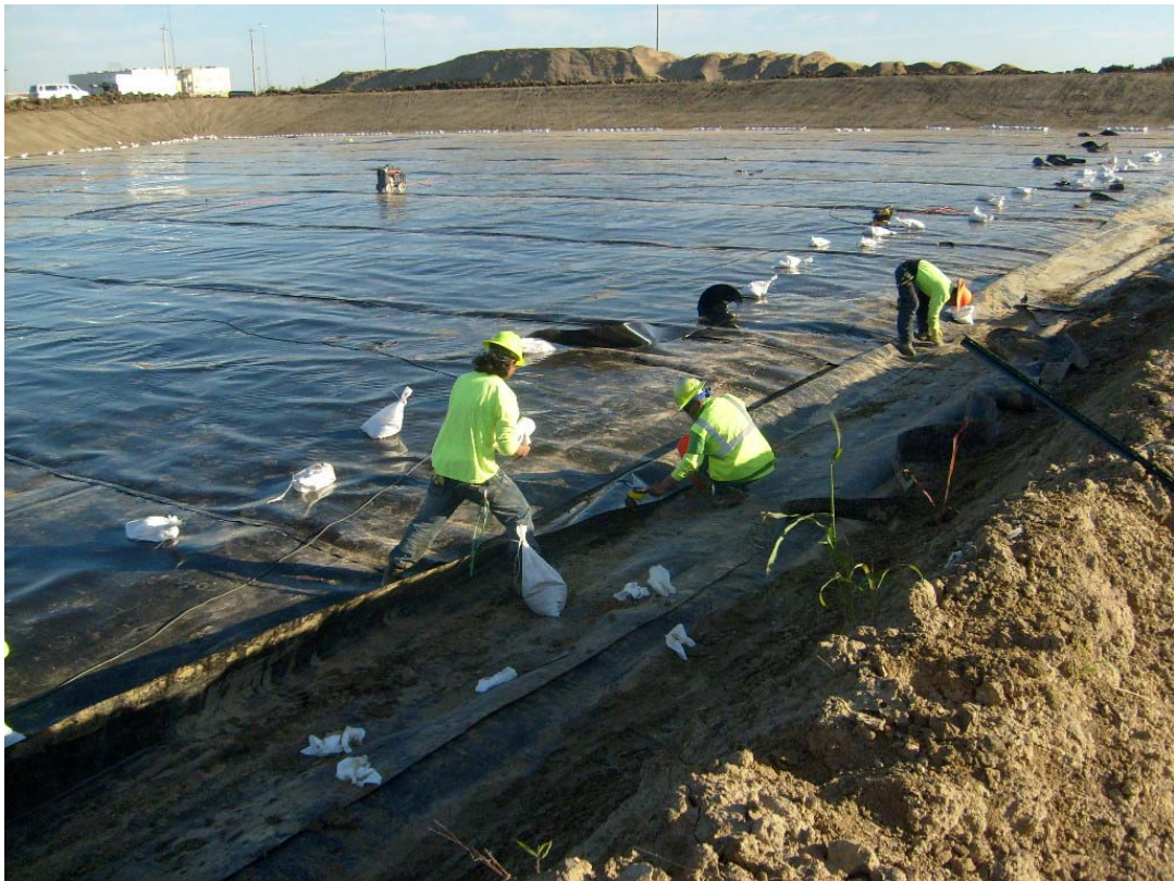
Photo 8. Looking northeast: geomembrane tie-in of Cell 13 with Cell 14.
