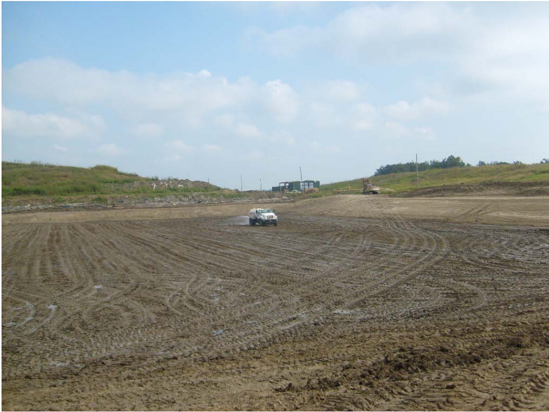
Photo 3. Looking north: clay liner installation.
