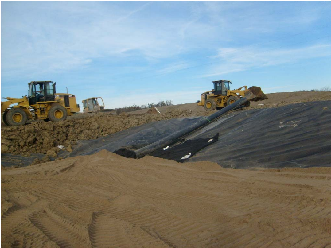
Photo 14. Installation of leachate collection riser pipe.
