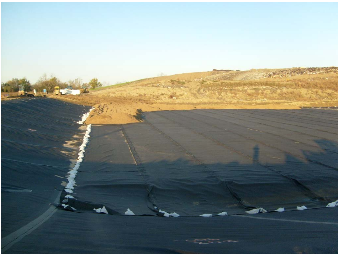
Photo 10. Looking west: installation of leachate drainage layer.
