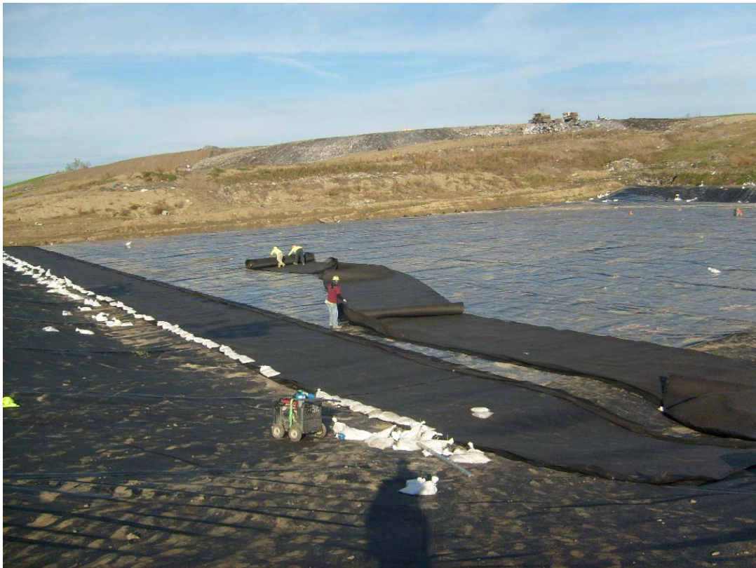
Photo 9. Looking west: installation of geotextile.
