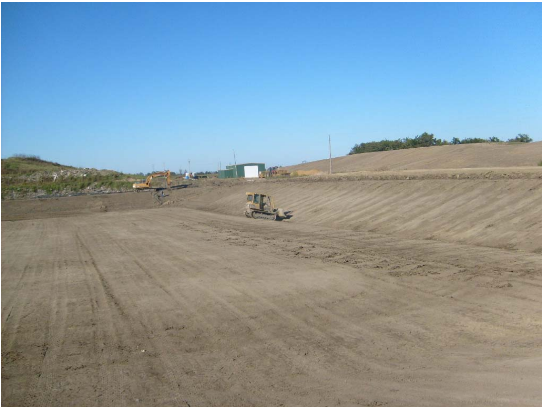
Photo 4. Looking north: clay liner installation in the leachate collection trench.
