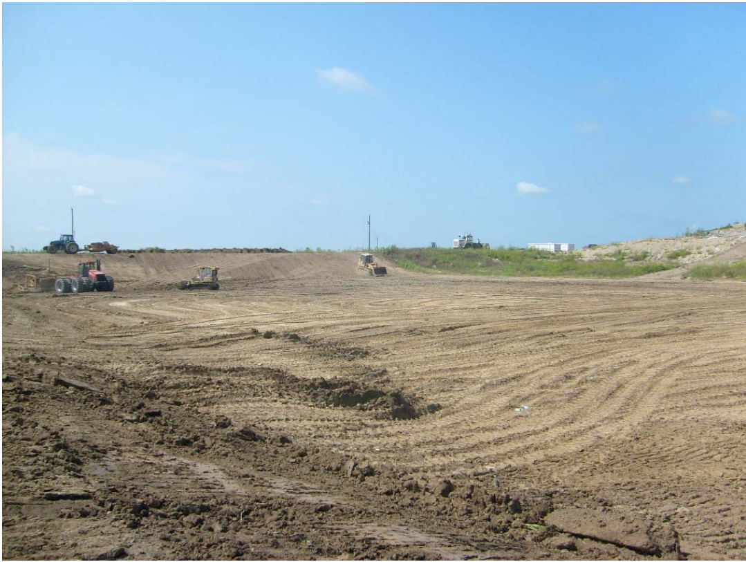
Photo 1. Looking south: subgrade preparation.
