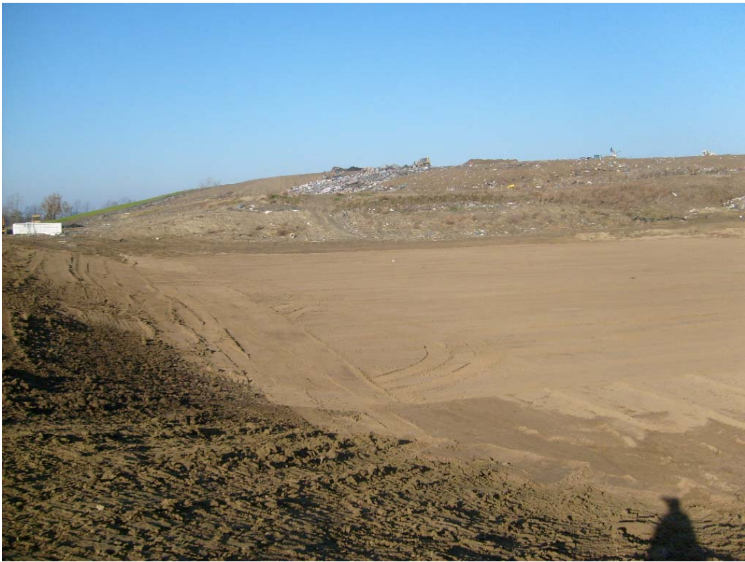
Photo 15. Looking west: installation of the protective cover layer.
