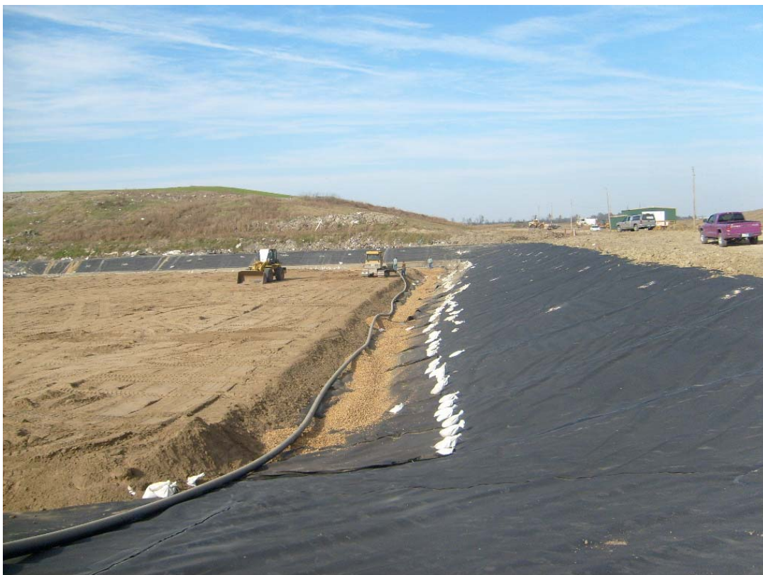
Photo 12. Looking north: installation of leachate collection pipe.
