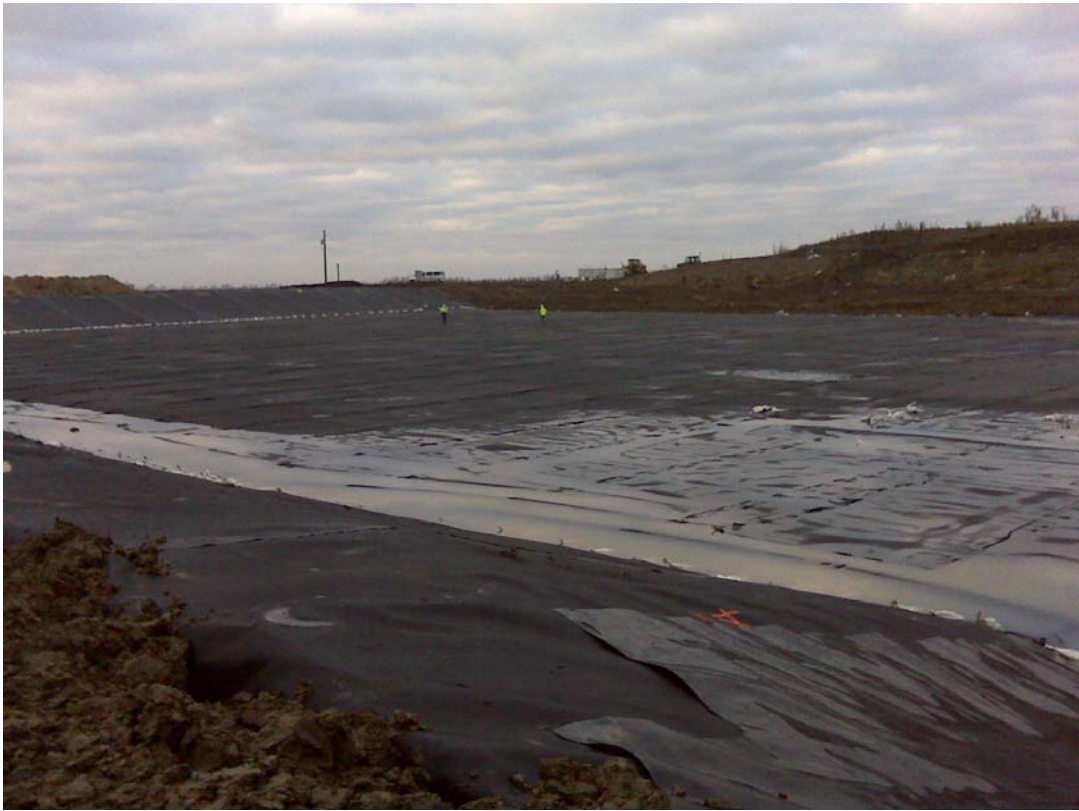
Photo 7. Looking southwest: completed geomembrane layout.
