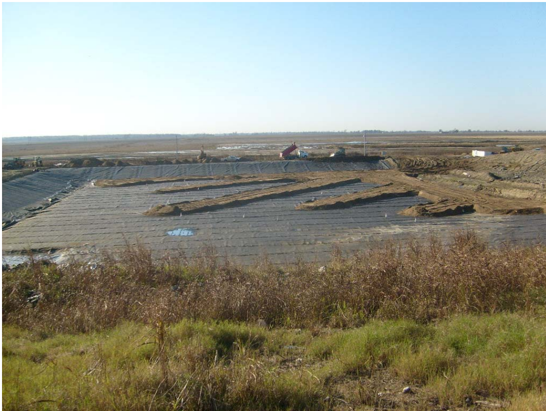
Photo 11. Looking south: installation of leachate drainage layer.
