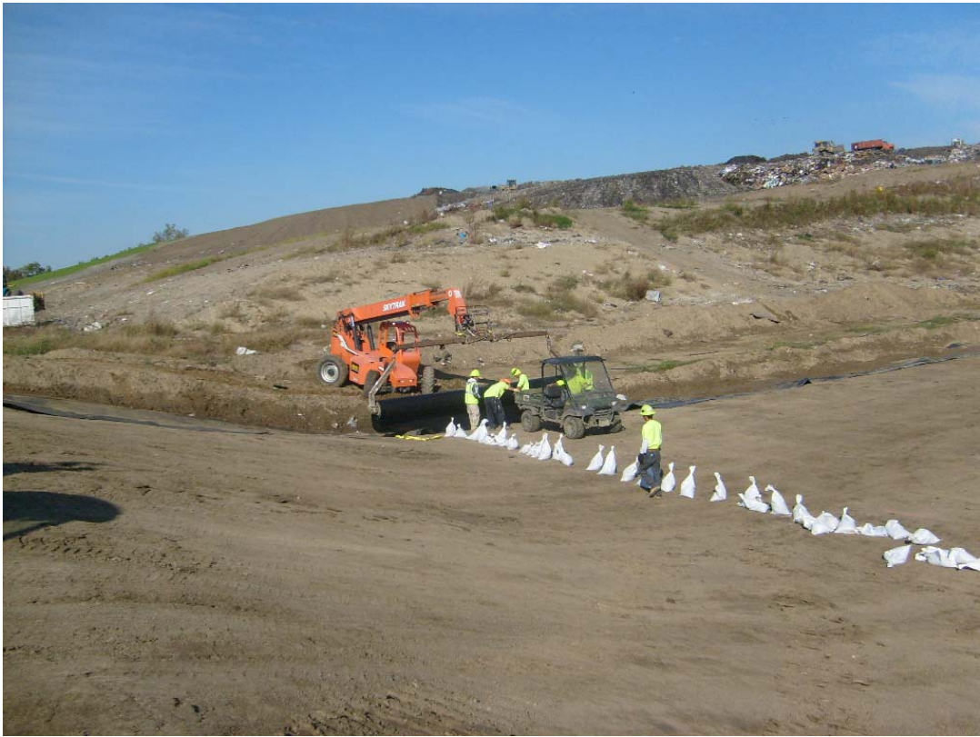
Photo 5. Looking west: installation of smooth geomembrane.
