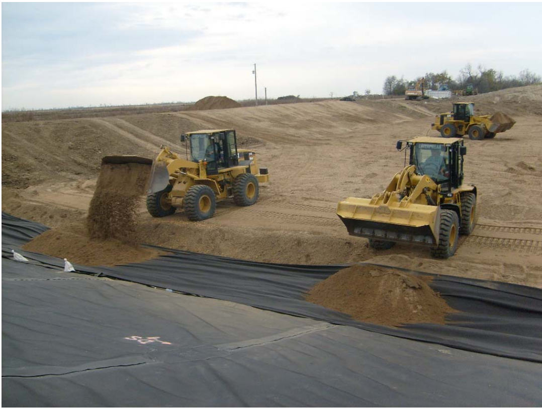
Photo 13. Installation of gravel on top of leachate collection trench.
