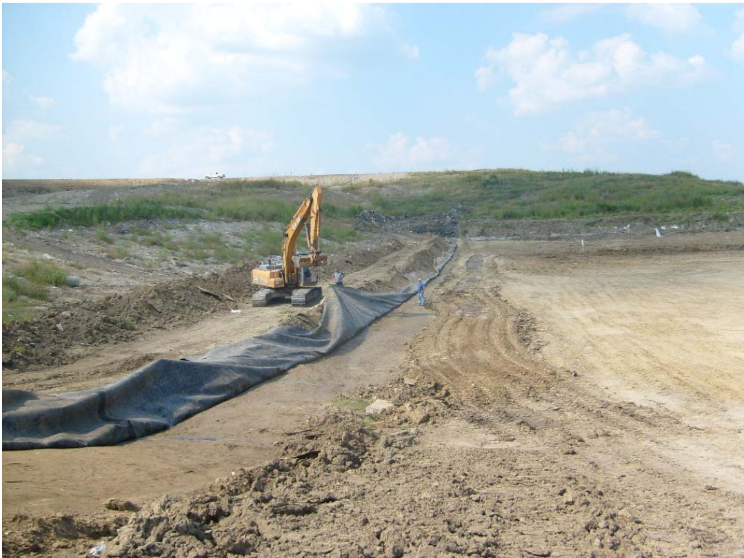
Photo 2. Looking north: pulling back Cell 13 geomembrane for tie-in to Cell 14.
