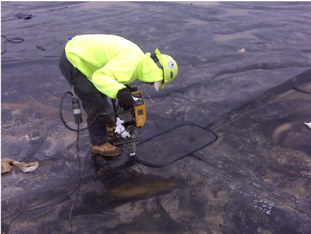
Photo 6. Fusion seaming on the geomembrane liner.
