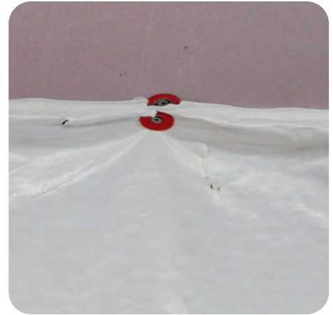
3. Seal seams of belly wrap
