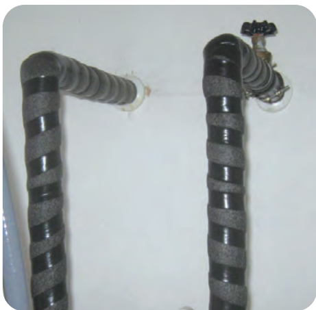
Secure seams with tape
