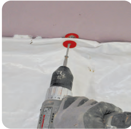
2. Attach new belly wrap
