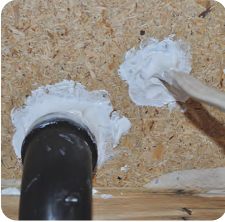
1. Ensure air sealing is complete
