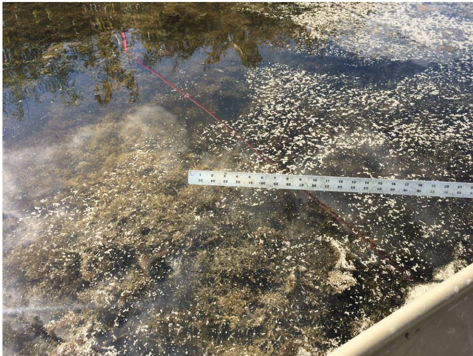
Photo 2 Organoclay Placement in the Heavily Vegetated Area
