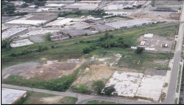
Heifer International World Headquarters site before remediation
