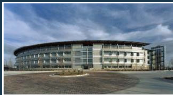
AFTER REMEDIATION AND CONSTRUCTION
