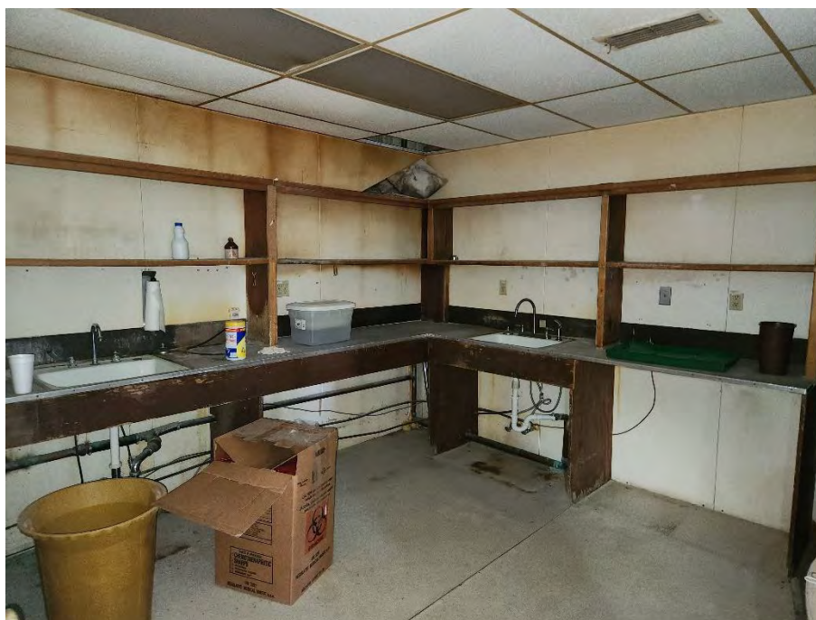
Photo 3: This photograph shows the asbestos-containing material (ACM) cream sheet vinyl flooring and black mastic (MA-SV01) found in the northern hallway and various dental exam rooms of the Medical Arts building.
