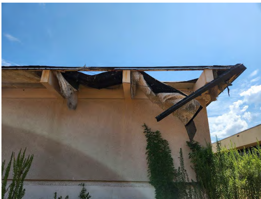
Photo 7: This photograph shows a closeup view of the assumed ACM roofing material on the Medical Clinics building and its damage.
