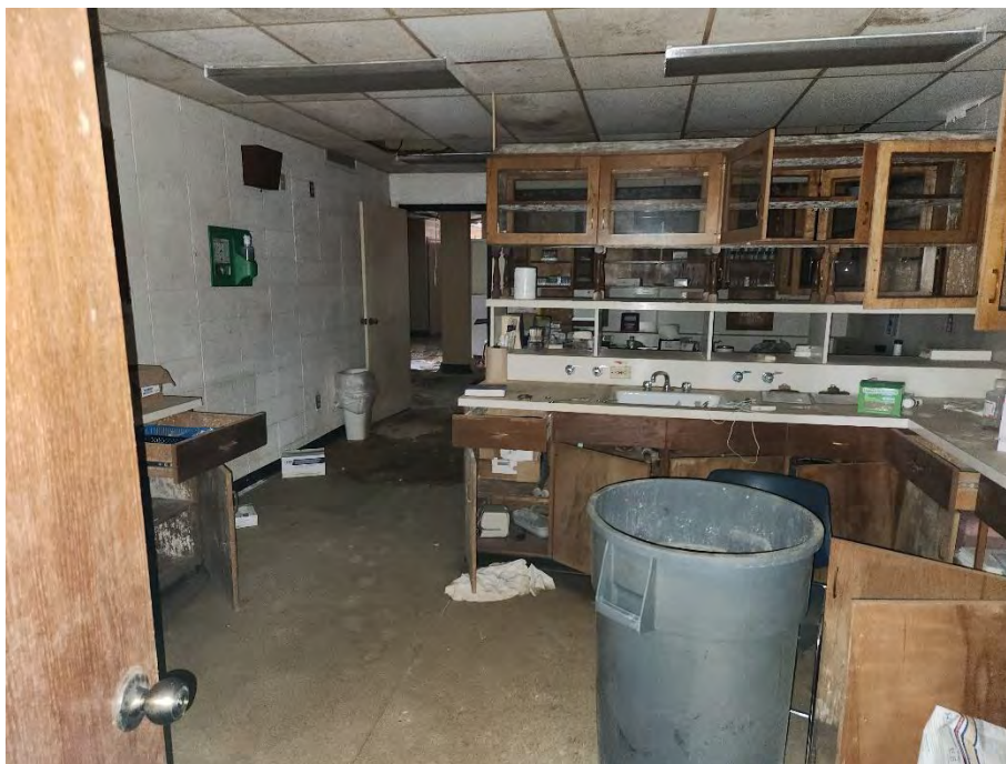
Photo 5: This photograph shows ACM cream sheet vinyl flooring and white mastic (MC-SV02) found in the laboratory room and rooms off the main hallway of the Medical Clinics building.
