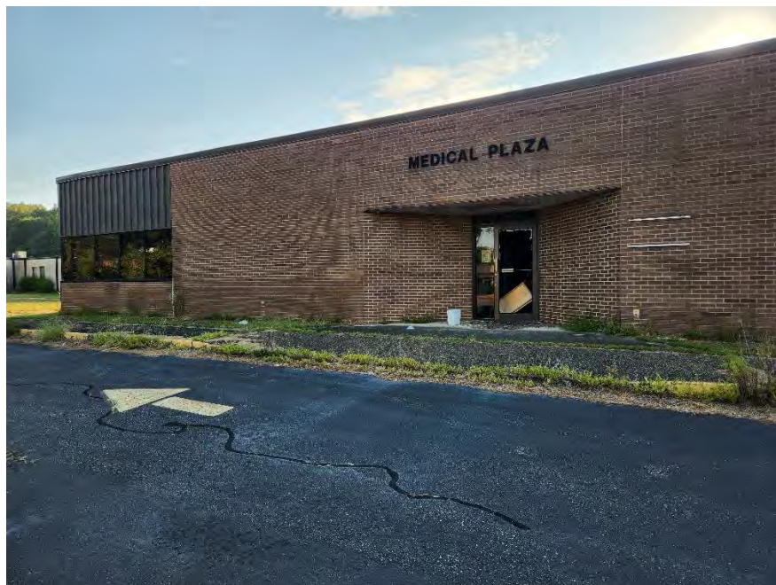
Photo 2: This photograph shows the side entrance of the Medical Plaza building.
