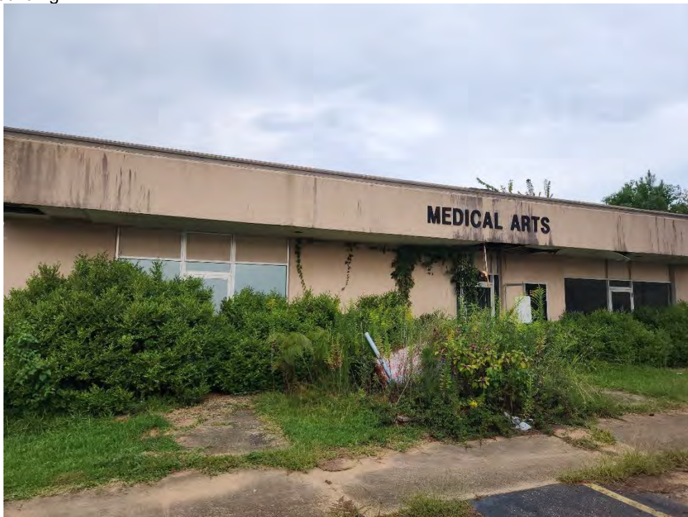
Photograph 40 (Northwest): View of the front of the Medical Arts building.
