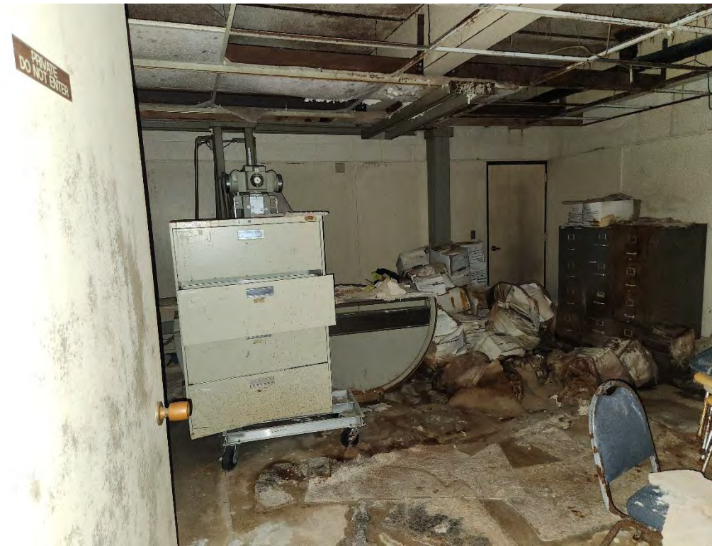
Photograph 37 (Overview): View of the x-ray office in the Medical Clinics building.
