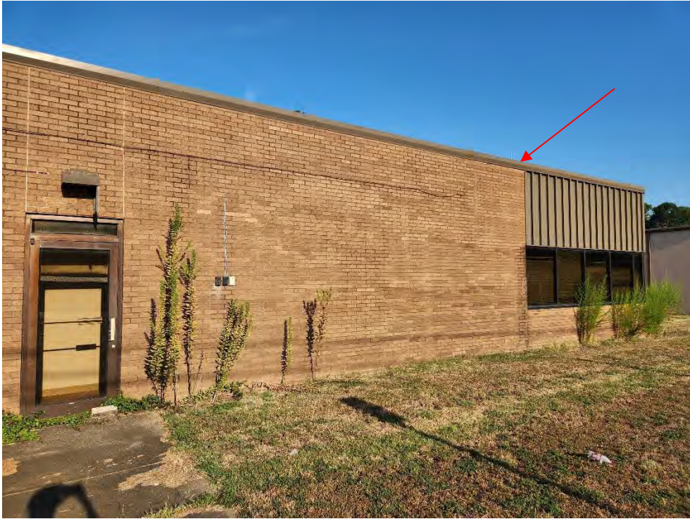
Photo 11: This photograph shows a view of assumed ACM roofing material on the Medical Plaza building (red arrow).
