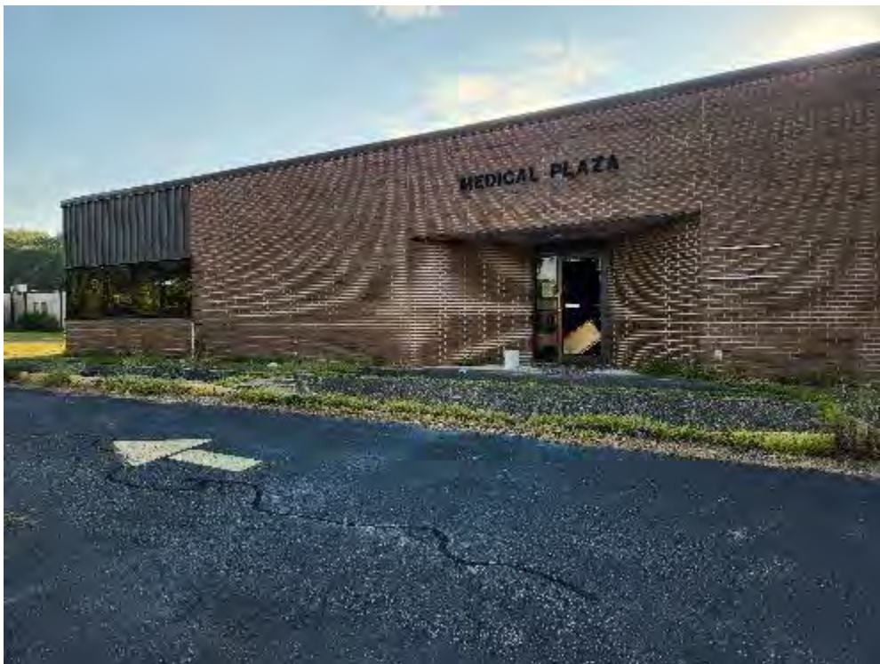
Photograph 46 (Northeast): View of west side of the Medical Plaza building.
