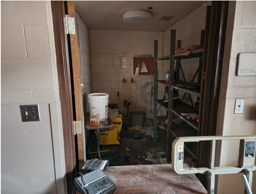
Photograph 3 (South): View of one of the utility closets in the Hospital building, with a 5-gallon container of floor cleaner.
