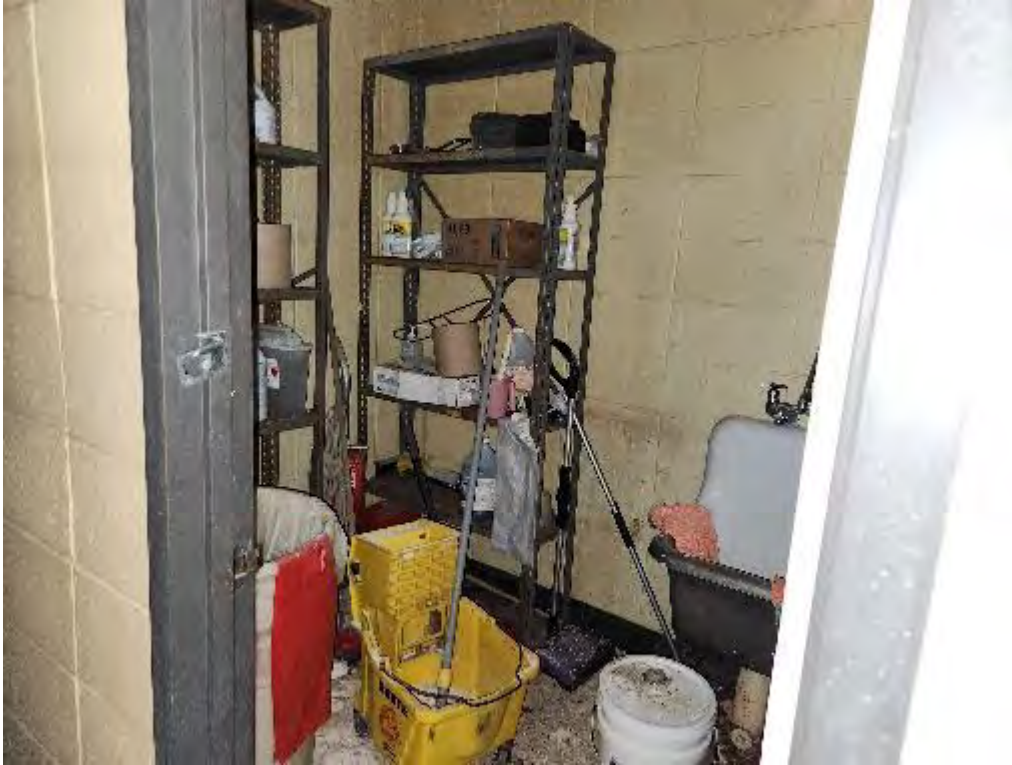
Photograph 21 (Overview): View of utility closet along the back hallway of the Medical Clinics building.
