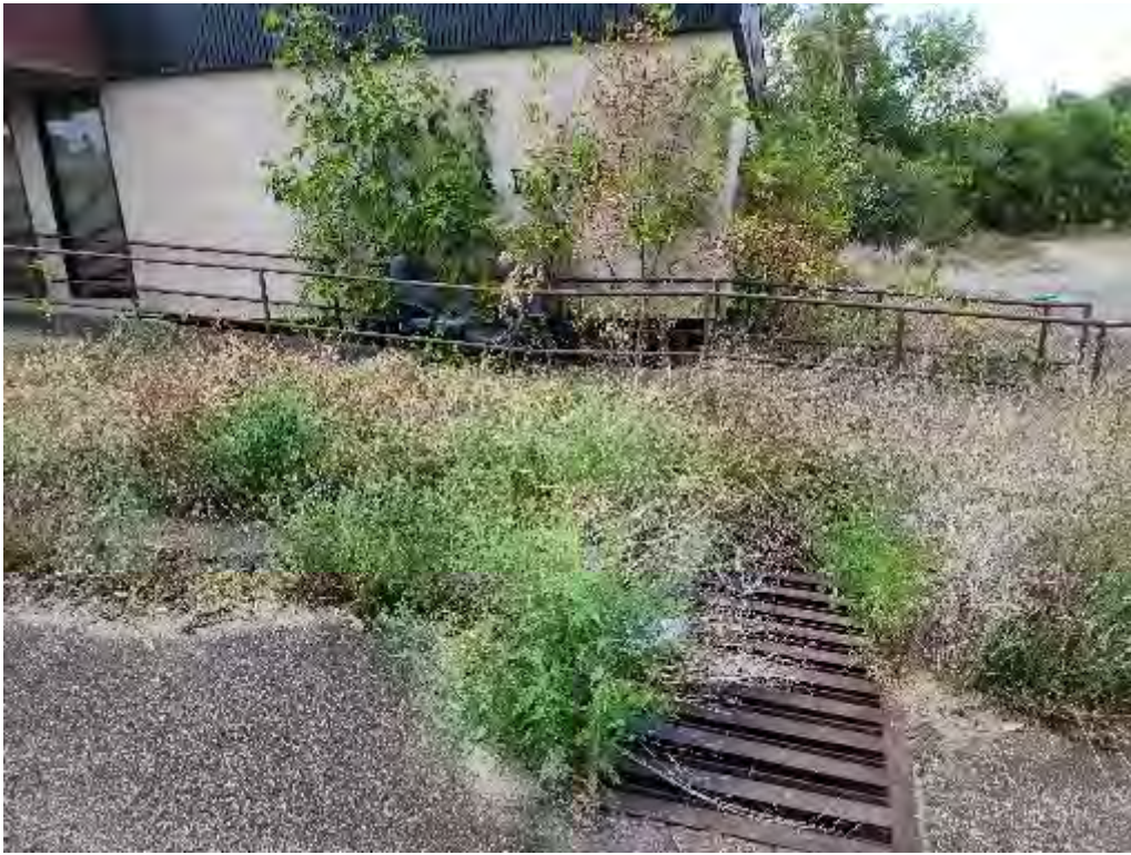
Photograph 17 (West): View of rain runoff drain in front of subject property building.
