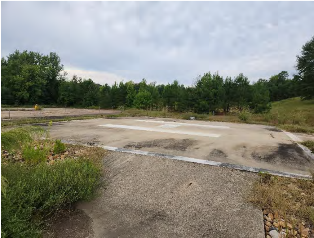
Photograph 29 (West): View of the helicopter landing pad, with de minimis staining.
