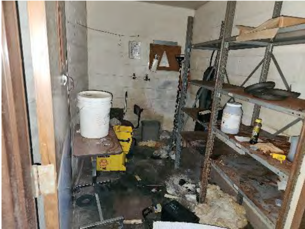
Photograph 9 (NA): View of a utility closet off of the kitchen area in the main Hospital building.
