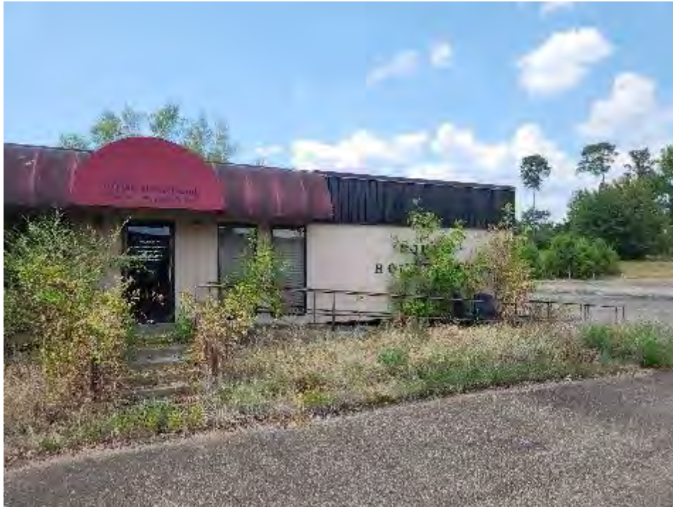
Photograph 1 (Northwest): View of the front of the subject property building.
