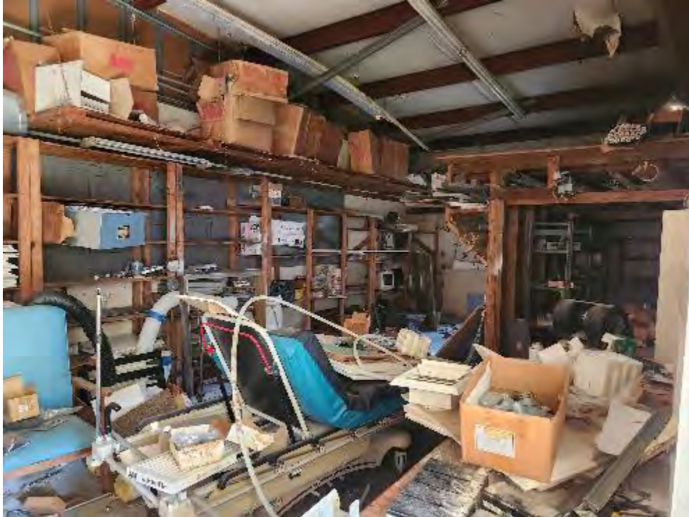
Photograph 41 (West): View of previous workshop area on the north side of the Purchasing Department building, currently filled with old hospital equipment.
