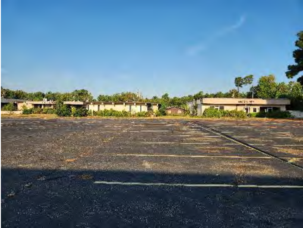
Photograph 1 (West): View of entire subject property with the Medical Arts building on the right (north), and the Medical Clinics building on the left (south).
