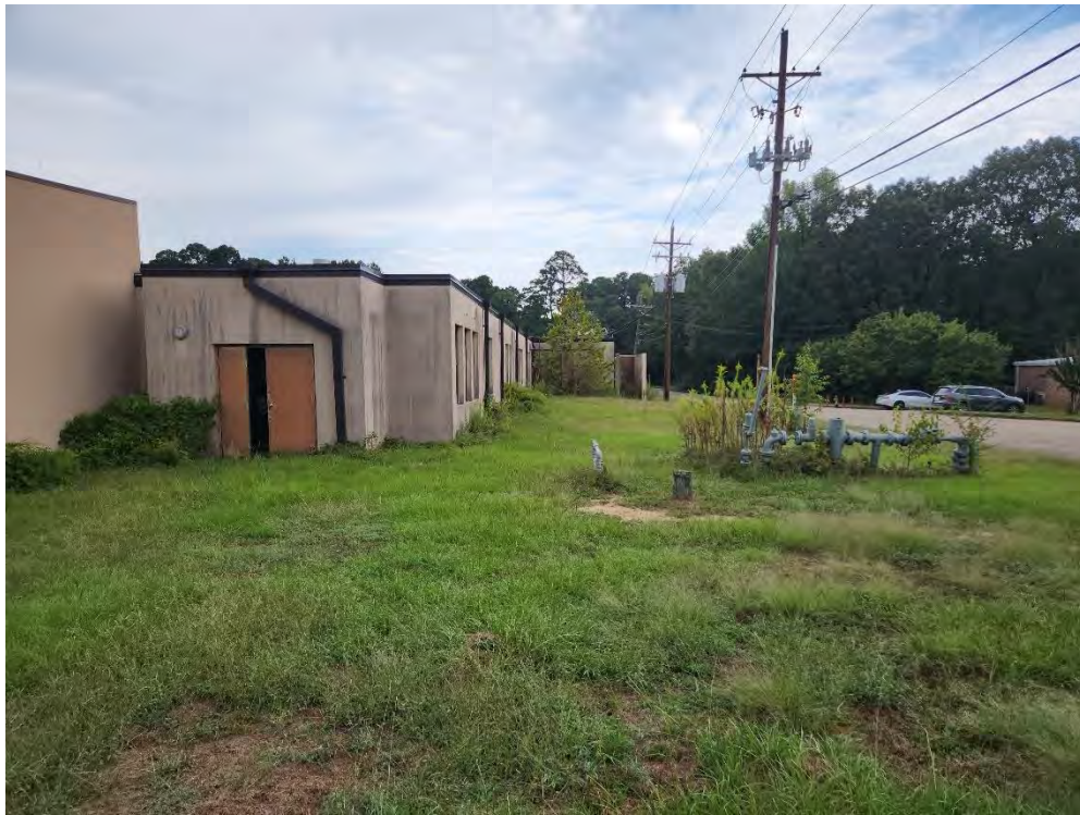
Photograph 47 (North): View of natural gas risers and pole-mounted transformers on the eastern side of the Hospital building.
