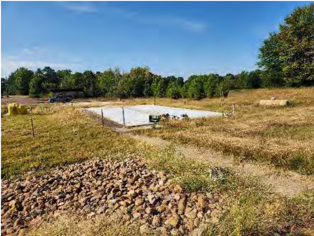
Photograph 23 (Southwest): View of cement pad for former helicopter hangar.
