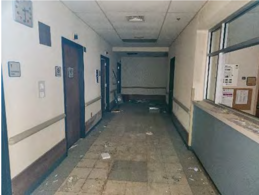
Photograph 3 (East): View of emergency room hallway in the Hospital building.
