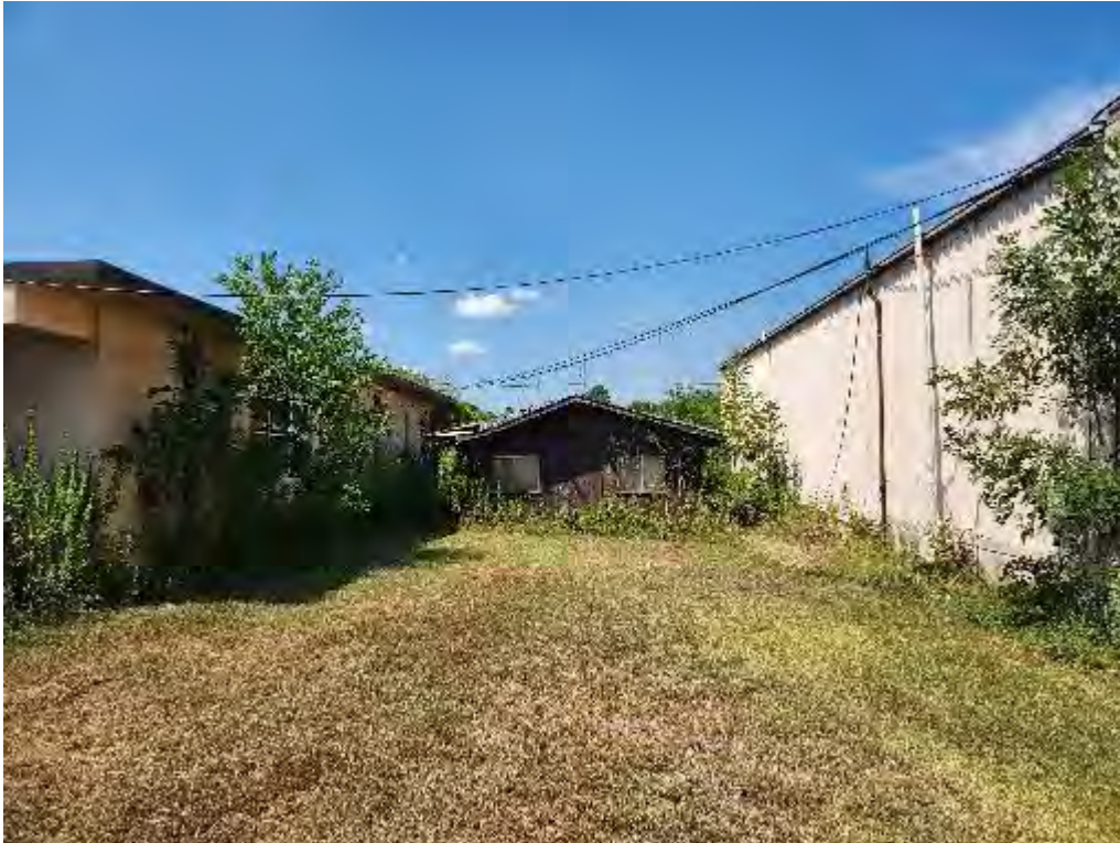
Photograph 15 (West): Front view of collapsed wooden structure between the Medical Arts building (right) and the Medical Clinics building (left).
