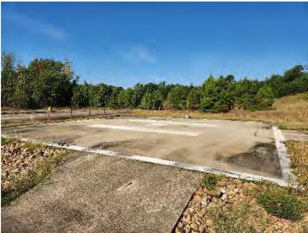
Photograph 28 (Southwest): View of helicopter landing pad.
