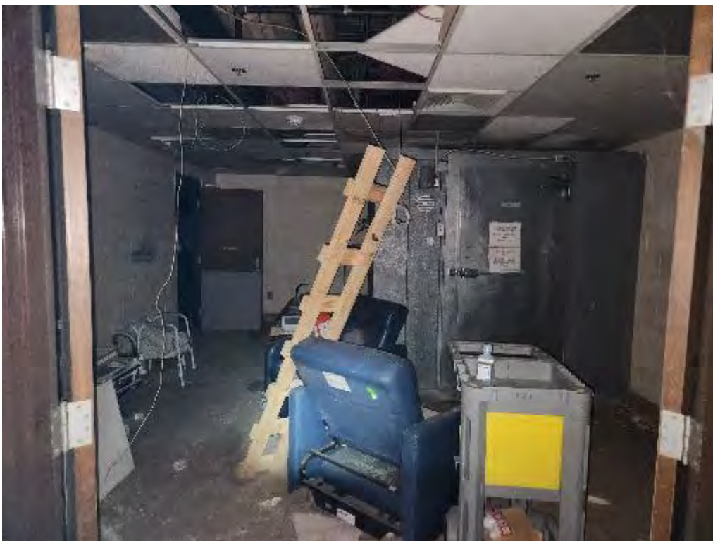
Photograph 12 (NA): View of walk-in freezer next to the kitchen in the main Hospital building.
