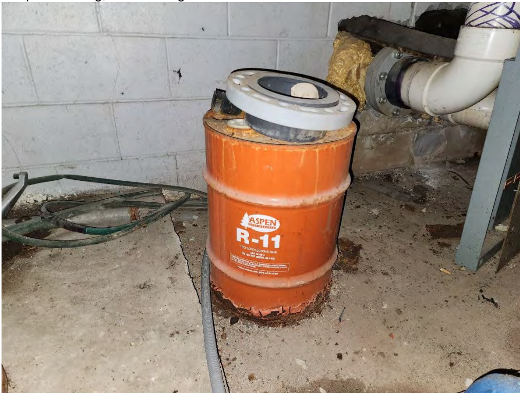
Photograph 14 (South): View of the metal drum of trichlorofluoromethane (Freon-11) in the boiler room of the Hospital building.
