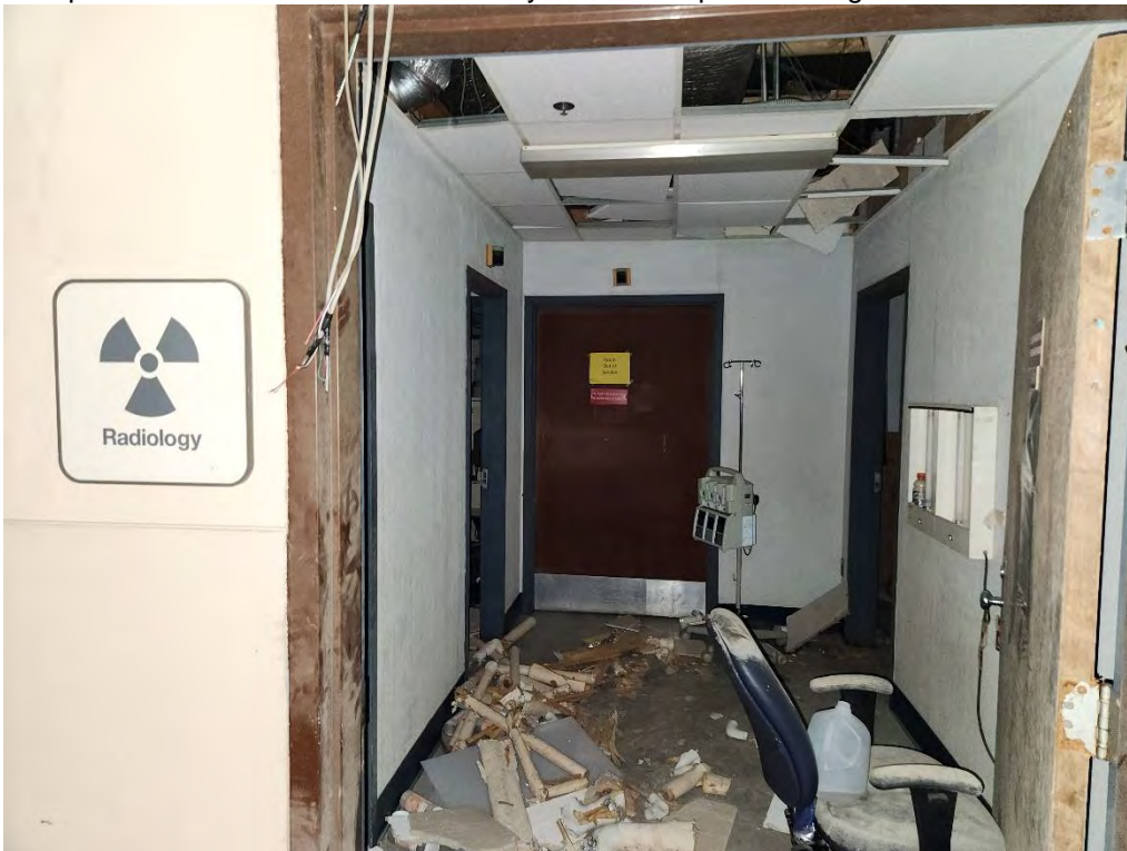
Photograph 6 (South): View of the x-ray room in the Hospital building.
