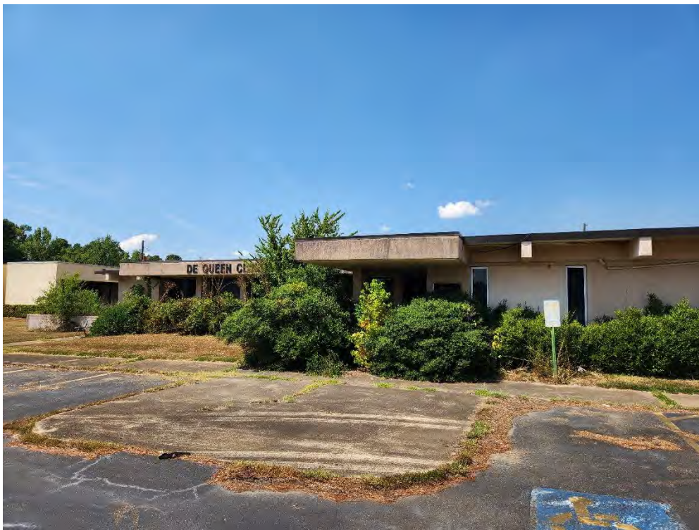
Photo 2: This photograph shows the east side of the Medical Clinics building.
