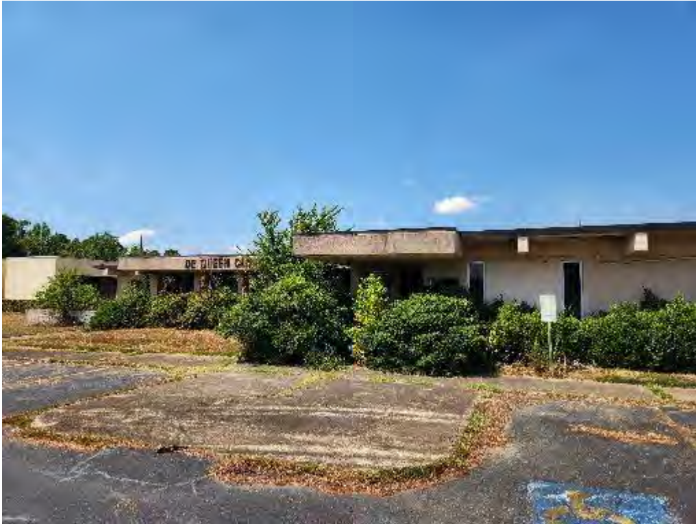
Photograph 17 (West): View of the front of the Medical Clinics building.
