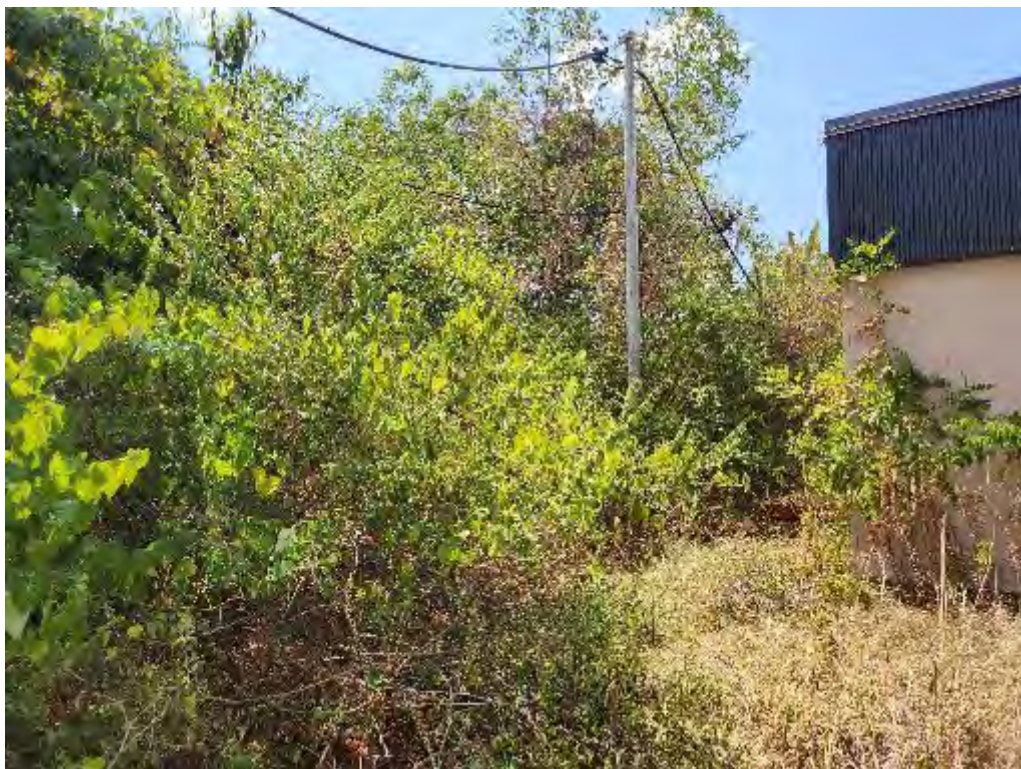
Photograph 16 (Southwest): View of the northeast corner of the subject property building with power lines visible connecting to the building.
