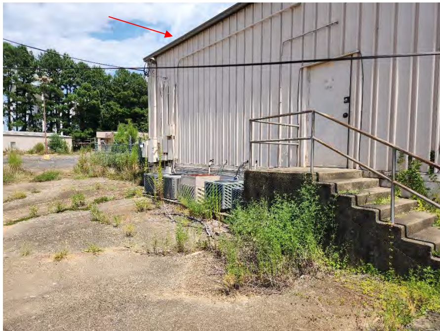
Photo 8: This photograph shows a view of assumed ACM roofing material on the Medical Arts building (red arrow).
