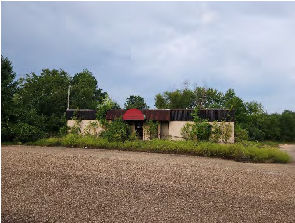
Photograph 23 (West): View of the front of the De Queen MC Emergency Medical Services (EMS) building.
