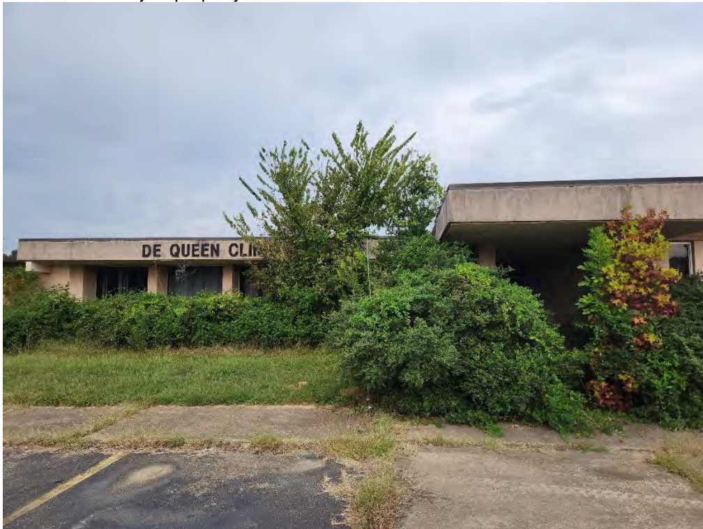
Photograph 34 (West): View of the front of the Medical Clinics building.
