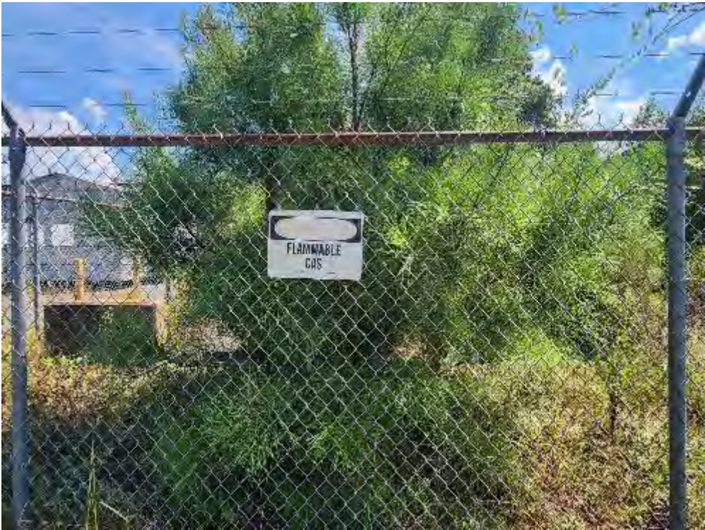
Photograph 34 (East): View of fenced off area on the west side of the Hospital building.
