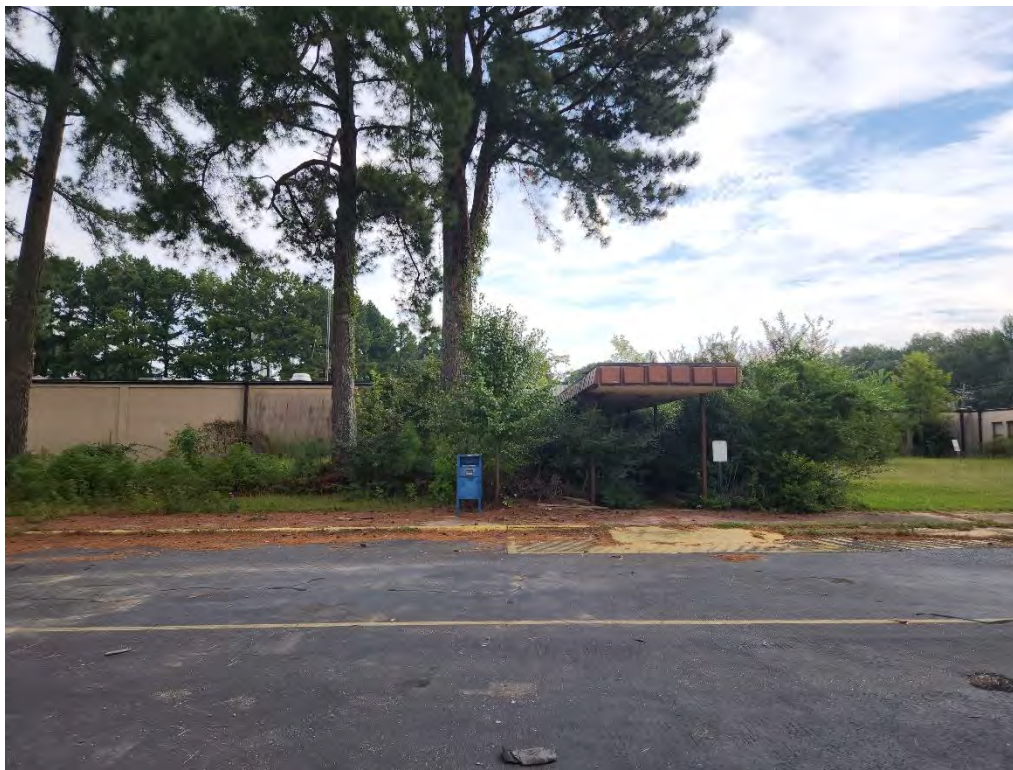
Photograph 1 (North): View of the front (south side) of the Hospital building.
