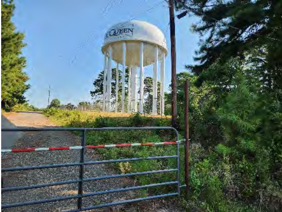
Photograph 45 (North): View of the De Queen water tower northwest of the subject property boundary.
