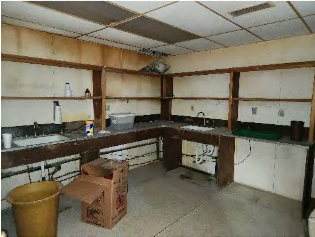
Photograph 7 (Overview): View of former sink area and prep area in the back northwest corner of the Medical Arts building.
