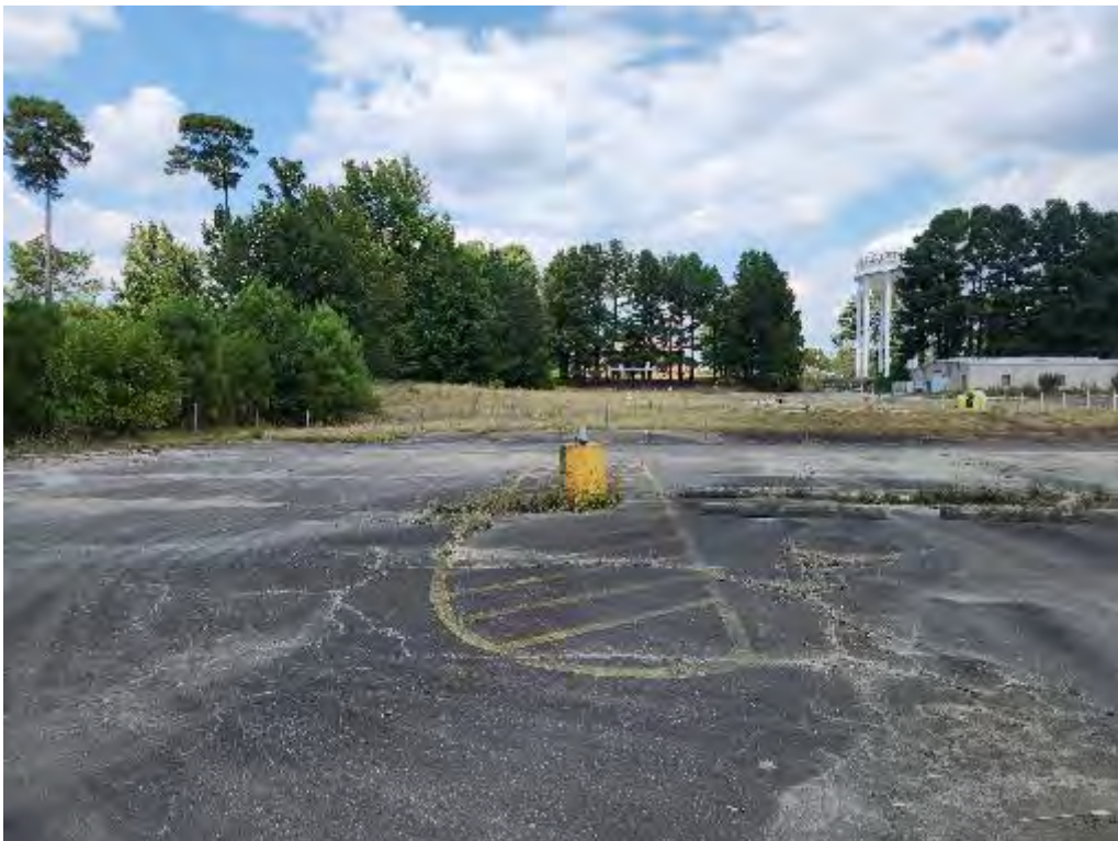
Photograph 20 (North): View of the southern parking lot adjoining the subject property building.
