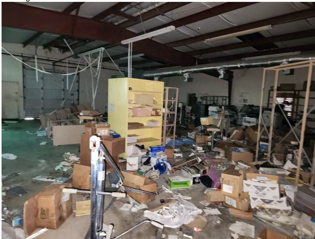
Photograph 12 (Northwest): View of the garage of the Purchasing Department building.
