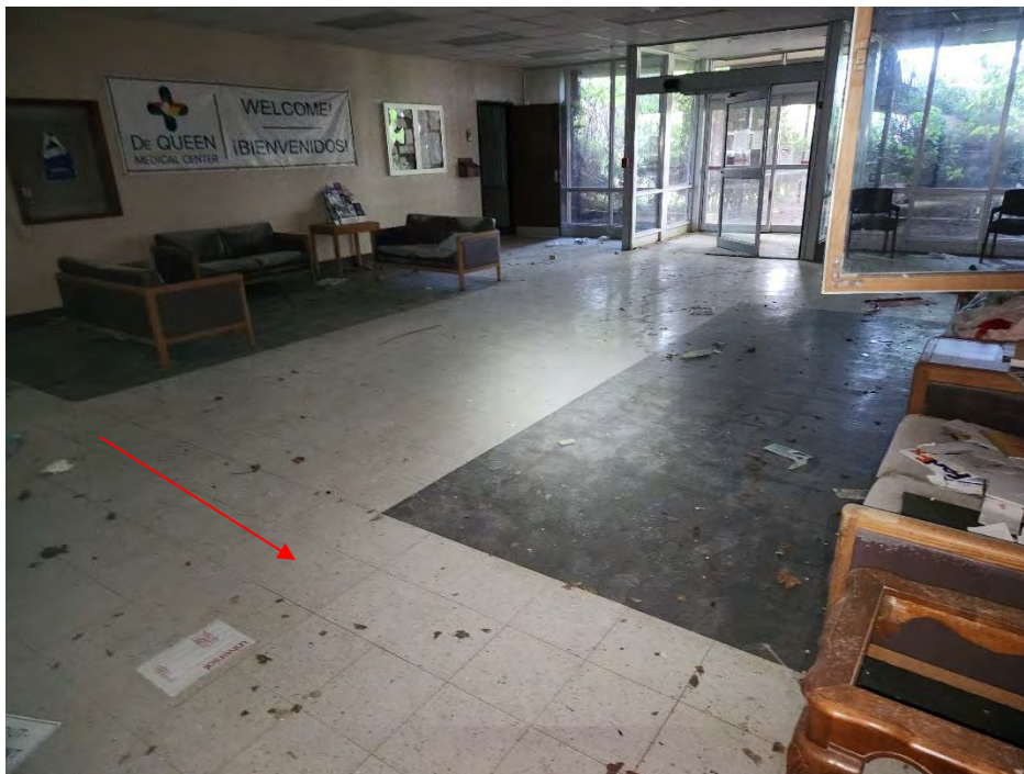
Photo 4: This photograph shows the asbestos-containing material (ACM) 12- x 12-inch white with green and gray streak vinyl floor and black mastic (HS-VFT03) in the front entryway of the Hospital building (red arrow).
