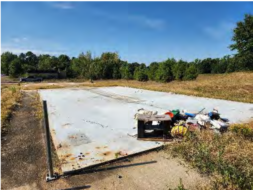
Photograph 24 (Southwest): View of slab and building footprint of the former helicopter hangar.
