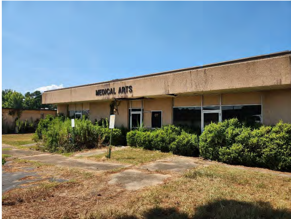
Photo 1: This photograph shows the east side of the Medical Arts building.
