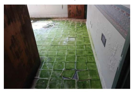
Photo 10. Interior of structure note mold and moss growth.
