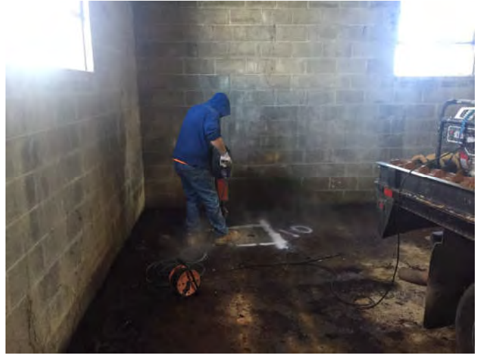
Photo 2. Jackhammering for flush-mount manhole cover, MW-1.
