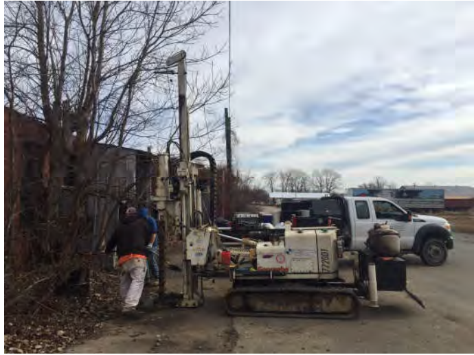
Photo 1. Track-mounted Geoprobe unit used for soil sampling and monitoring well installation, B-16 (MW-4).
