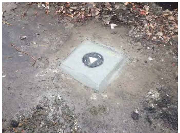
Photo 4. Flush-mount surface completion, MW-4.
