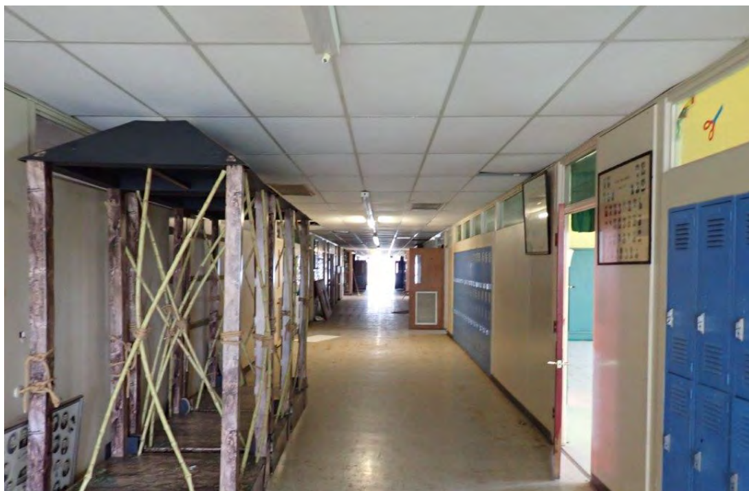
Photograph 14. Classroom building #7380 view of interior corridor
