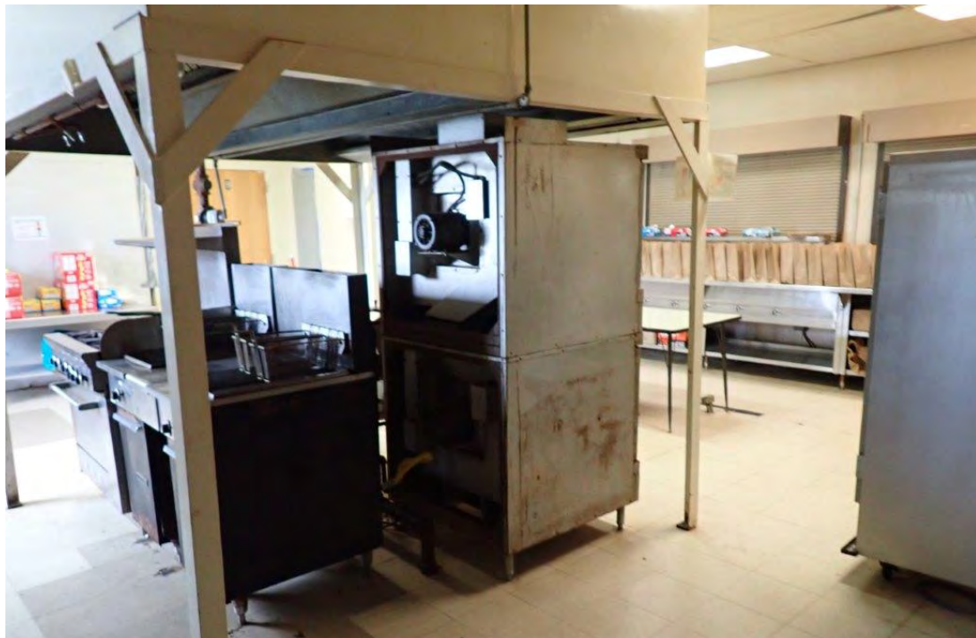
Photograph 27. Cafeteria building #7381 view of kitchen
