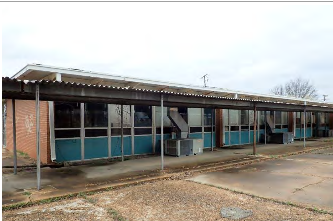
Photograph 2. View of classroom building #7380 from east side
