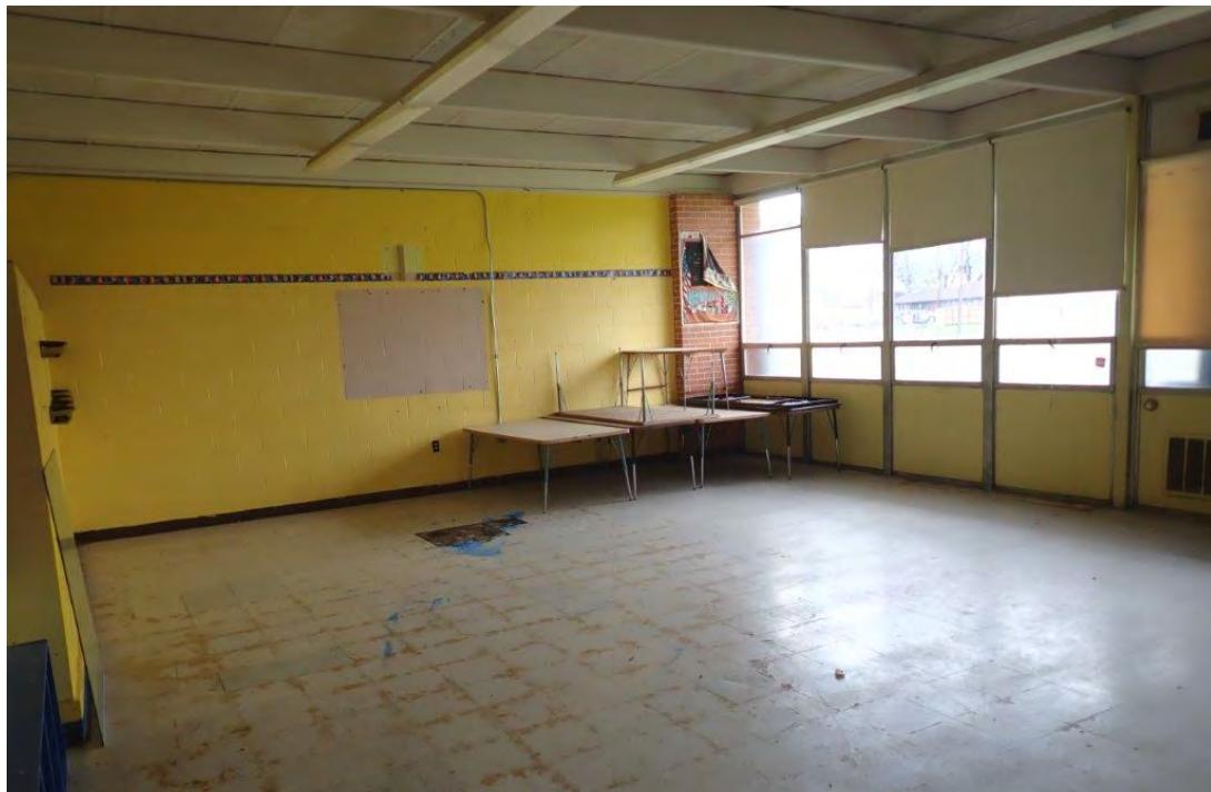
Photograph 15. Classroom building #7380 view of typical classroom
