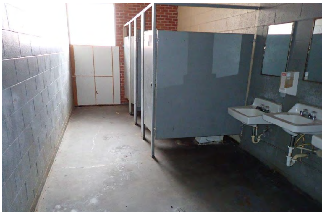
Photograph 18. Classroom building #7380 view of girls bathroom
