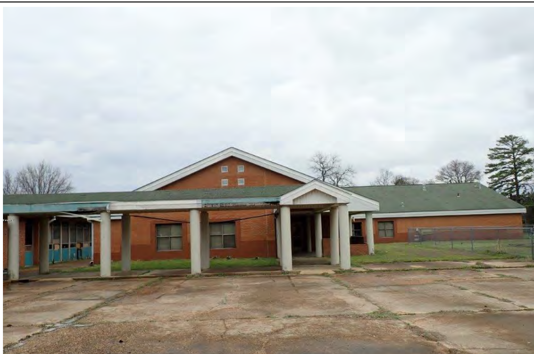
Photograph 4. View of cafeteria and classroom building #7381 from south side
