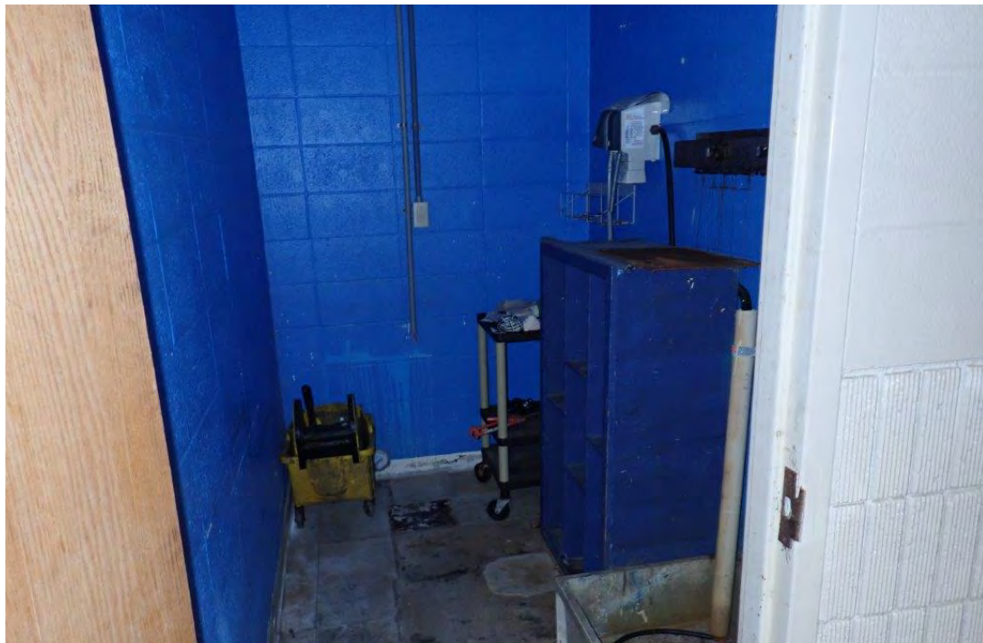
Photograph 33. Cafeteria building #7381 view of janitorial closet
