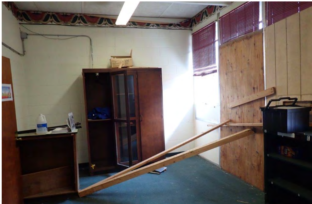
Photograph 17. Classroom building #7380 view of administrative office
