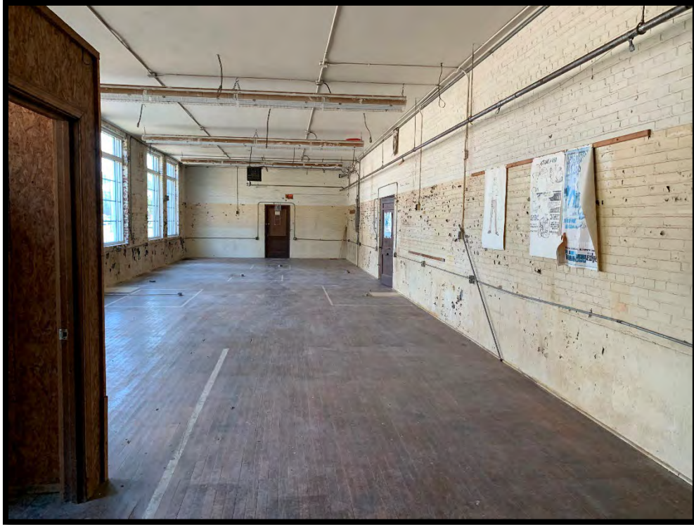
Photograph 15: View of classroom in eastern portion of building.
