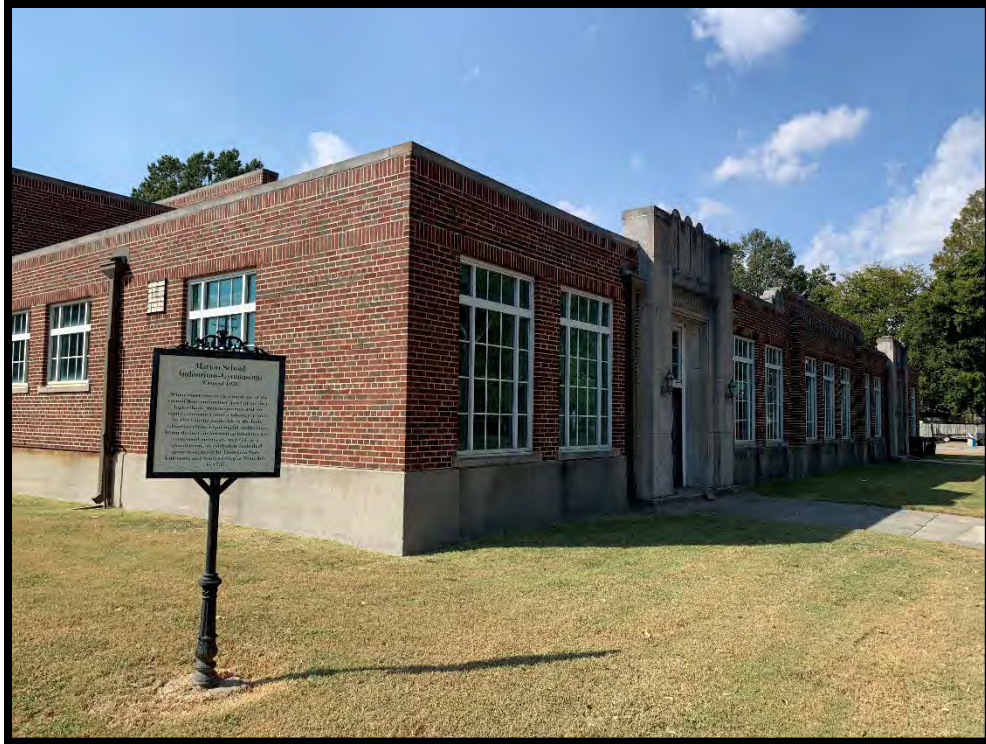
Photograph 3: View north of east side of building on subject property.
