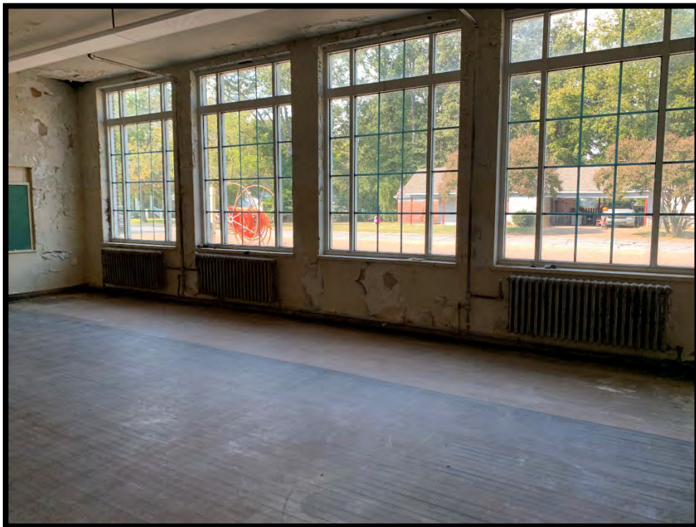
Photograph 12: View of classroom on southern portion of building.
