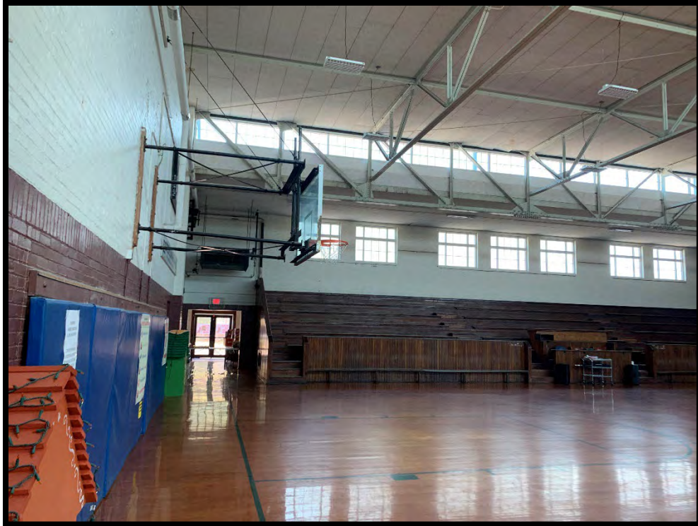
Photograph 9: View east of gym area inside building on subject property.
