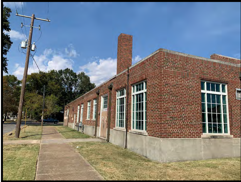
Photograph 25: View of transformers on western boundary of subject property.
