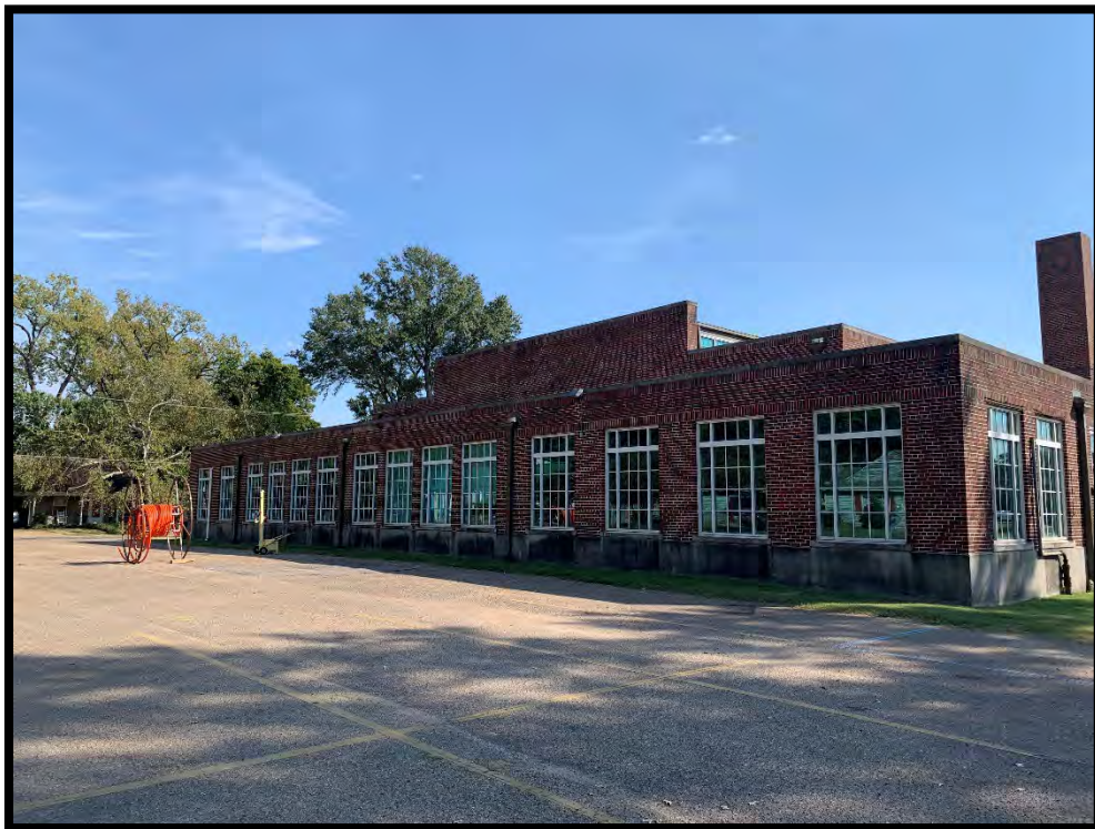
Photograph 4: View southeast across parking lot on the southern side of the subject property.
