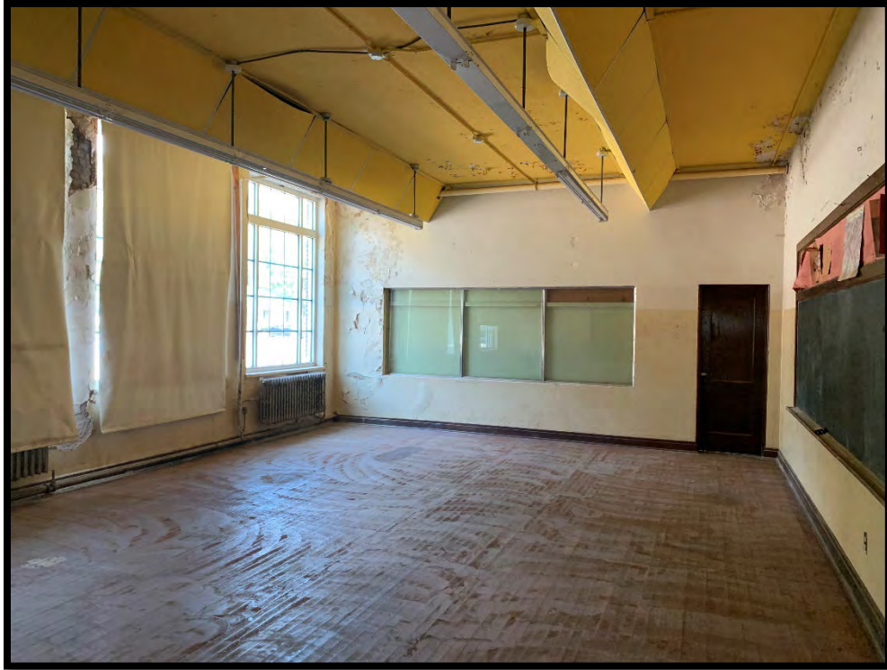
Photograph 11: View of classroom on southern portion of building.
