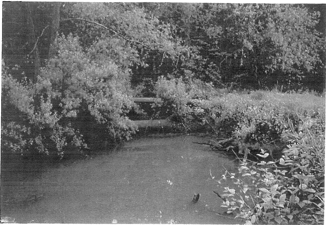
Figure C-25. GLCC-Central Outfall 001 with no discharge. Note brine line downstream of discharge.
