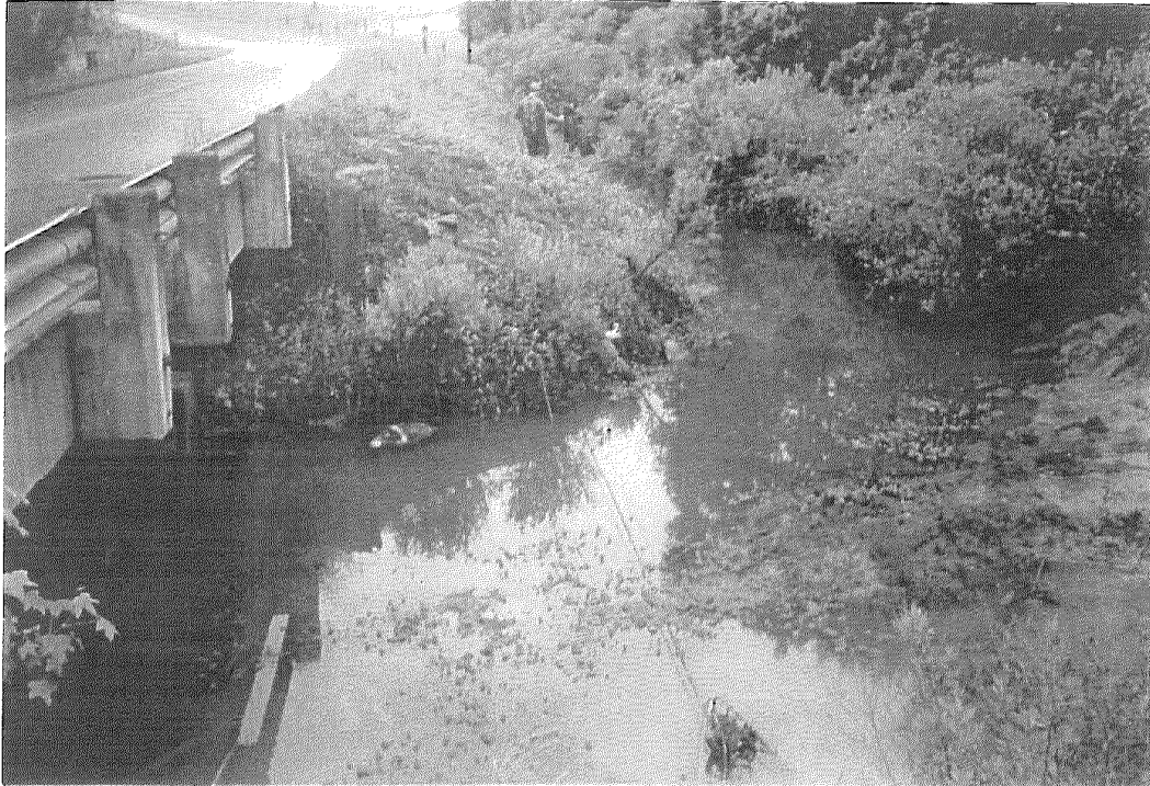
Figure C-1. BDL-1 upstream of County Road during Spring 1999.
