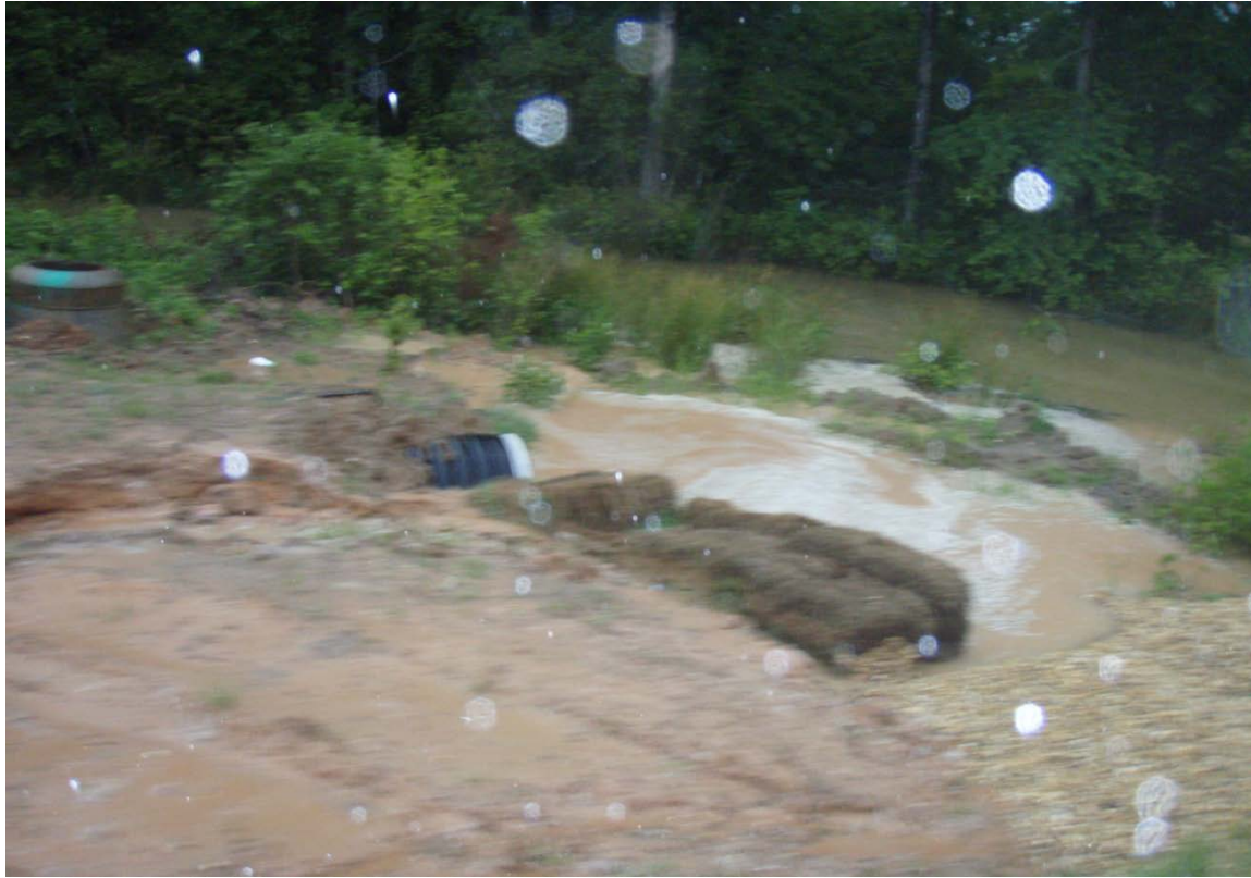
Figure 5.20. Storm water runoff into Loutre Creek upstream of study reach LC-1. Storm flow from construction site for new high school. Loutre Creek in background. July 2009.
