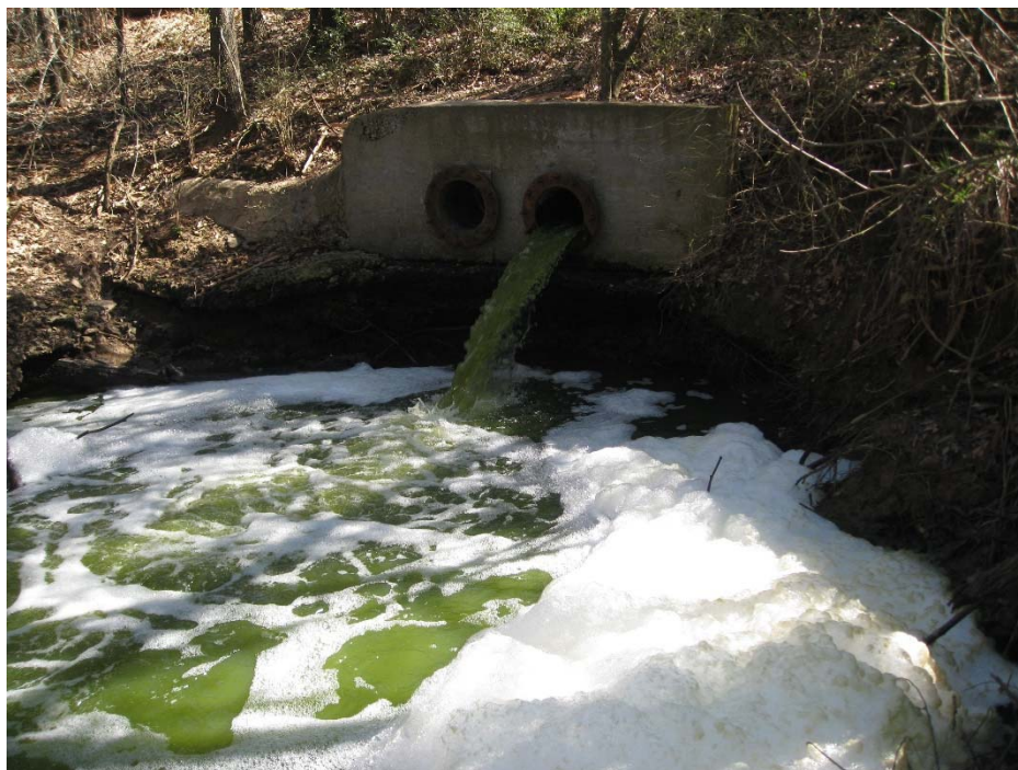
Figure 6.6. Discharge from the City of Waldron's Equalization Basin.
