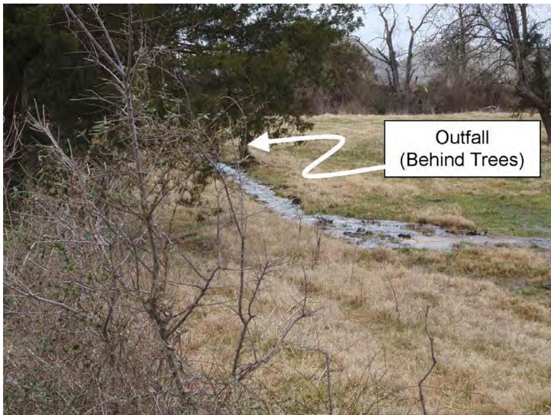
Figure 1.3. Outfall 001, located behind trees.
