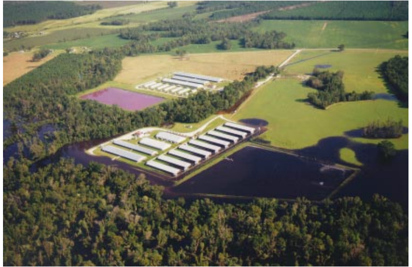
Brown's 5 & 6, a wholly-owned Smithfield hog factory, lost the contents of one of its cesspools to floodwaters caused by Hurricane Floyd. This factory is located along the Trent River above New Bern, North Carolina.
