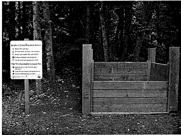
Figure 37. Use of Composting Facilities
