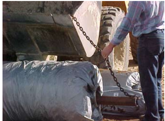
Figure 10E-5 Unloading a roll with steel pipe through core
