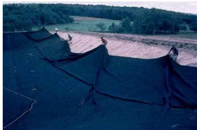
Figure 10E-1 Geotextile padding
