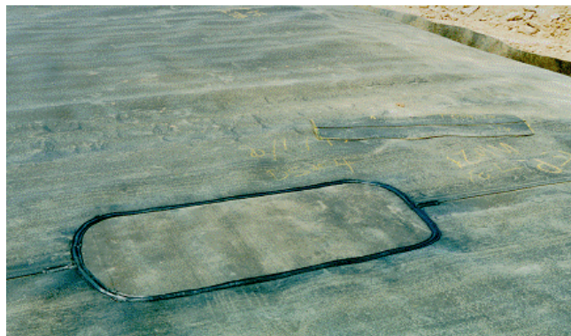
Figure 10E-30 Liner repair
