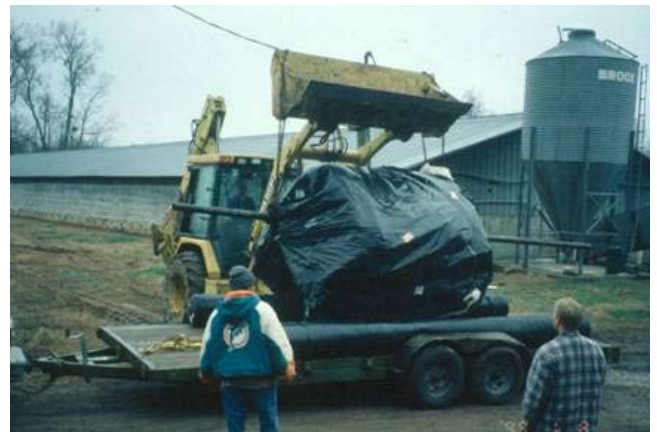
Figure 10E-5 Unloading a roll with steel pipe through core
