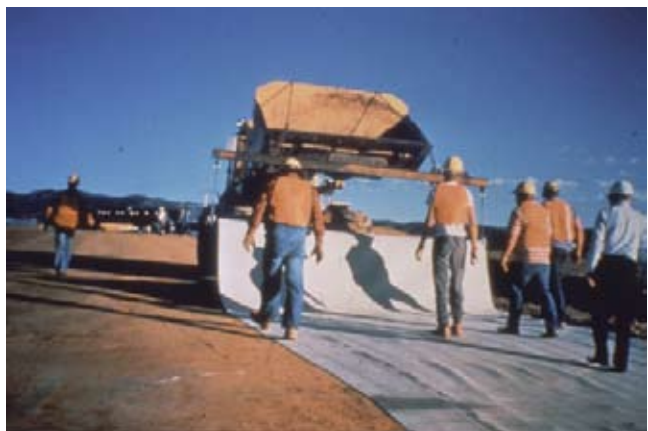
Figure 10E-8 Moving roll pull
