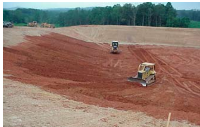
Figure 10D–11 Bathtub construction of clay liner ( photo courtesy of NRCS Virginia (top) and NRCS Nebraska (bottom) )
