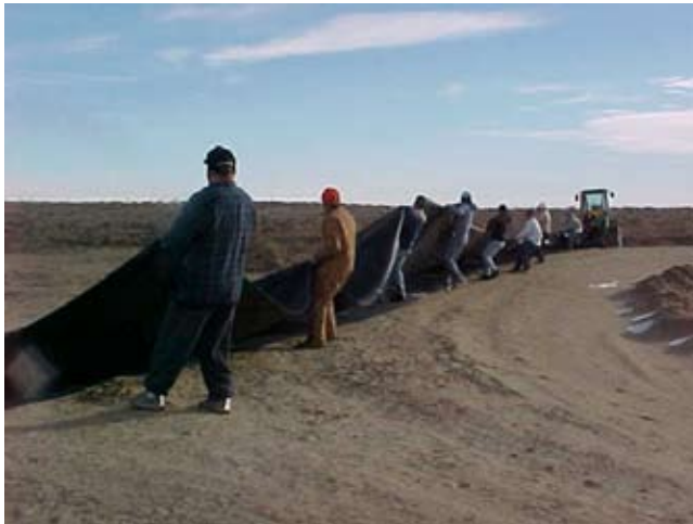
Figure 10E-10 Floating liner into place
