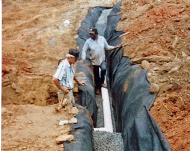
Figure 10D-28 Perforated collector pipe installed the gravel envelope with trench lined with geotextile
