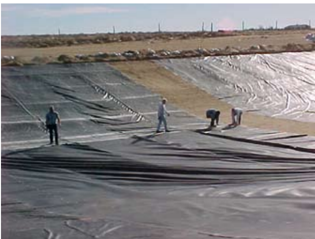
Figure 10E-6 Seams up and down the slope
