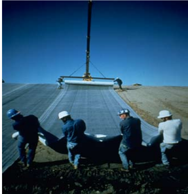
Figure 10E-7 Stationary pull
