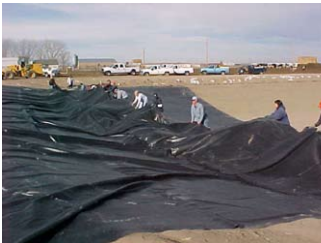
Figure 10E-10 Floating liner into place
