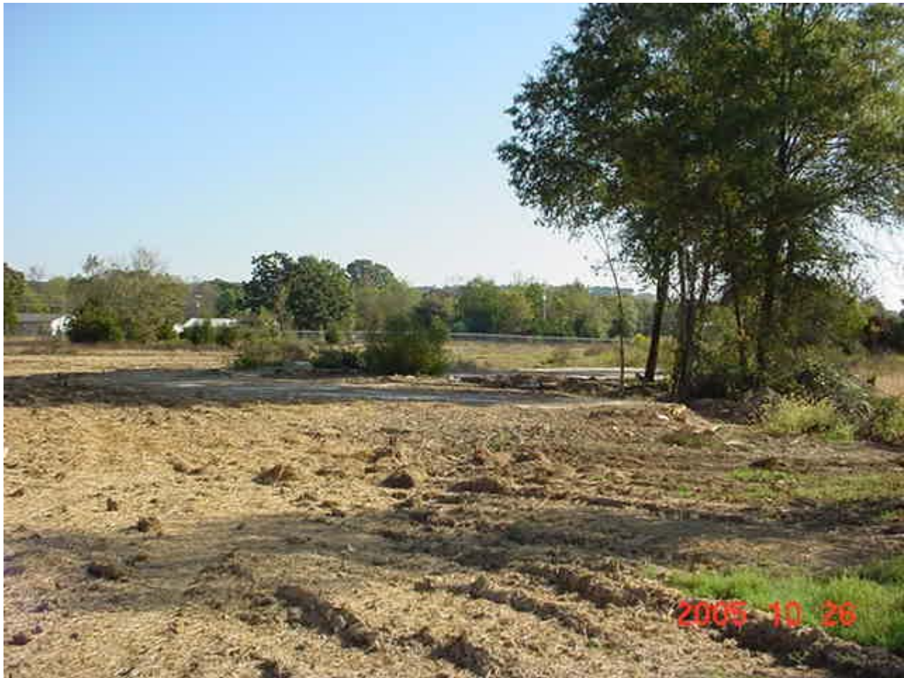
Mountain Pine Pressure Treating Site (Photograph taken post-remediation on October 26, 2005)
