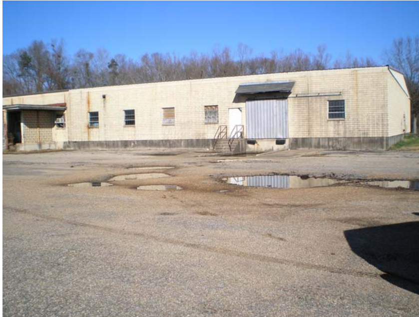
Photo: Front of Building of Former Value Line Company on Third Street.
