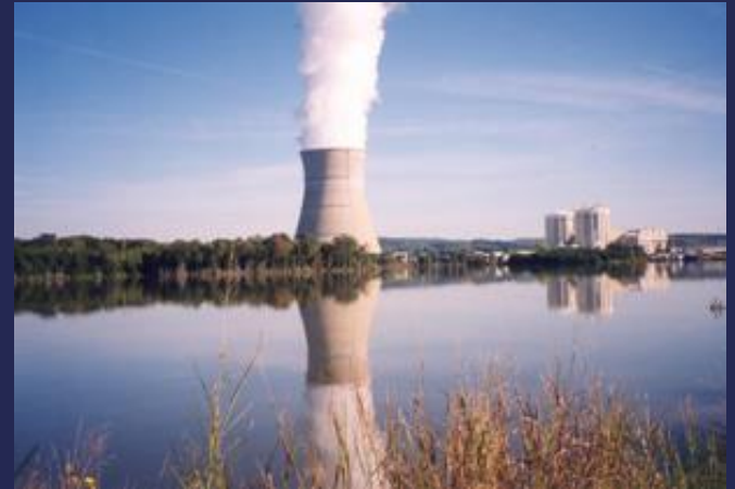
Industrial Water Supply
