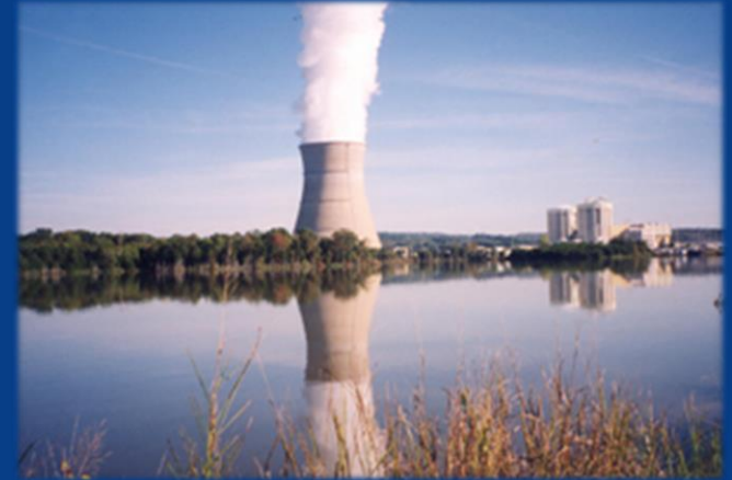
Industrial Water Supply
